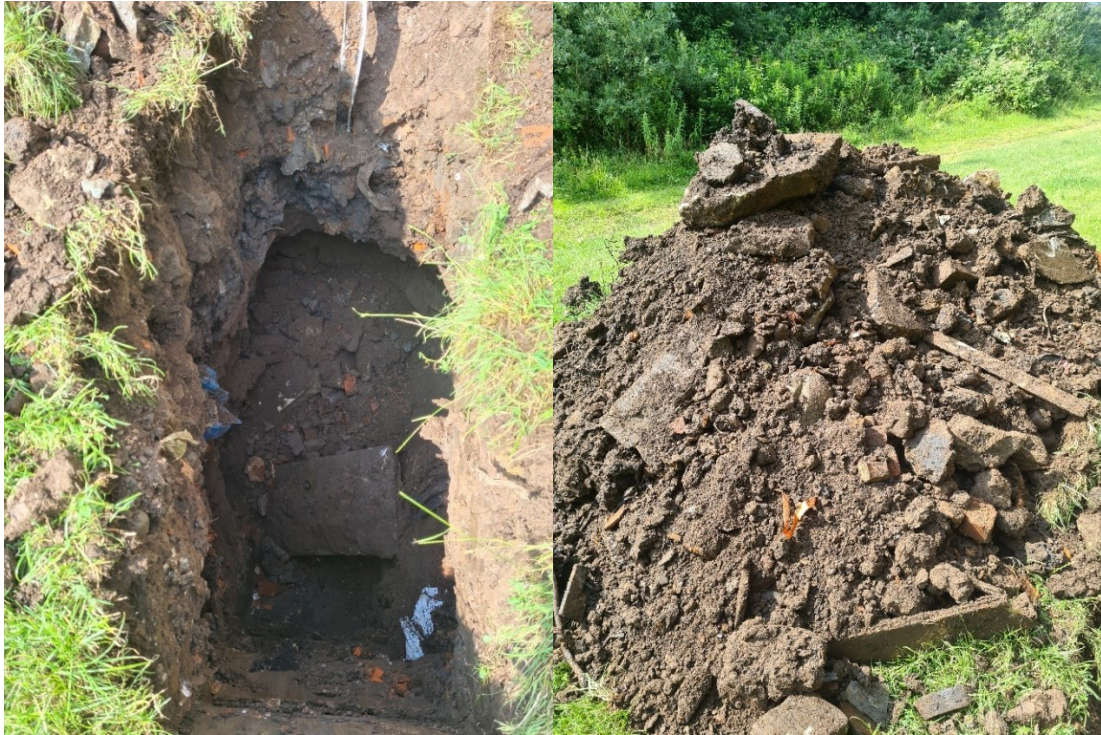
PLATE 7 TP103 EXCAVATION AND ARISING
