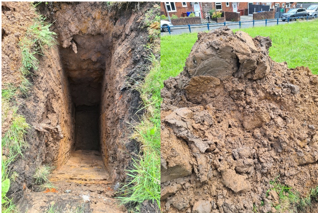
PLATE 8 TP107 EXCAVATION AND ARISING
