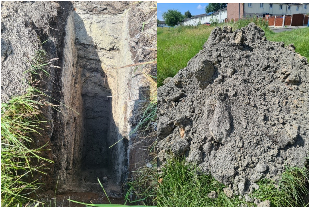
PLATE 6 TP101 EXCAVATION AND ARISING
