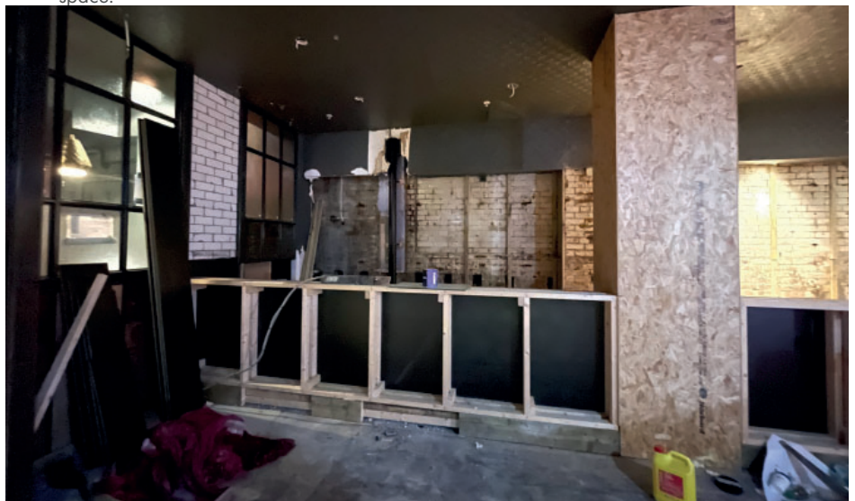
6 View of the reception area where evidence of timber studwork remains on the tiled brickwork.
