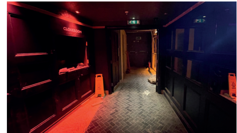
12 View along the corridor showcasing the extension of the timber paneling and the studwork to the end of the corridor.
