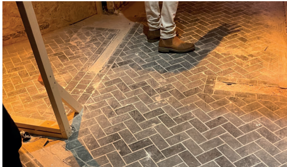
2 View of the modern tiled finishes. Evidence can be seen of where previous walls sub-divided the space.
