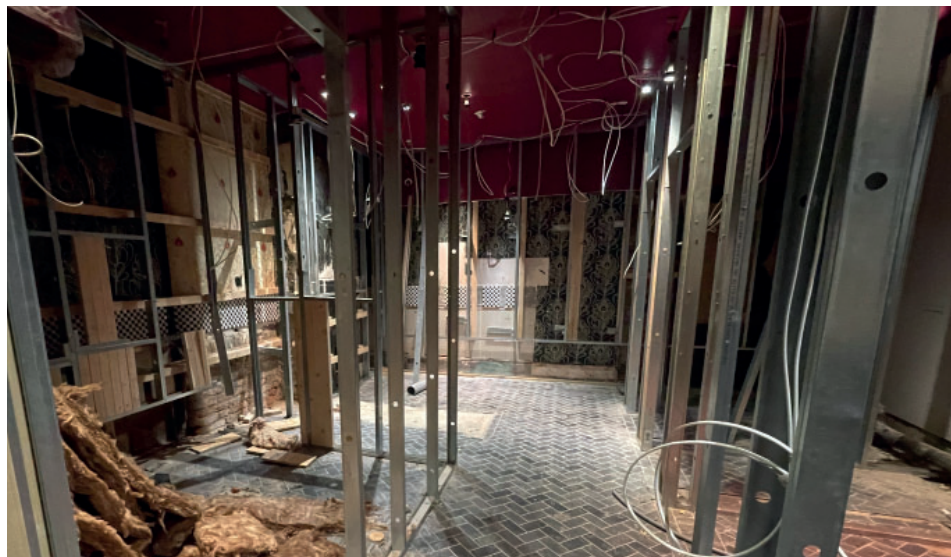
4 View of the existing male changing rooms. The existing stud walls remain unfinished, as does the tiled floor.
