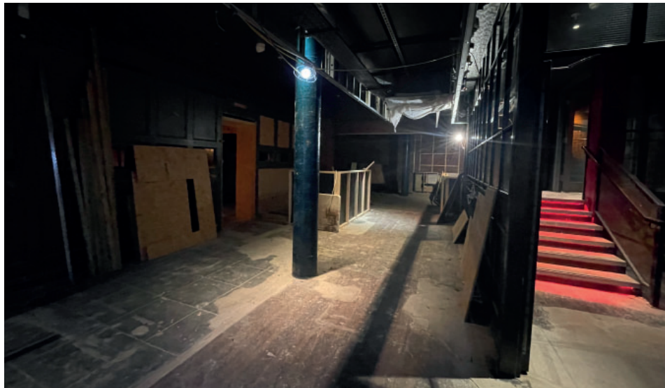
3 View of the entrance towards the yoga studio. Timber panelling can be seen throughout this space.
