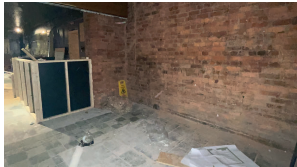
10 View of low level timber stud walls within the reception space.
