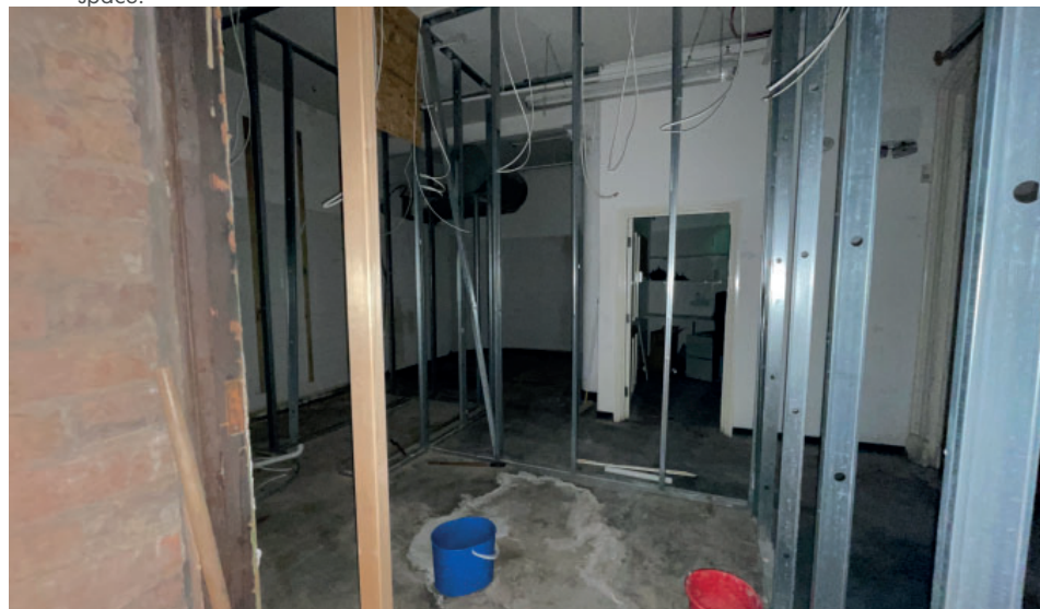
5 View of the existing female changing rooms
