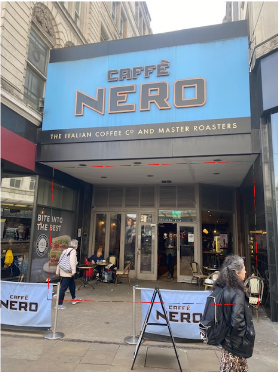
Existing shopfront entrance Red dash line showing approximate position of new shutter
