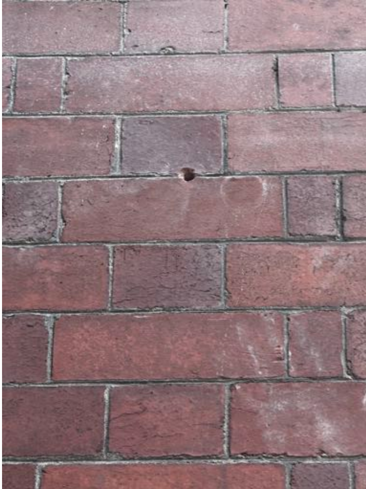
Holes left after scaffolding
