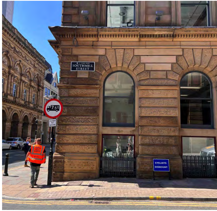
REFERENCE IMAGE SOUTHMILL STREET EXISTING PHOTO
