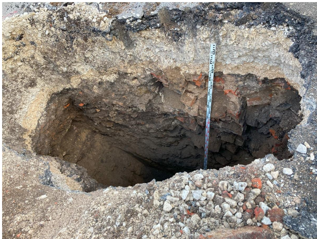
Plate 10 – TP04 gl to 3.1mbgl, with relic in-situ brick wall (0.5m – 2.0m bgl).
