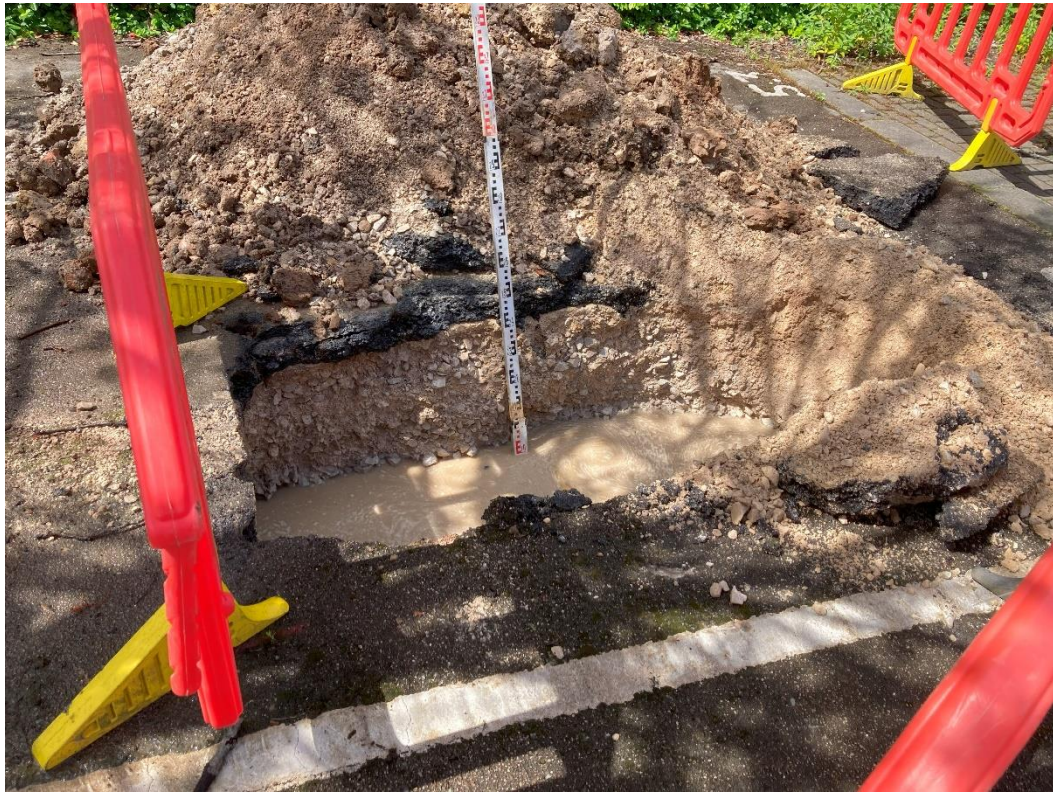
Plate 13 – TP05 undergoing BRE infiltration testing (SA02).
