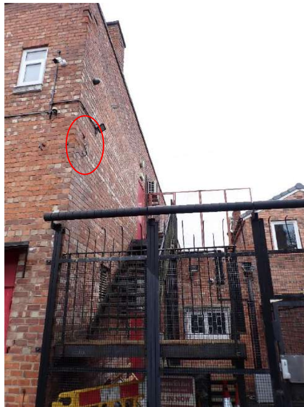
Photograph 4 – north aspect of the building and location of external PRF.
