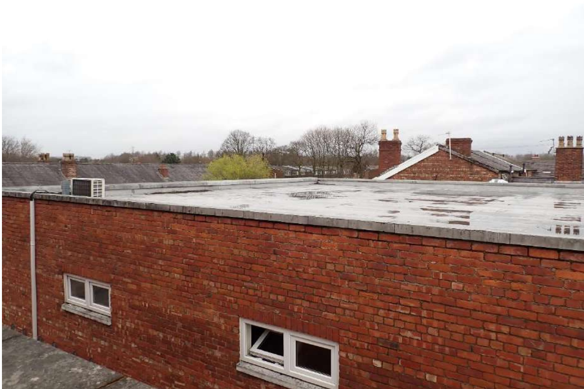
Photograph 6 – view from south to north across roof, showing good condition.
