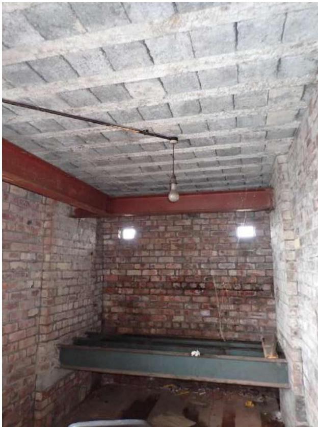
Photograph 11 – view from north to south within the roof access building.
