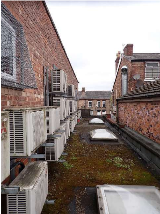
Photograph 7 – flat roof on northern aspect, ajointed to adjacent building
