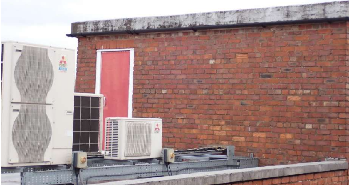
Photograph 5 – view of brick-built roof access building southeast of roof.
