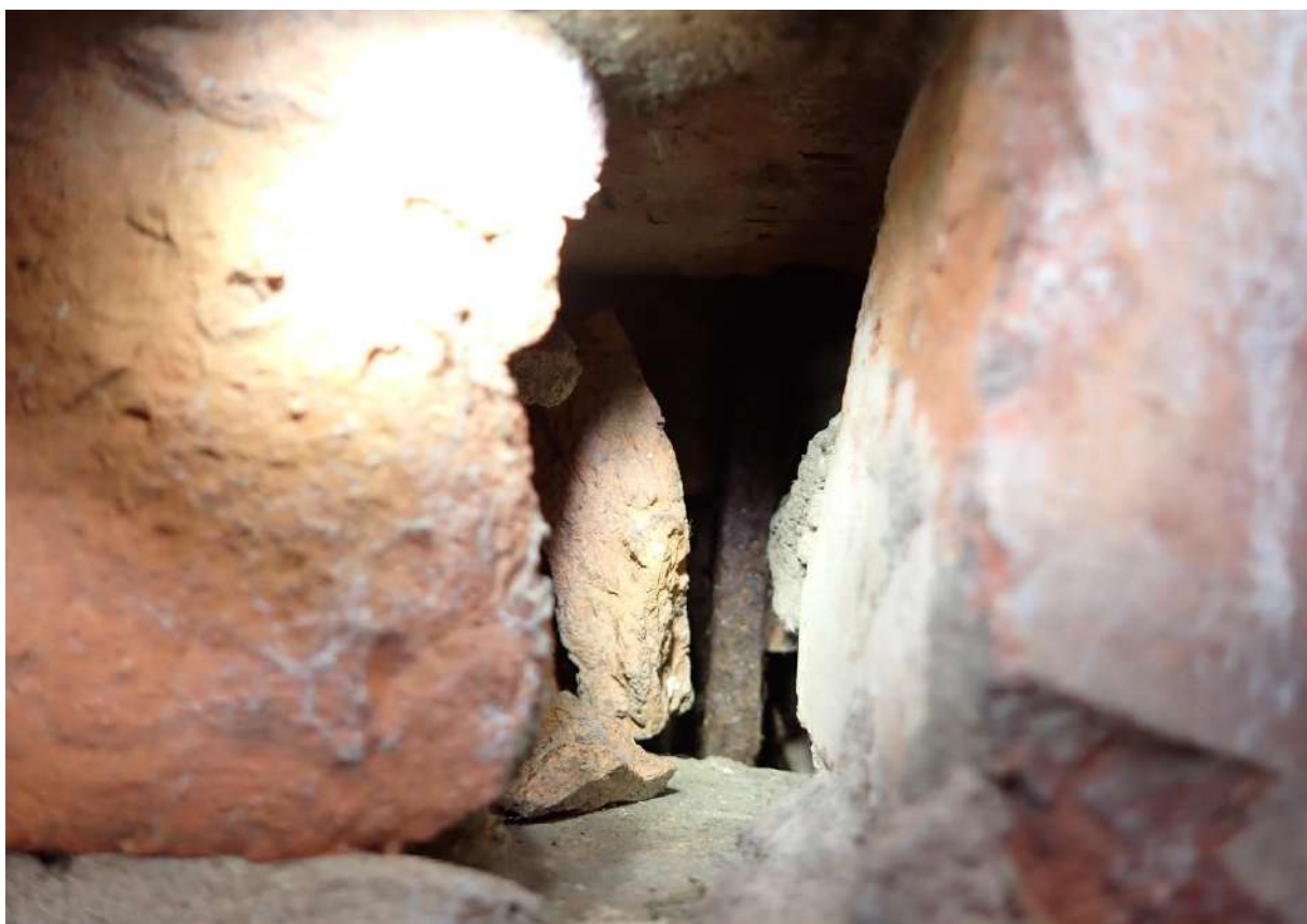
Photograph 9 – close up of wall cavity PRF.
