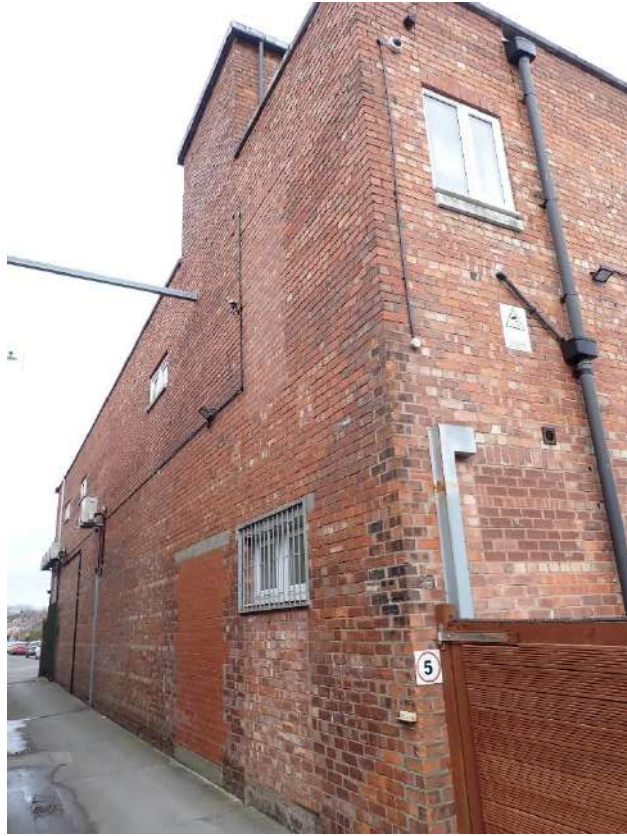
Photograph 3 – south aspect of the building.
