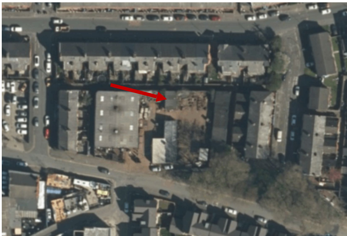
1.6b – Building B3 - Chapel Street – aerial photograph.
