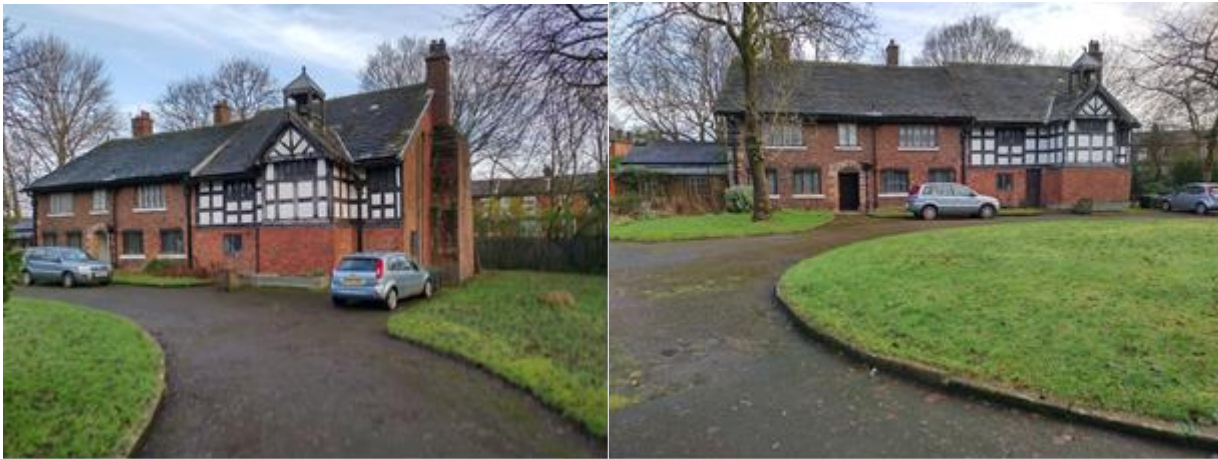
Fig. 2 - Principal elevation Clayton Old Hall (west)
