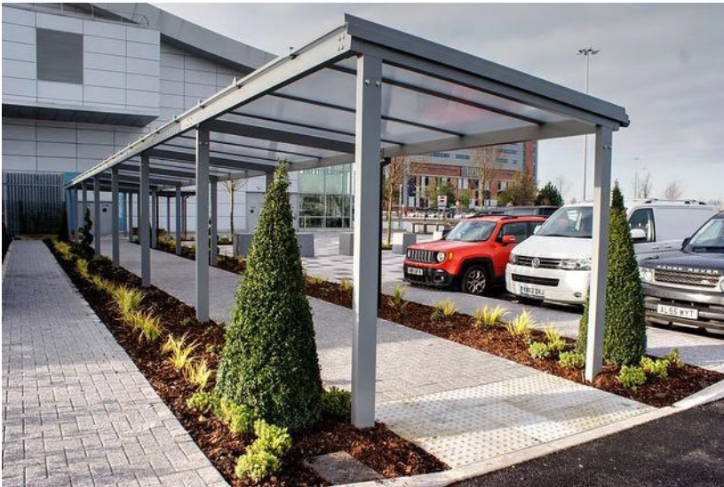
Image 2: Covered cycle parking structure adjacent to the car parking
