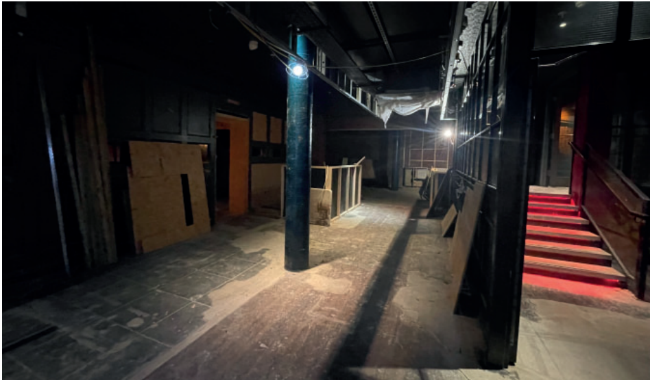
3 View of the entrance towards the yoga studio
