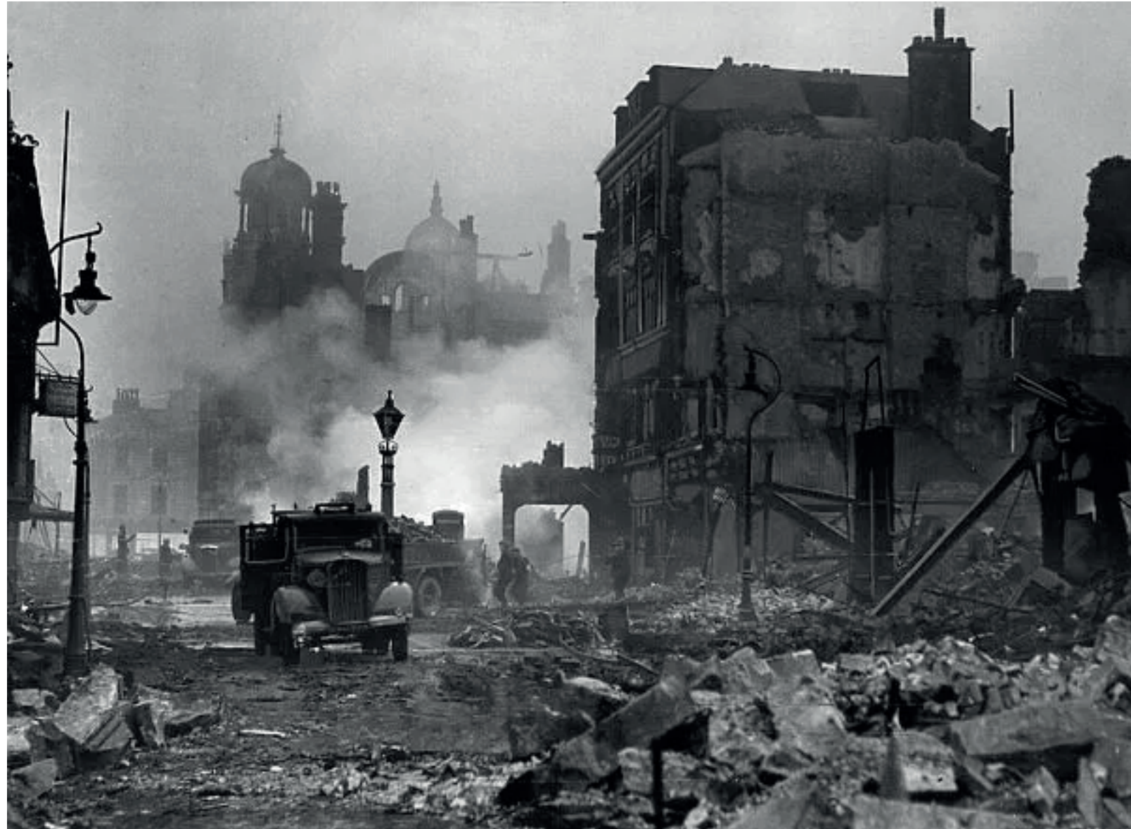
Figure 09 Photo thought to be taken of the north entrance to St Anne's Square, with the exchange in the background. (Source : https://www.mediastorehouse.com/memory-lane-prints/mirror/1400to1499-01466/manchester-blitz-also-known-christmas-blitz-21900435.html accessed 07th July 2023).
