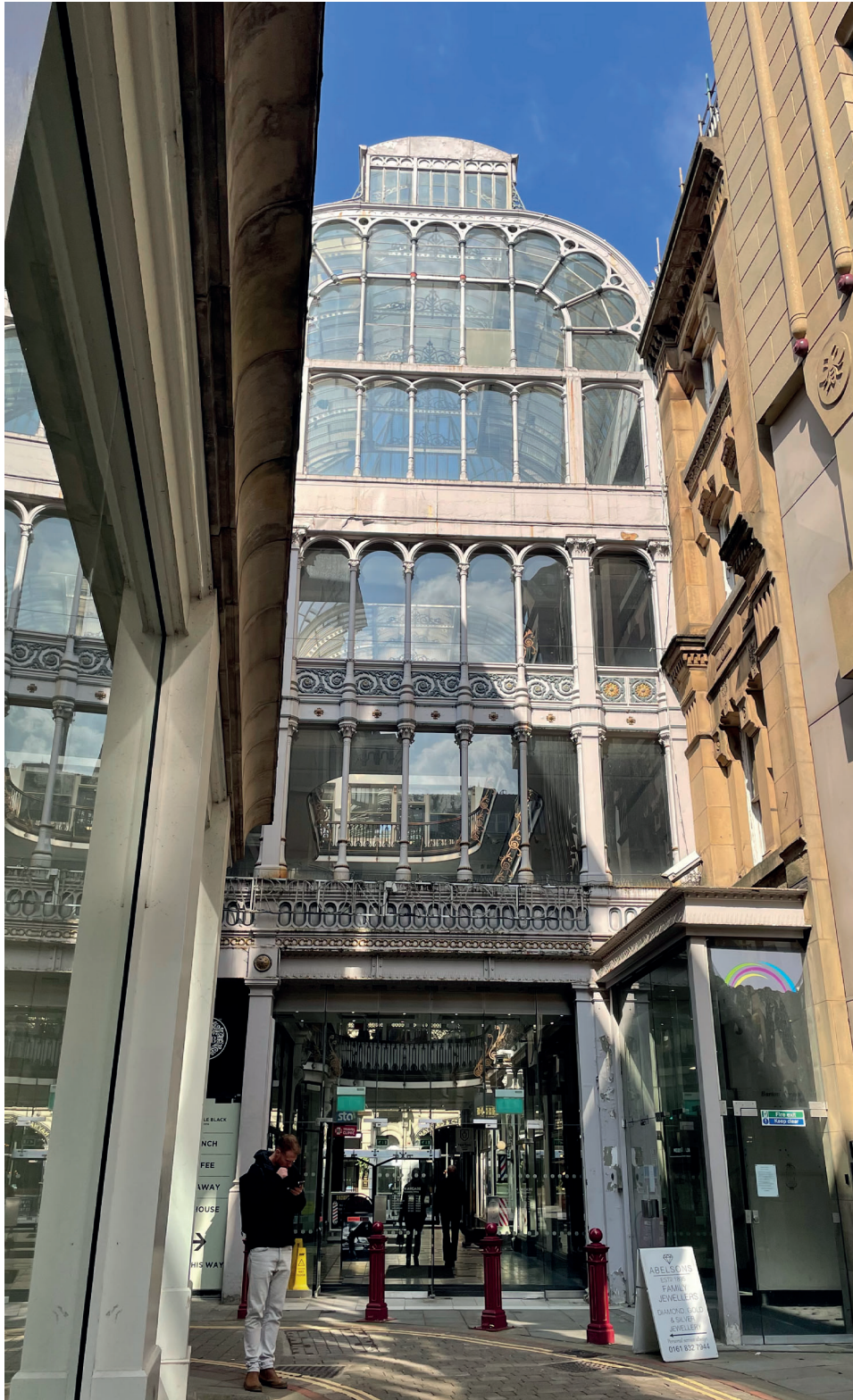
1 View looking to the principle, east, elevation
