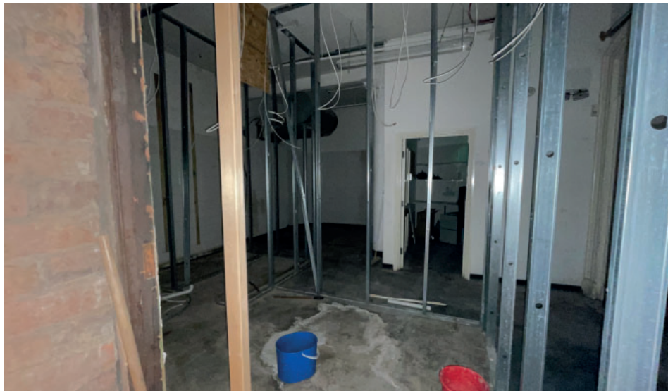
5 View of the existing female changing rooms
