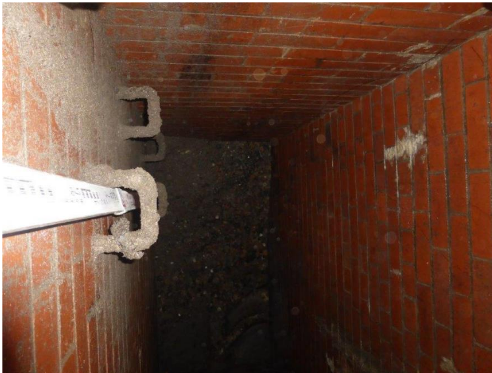
Figure 4-Abandoned chamber found during GI (2)
