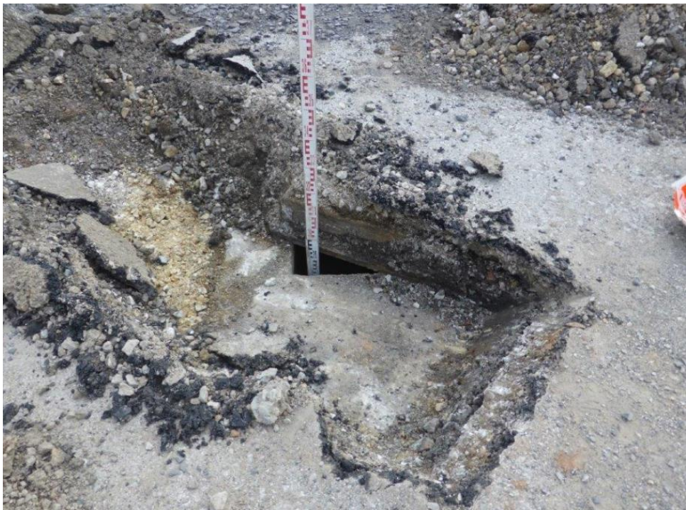
Figure 3-Abandoned chamber found during GI (1)
