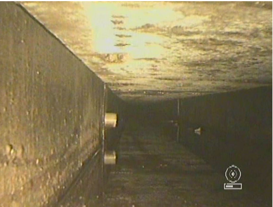
CCTV inspection showing 50mm pipe, suspected to be connected to internal rainwater downpipe which connects into the north cast iron gutter
