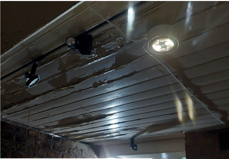
Station Building – Room SB LG05A – Adjacent Arch 6
