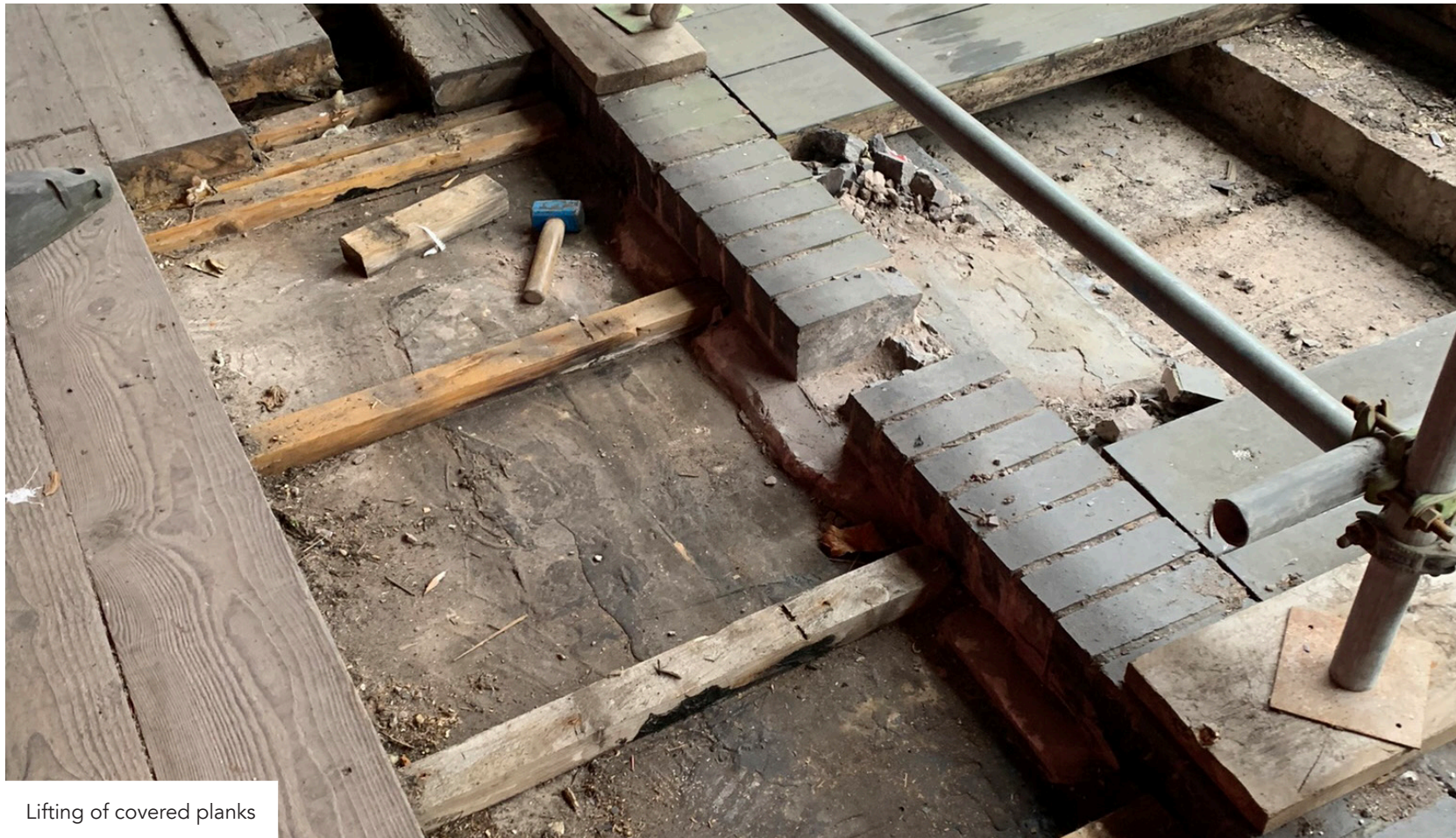
Lifting of covered planks at abutment with glazing
