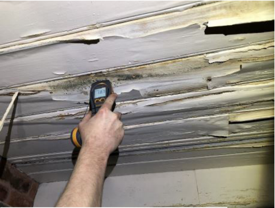
Moisture content reading being taken within the lower ground floor
