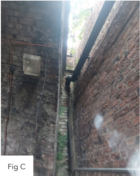
Southern Trough and Station Platform
