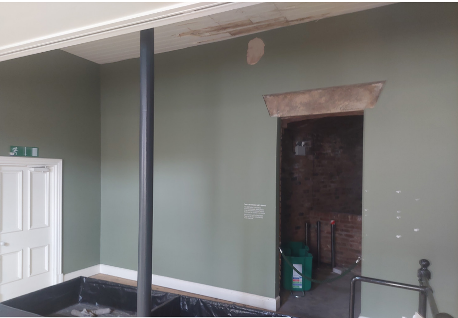
Station Building – Room SB G05 – Adjacent Arch 6
