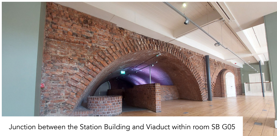
Junction between the Station Building and Viaduct within room SB G05
