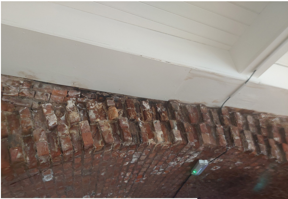
Station Building – Room SB G05 – Adjacent Arches 4-5
