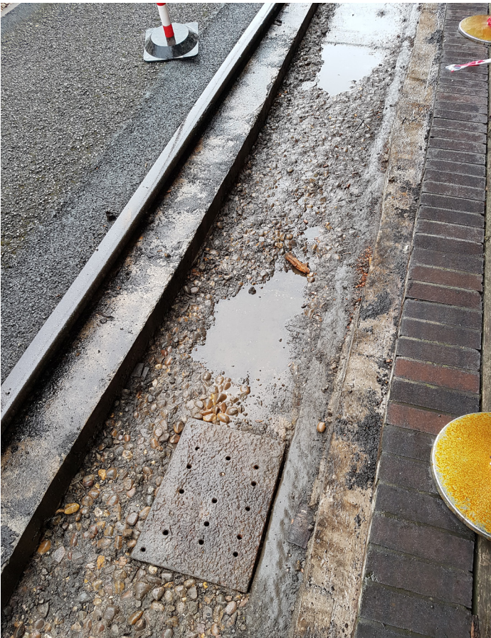
Upper chamber visible following temp removal of timber planks
