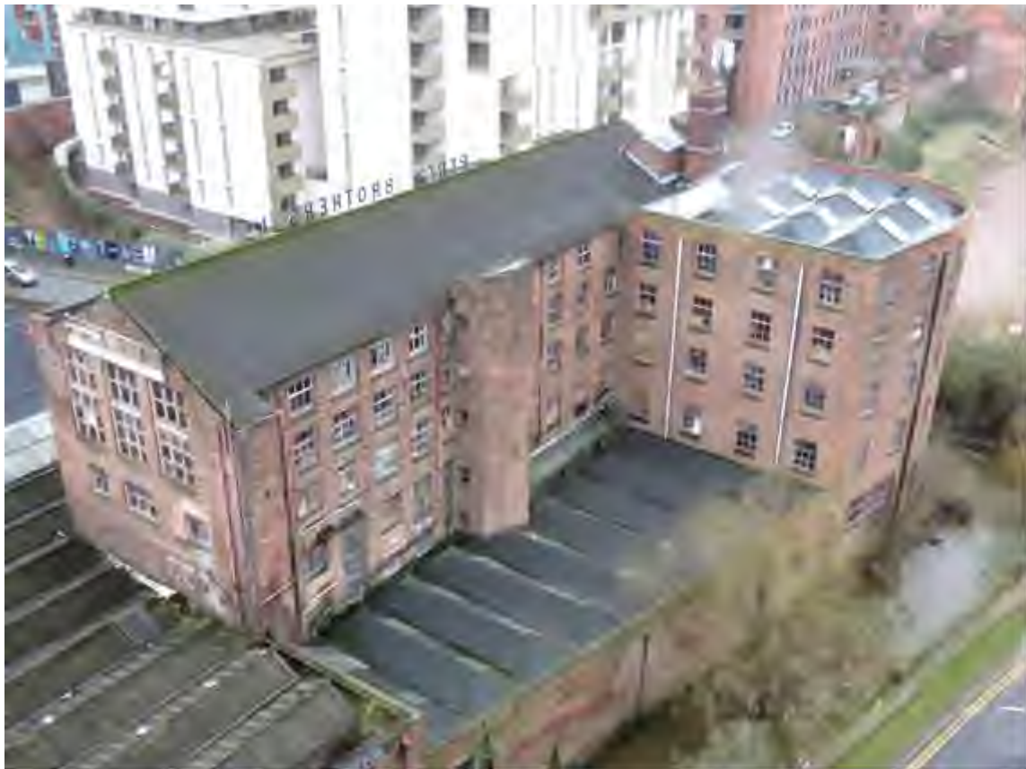
Figure 48: Aerial view from January 2017 view of the north and west elevations of Medlock Mills taken from above the First Street development, surrounded by the north and west single storey sheds.
