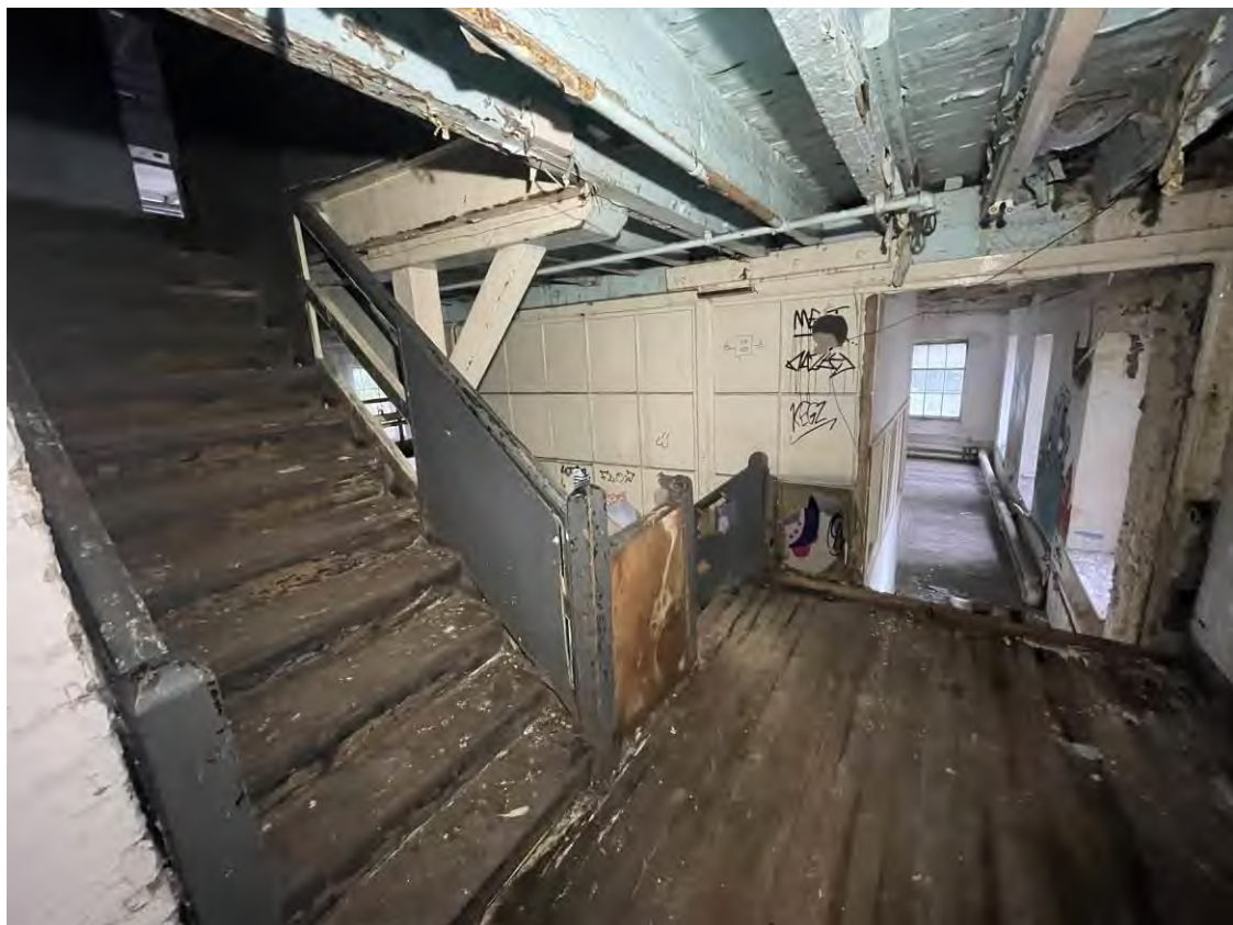
Figure 95: The 1930s staircase, showing the different floor levels.
