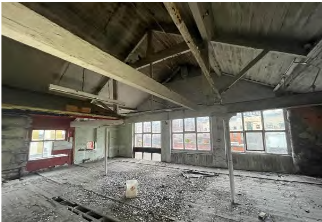
Figure 80: The northern end of the floor, showing the use of a much more slender form of cast iron column, which is likely to be original.
