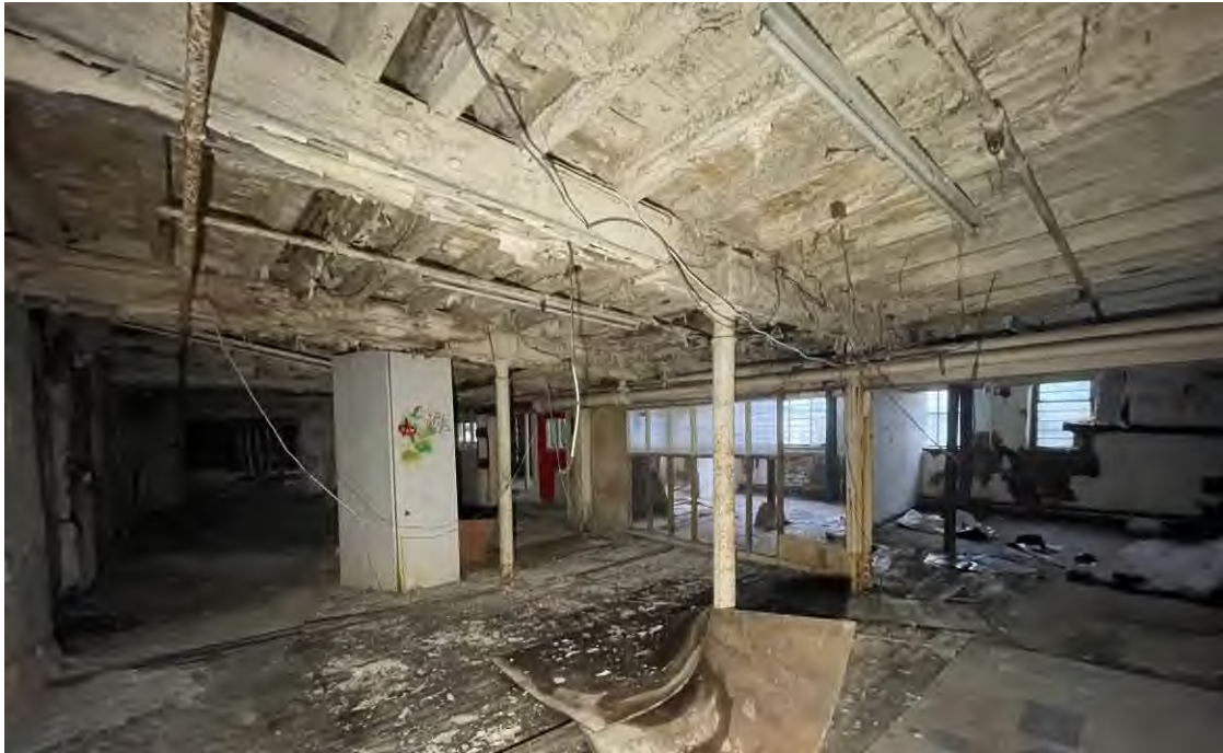
Figure 50: Looking south across the length of the original 1801 mill building, showing original timber ceiling structure supported by cast iron columns.
