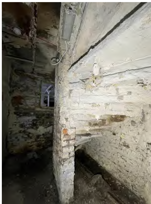
Figure 92: Basement level of the early 1800s staircase
