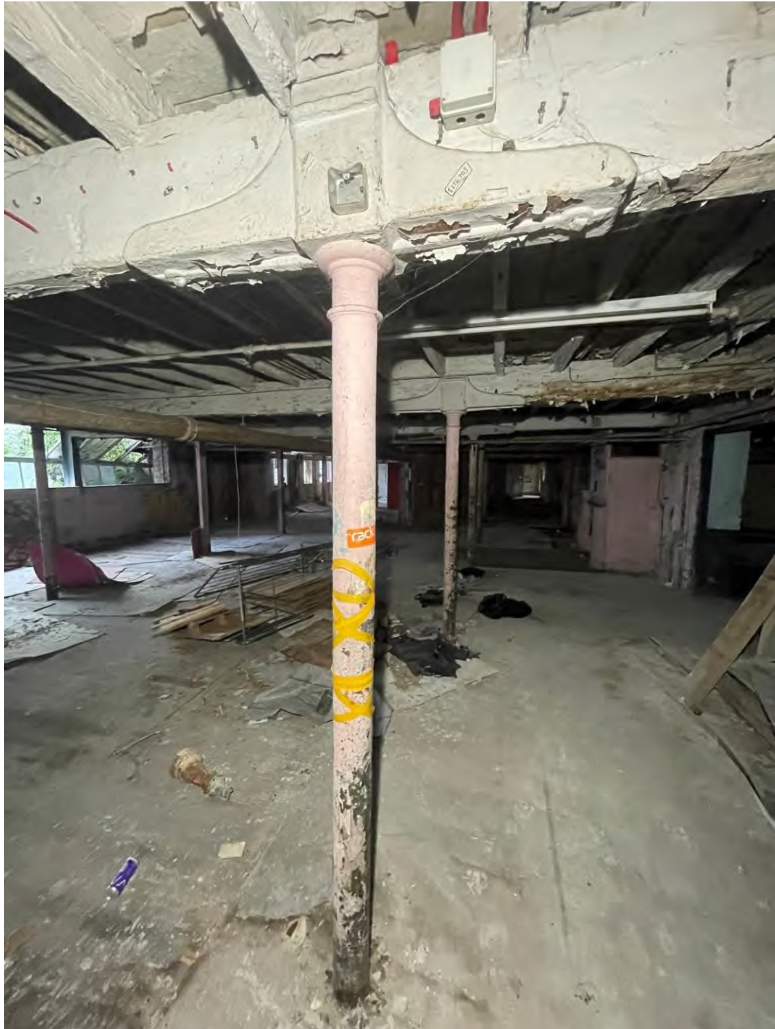
Figure 55: An example of one of the early/original cast iron columns to the centre of the building (looking north).
