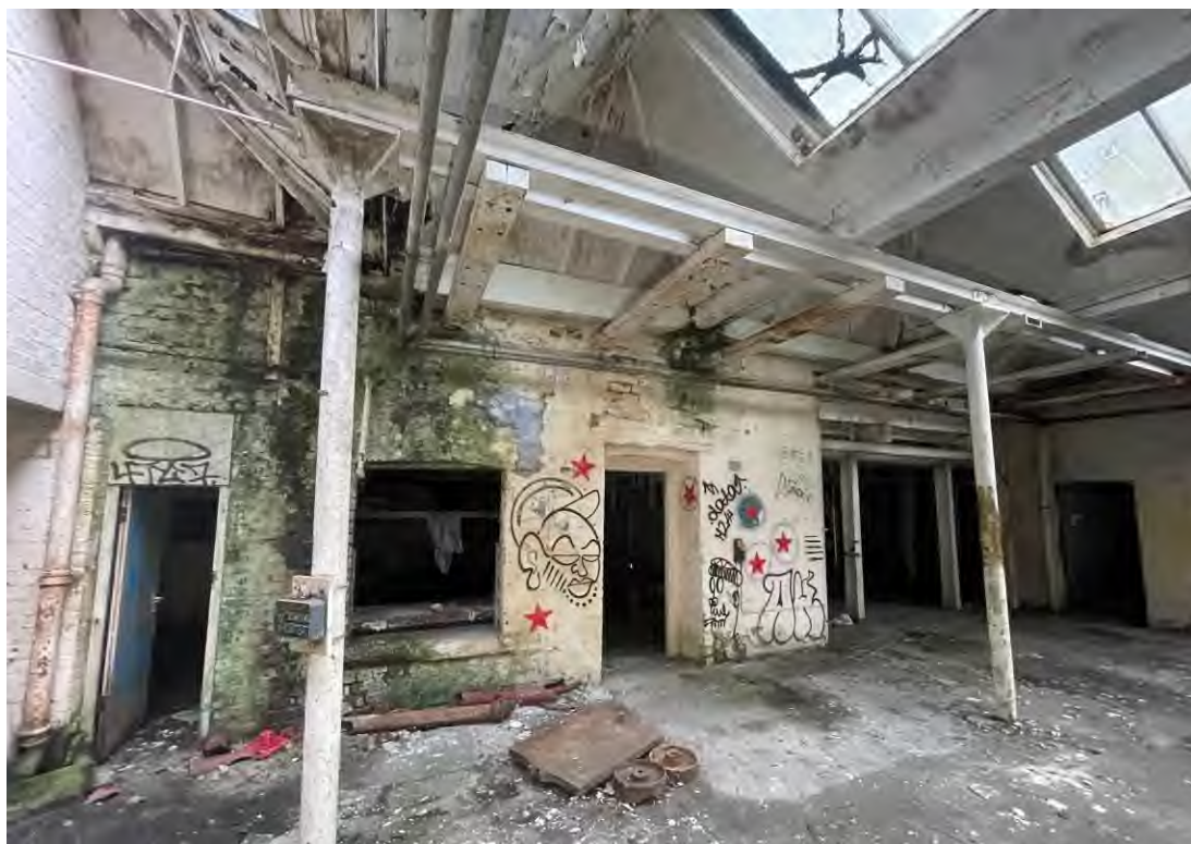
Figure 88: Looking east at the central part of the original lower ground/basement floor level of the 1801 building, which was originally external.
