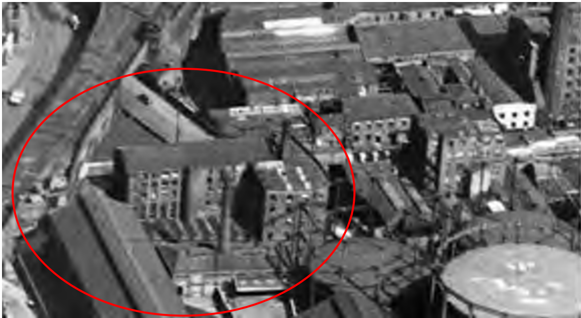
Figure 26 – 1939 – Looking east over the site. (Source: Britain From Above)
