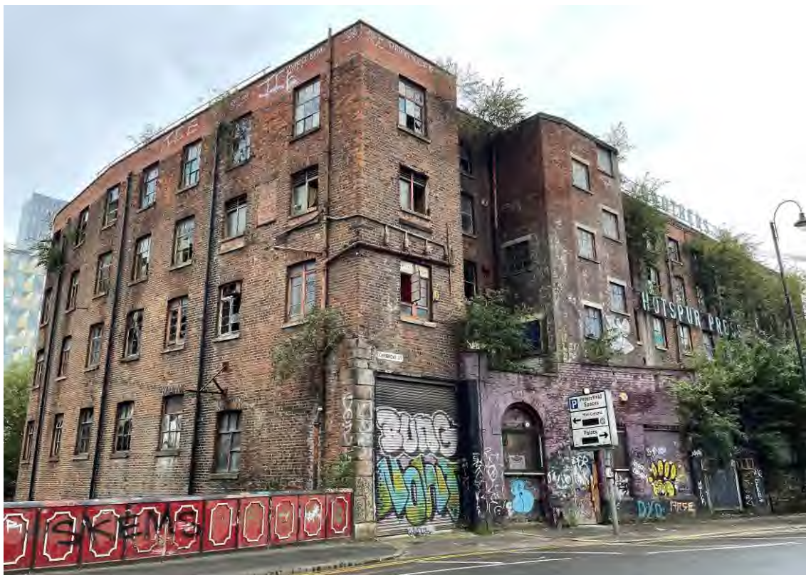
Figure 45: A view looking north-west at Hotspur House, showing the original 1801 mill to the right and later, 1880s curved wing to the left.
