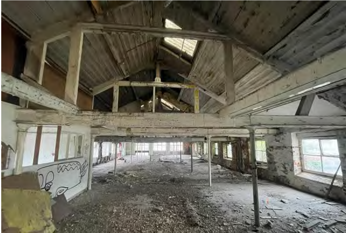
Figure 81: Looking north from the southern end of the 1801 building, showing the slender cast iron columns,
