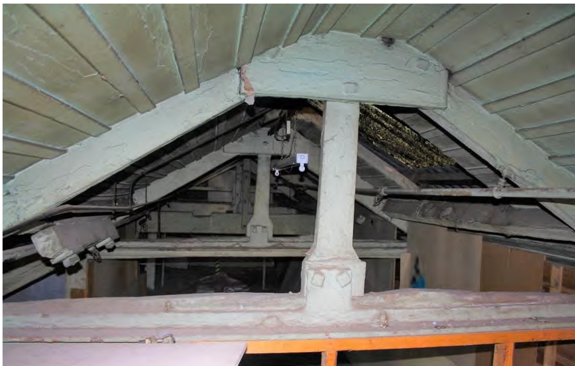
Figure 78a: A view looking through the 1801 roof timbers.
