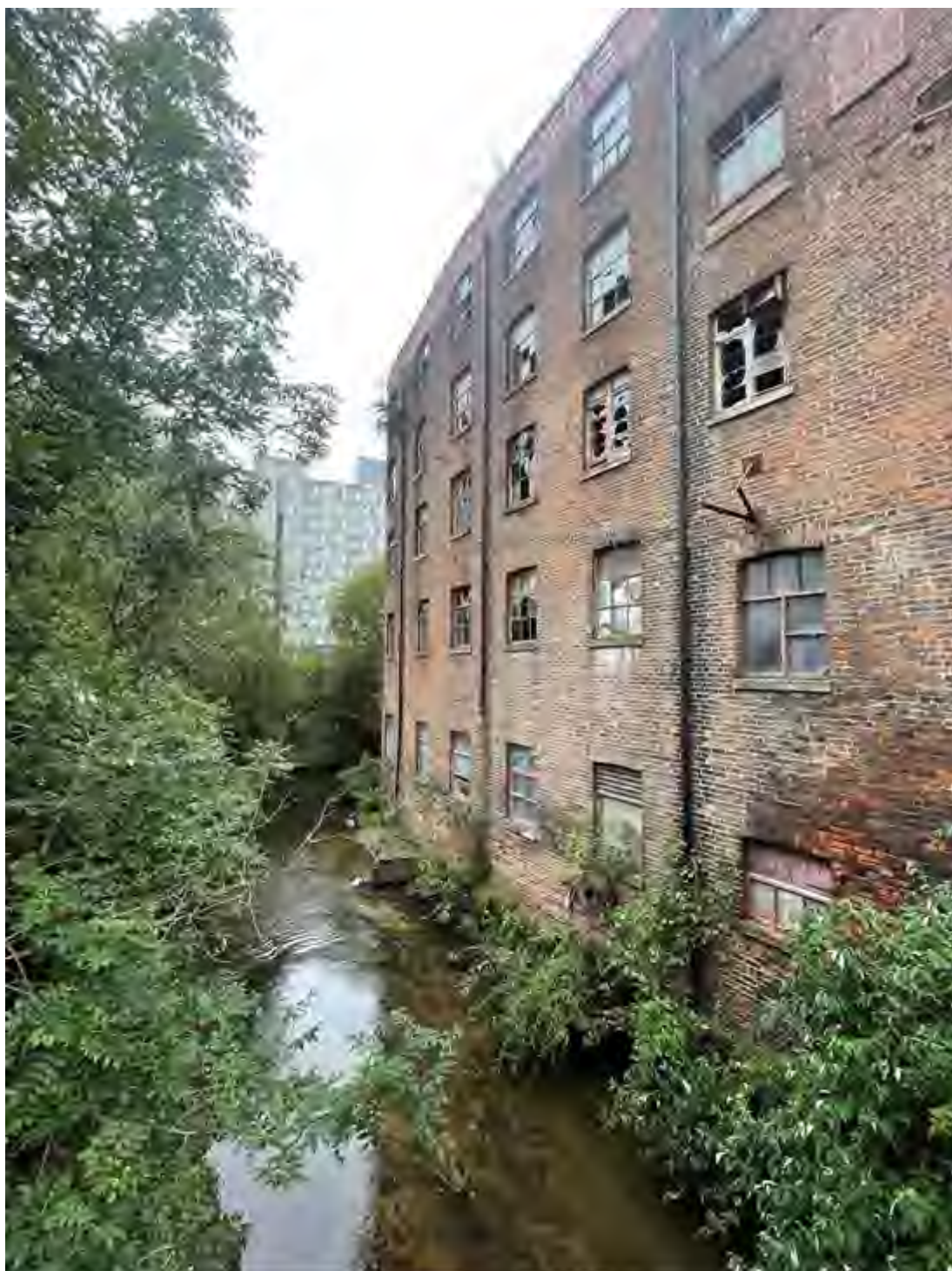
Figure 46: View of the south elevation of Medlock Mills taken from Cambridge Street. Part of the recent First Street development can be seen to the rear of the image.
