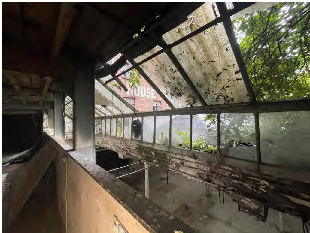
Figure 25: The same structure as seen today.
