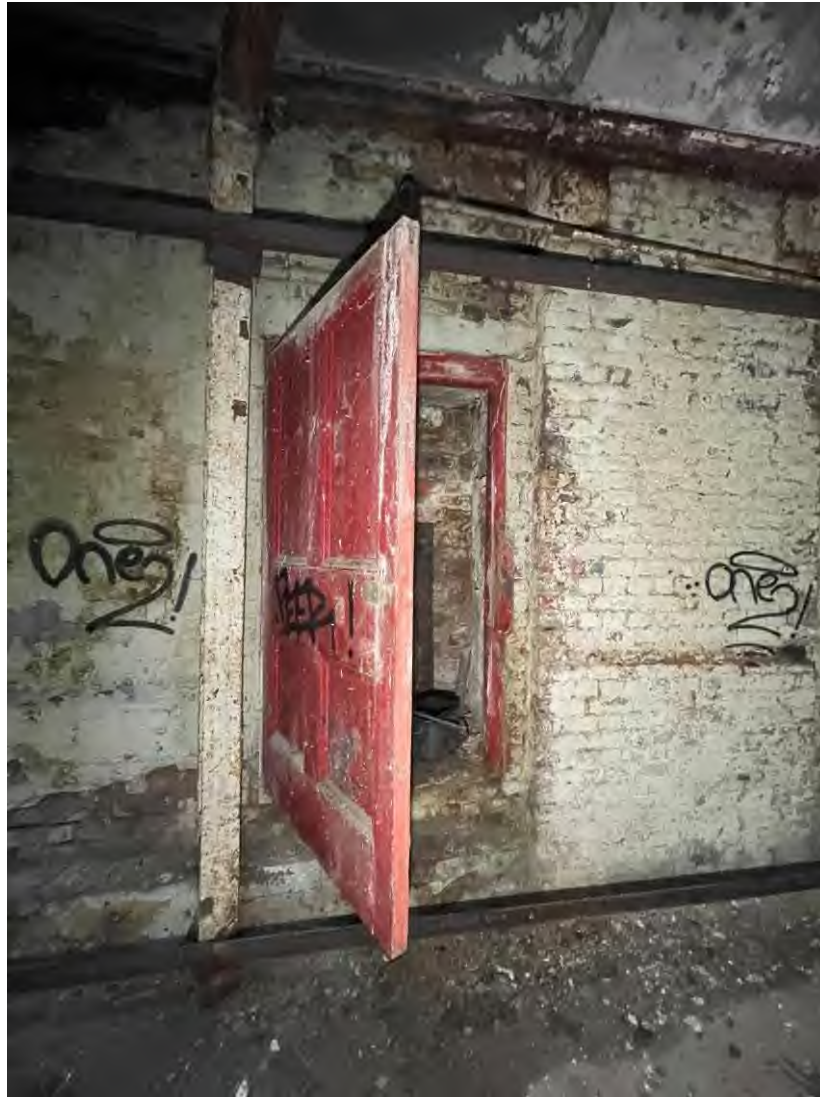
Figure 63: A 19 th century panelled doors within one of the railway arches which will have originally led into Percy Brothers' paper store.
