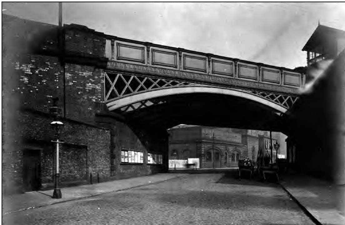
Figure 26 – 1909 – Looking north-east along Gloucester Street. The single-storey shed occupying part of the Site is just visible to the far left of the image. (Source: Manchester Archives)
