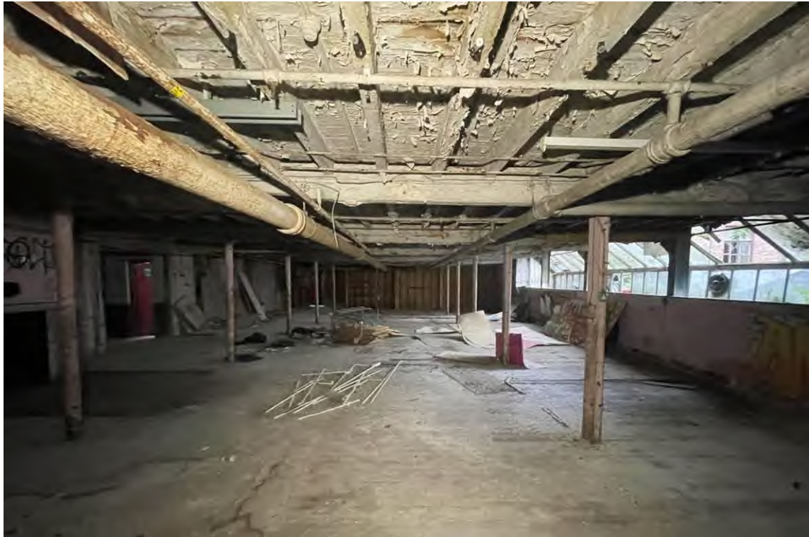
Figure 52: Looking south from the centre of the 1801 mill building, showing the 1907 lightwell alterations to the right, and additional c1950s steel columns.
