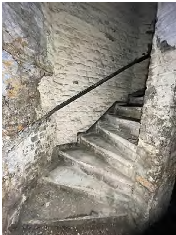
Figure 91: detail of the early 1800s staircase showing stone treads and solid brick external and core walls.
