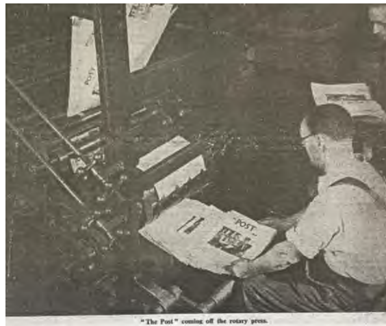
Figure 31 – Collecting printed copies at the delivery end of the machine, ready to be wheeled in a truck to the hoist and lifted up to the Bindery for wire stitching. (Source: Enterprise Rise Demise, Clifford Bevan (2019))
