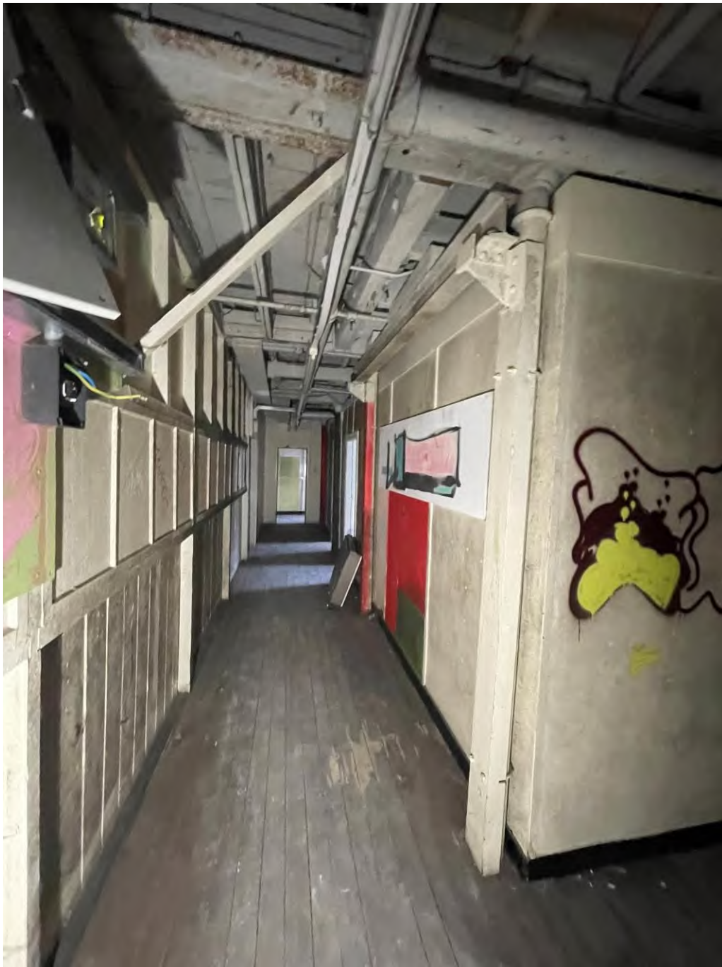
Figure 67: Looking south along the central corridor showing the inserted offices.
