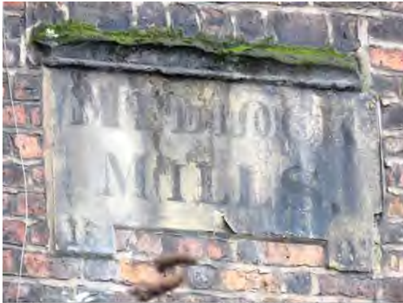
Figure 9: The original date stone stating, 'Medlock Mills, 1801'. This stone can be seen to have been repainted beneath. (Source: SLHA)
