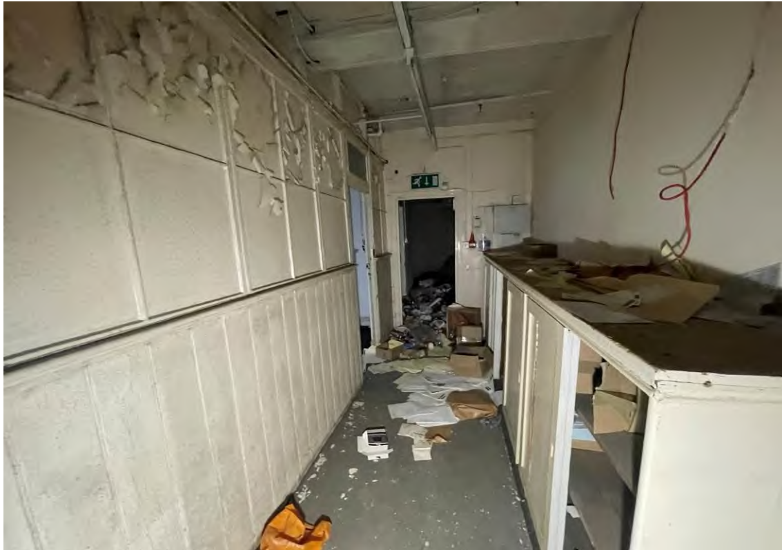
Figure 68: An example of an early 1900s partitioned office.
