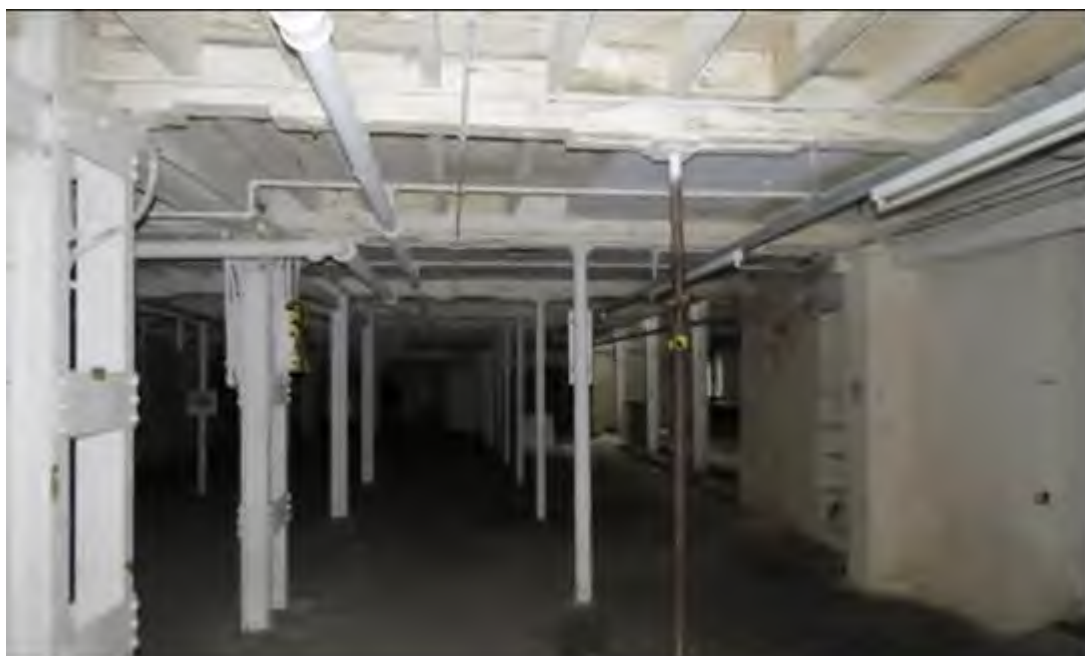
Figure 86: Looking south through the basement level of the 1801 mill, showing some of the original 1801 cast iron columns. Compared to other columns throughout the building, these are very slender with simple mouldings to their heads.
