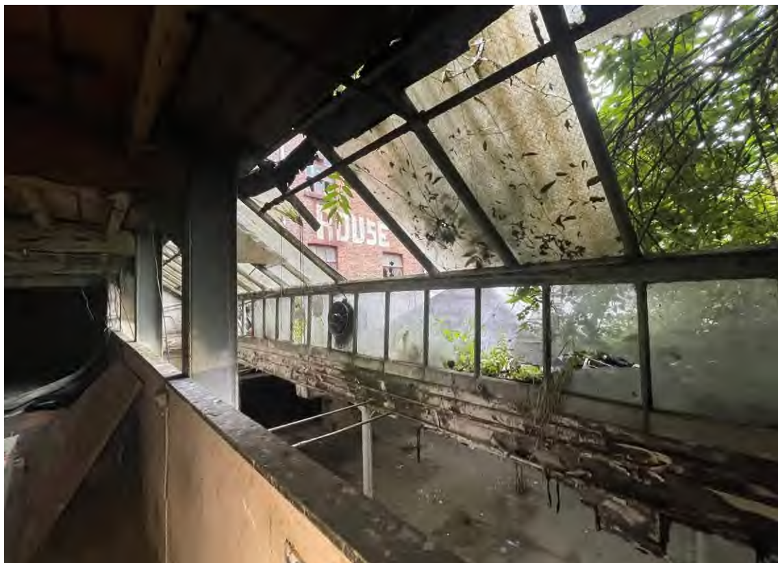
Figure 53: The 1907 alterations, which provided additional light to the ground floor and basement levels.
