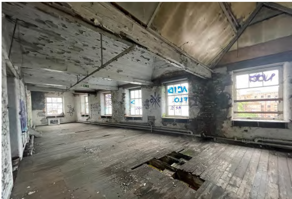
Figure 82: Looking east across the southern, curved 1880s wing, showing the original sawtooth roof.
