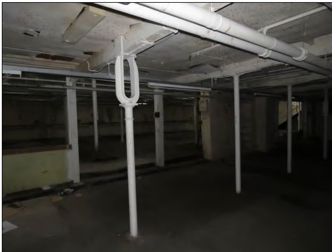
Figure 85: Detail of the interior of the basement level showing a single cast iron column designed with an adaptation to carry moving machinery. Note the slender design of the original c1801 columns at this level.
