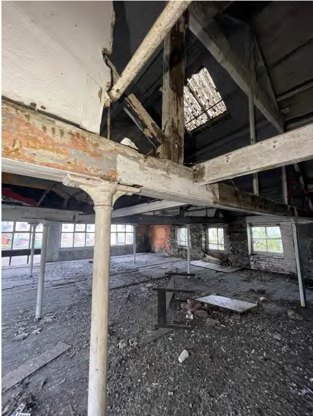
Figure 83: A view of one of the original c1801 cast iron columns, supporting the substantial timber roof structure to the northern end of the floor.
