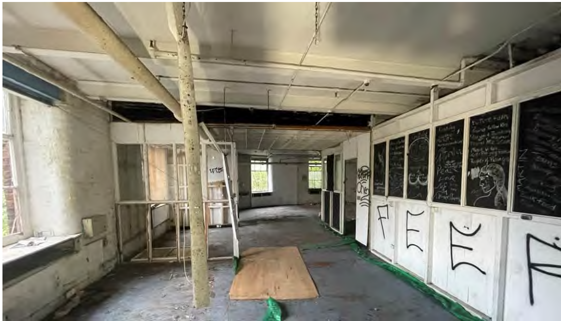
Figure 70: Looking west along the 1880s curved wing.
