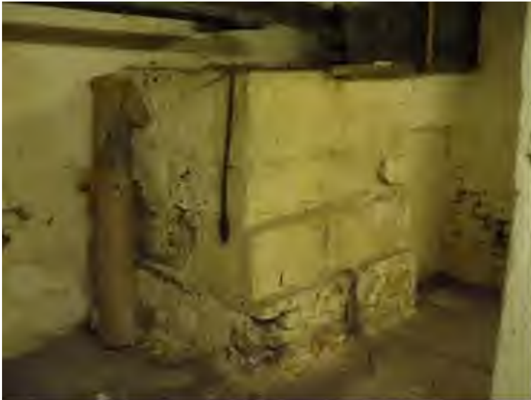
Figure 84: Detail of the interior of the basement level showing large stone block sections at the base of the original steam engine chimney.
