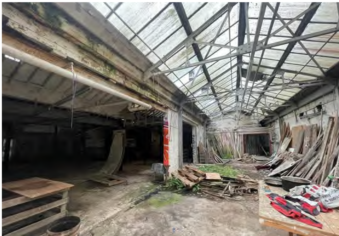
Figure 65: Looking south along the original external east elevation of the 1801 mill (right), and c1860s shed (left). The area to the centre was originally Kenyan Street and now contains a c1950 glazed roof.
