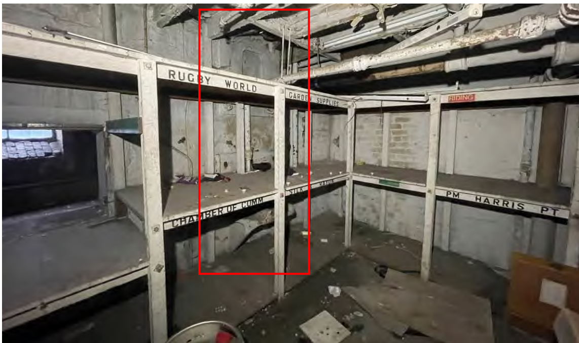
Figure 57: The surviving timber racking showing a number of historic publications adjacent to the entrance office. The hatch (left) led directly to the loading bay and dispatch area. The area outlined red shows parts of the original c1801 cast iron wall openings that originally connected to the mill's steam engine on the opposite side.
