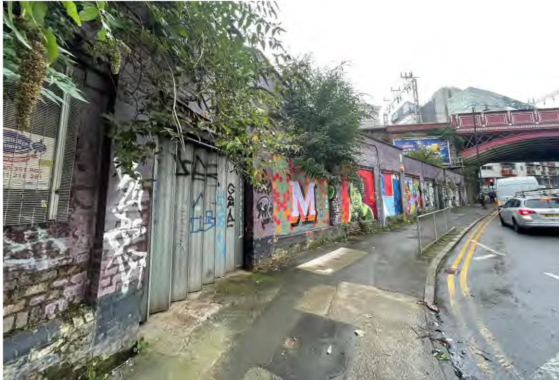
Figure 44: View looking along the c1860s single-storey shed on Cambridge Street.
