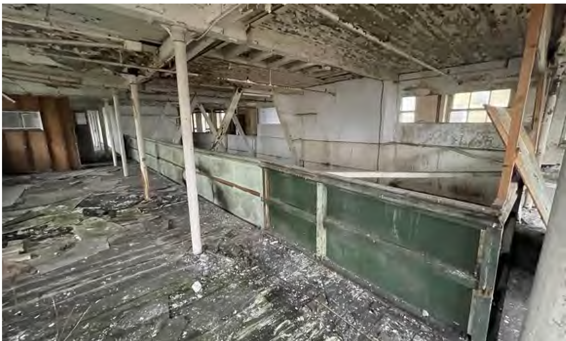
Figure 75: Looking south-west from the northern end of the floor, showing the early-1900s inserted floor opening to the composing room.
