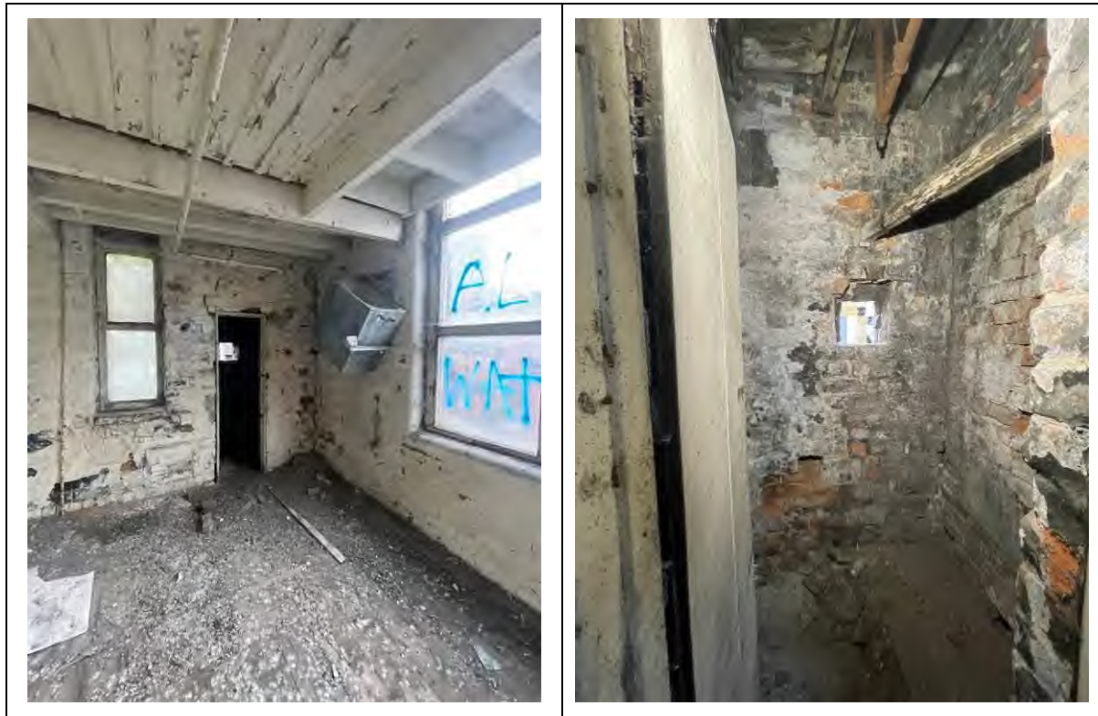
Figure 76 & 77: An unusual example of a surviving 1801 mill worker's latrine. Originally each floor level had a single latrine for workers, all housed in a narrow, projecting tower structure to the north-west corner of the 1801 mill. This example retains its original, wide timber plank door, roof structure and early paint finishes.
