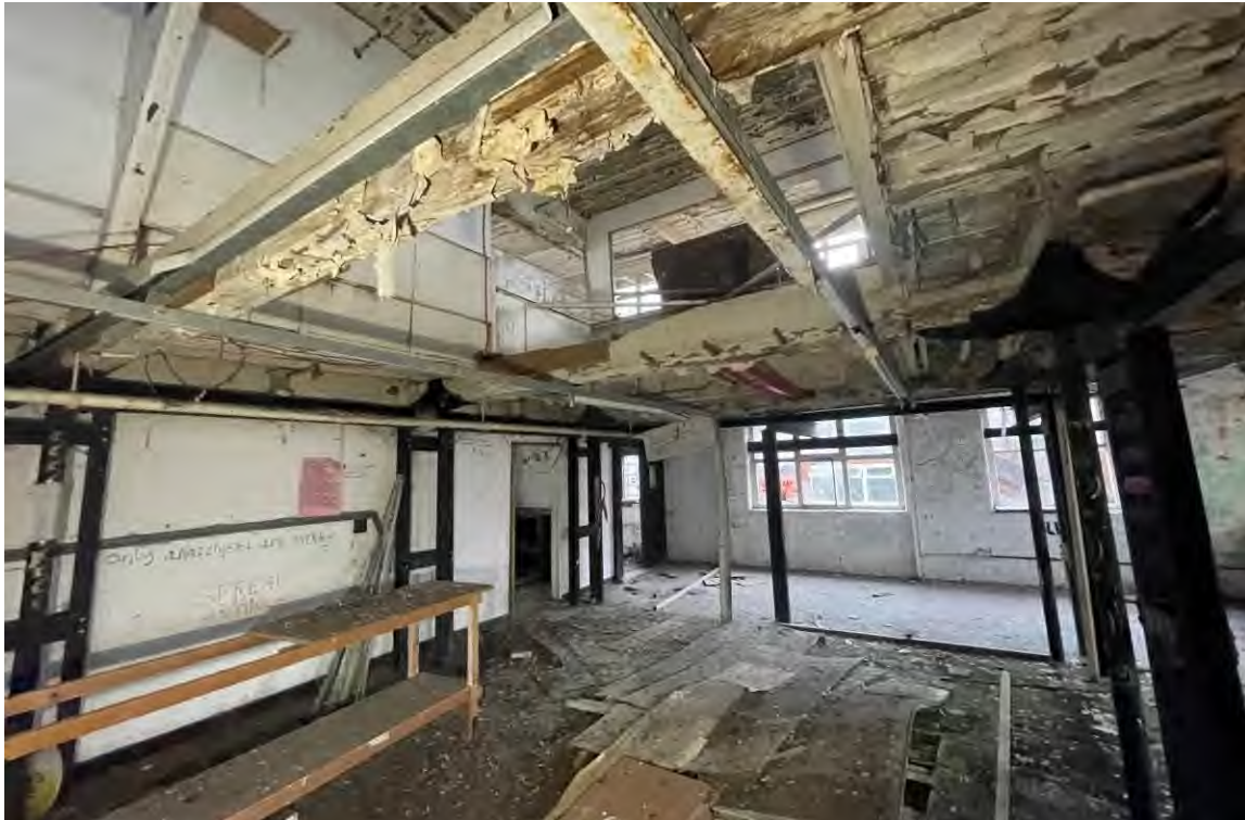
Figure 72: Looking north at the northern end of the floor, showing the large, early-1900s inserted gable windows and opening in ceiling allowing for printing machinery to be placed and illuminated.
