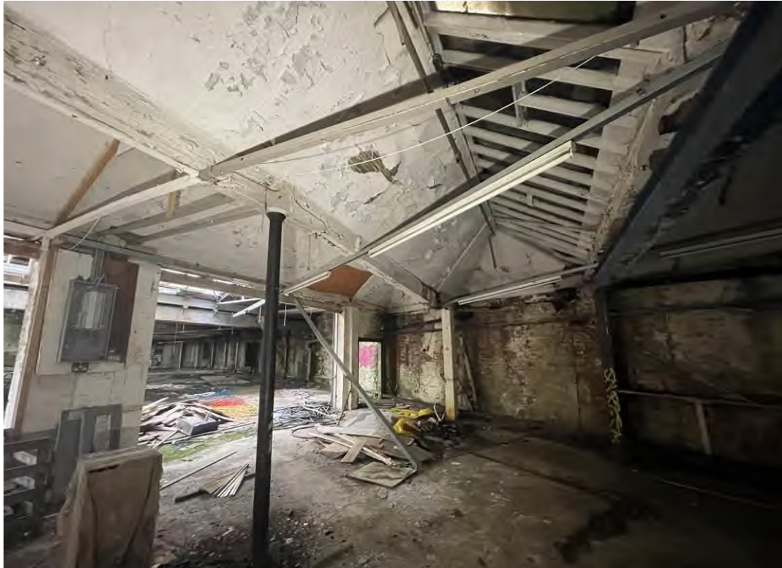
Figure 64: Looking north-west across the eastern part of the c1860s shed, showing the narrow cast iron columns and north-light roofs.
