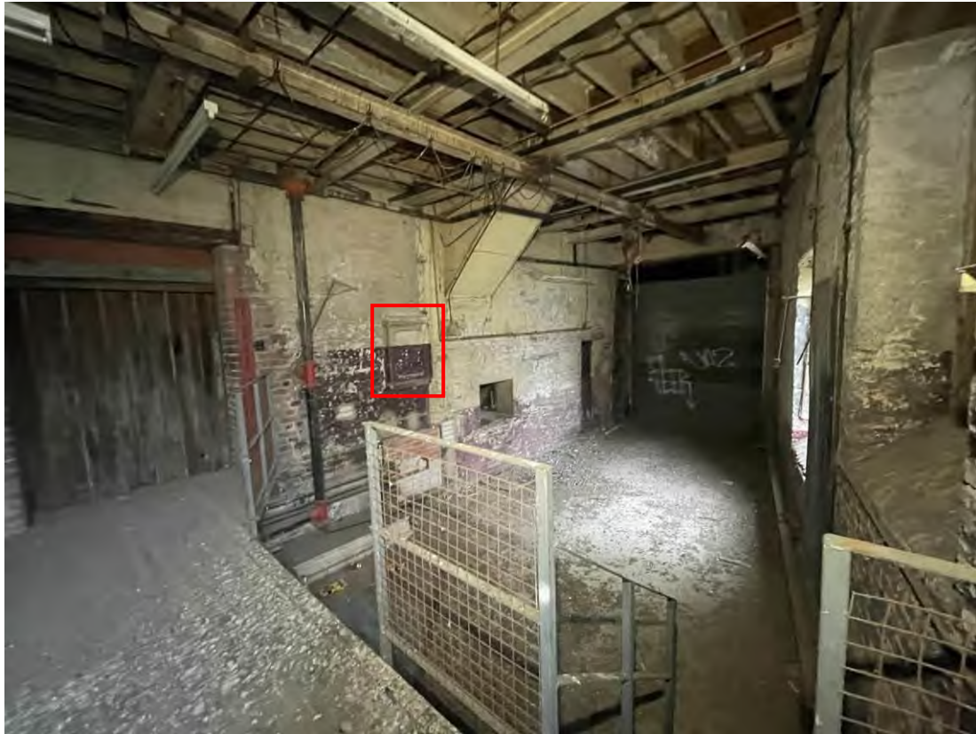
Figure 66: The 1880s curved wing, showing the 1801 mill (left, and River Medlock to the other side of the right elevation. When originally constructed, this was the location of the mill's engine house – part of the original cast iron wall opening for the beam engine can be seen highlighted (see Figure 57 above).
