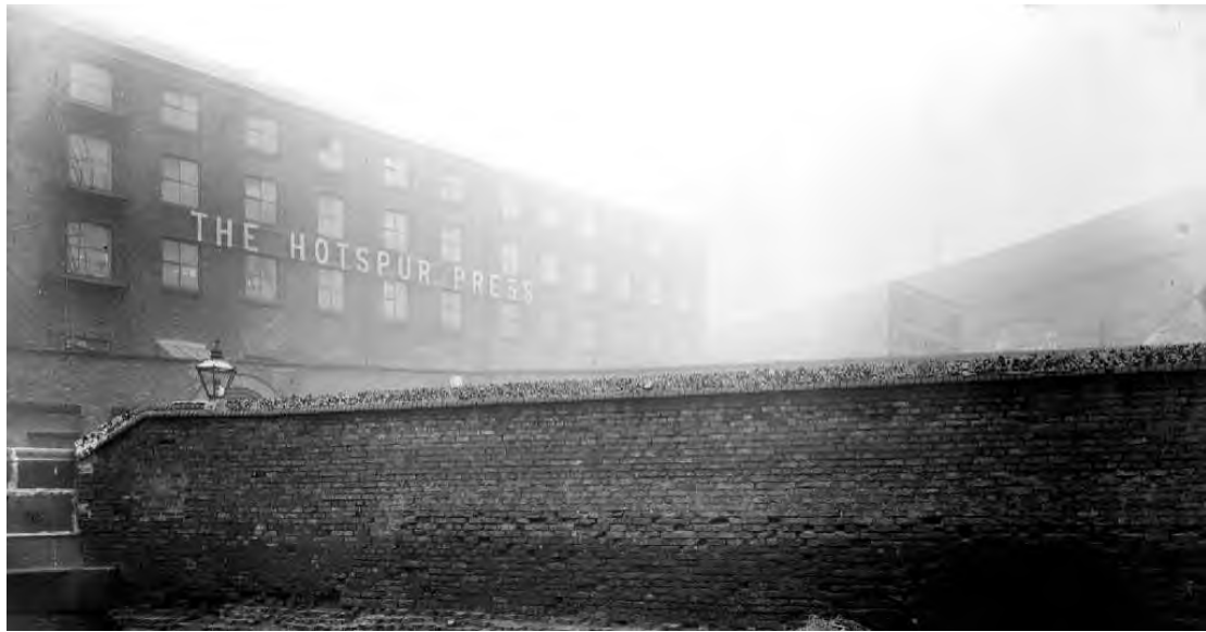
Figure 19 – A view looking across to the eastern elevation of Medlock Mill in 1903, showing a piece of early wall to be removed to allow for the Cambridge Street bridge to be widened. Note the early cast iron fire escape (far left) and original signage 'THE HOTSPUR PRESS' which still survives today. (Source: Manchester Archives)
