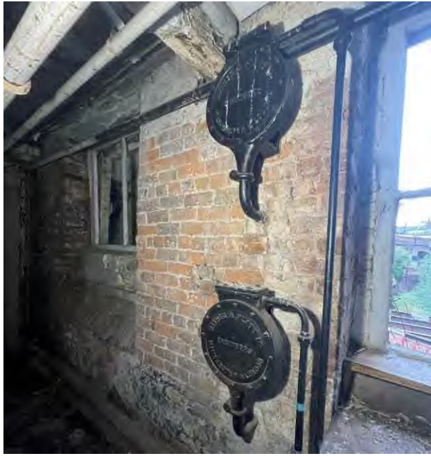
Figure 74: remnants of early heating system to the 1801 block.
