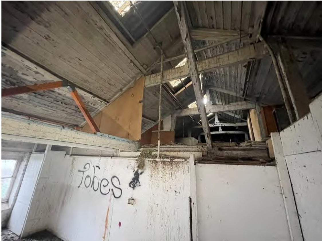
Figure 79: Looking south, showing the modern stud partitions.
