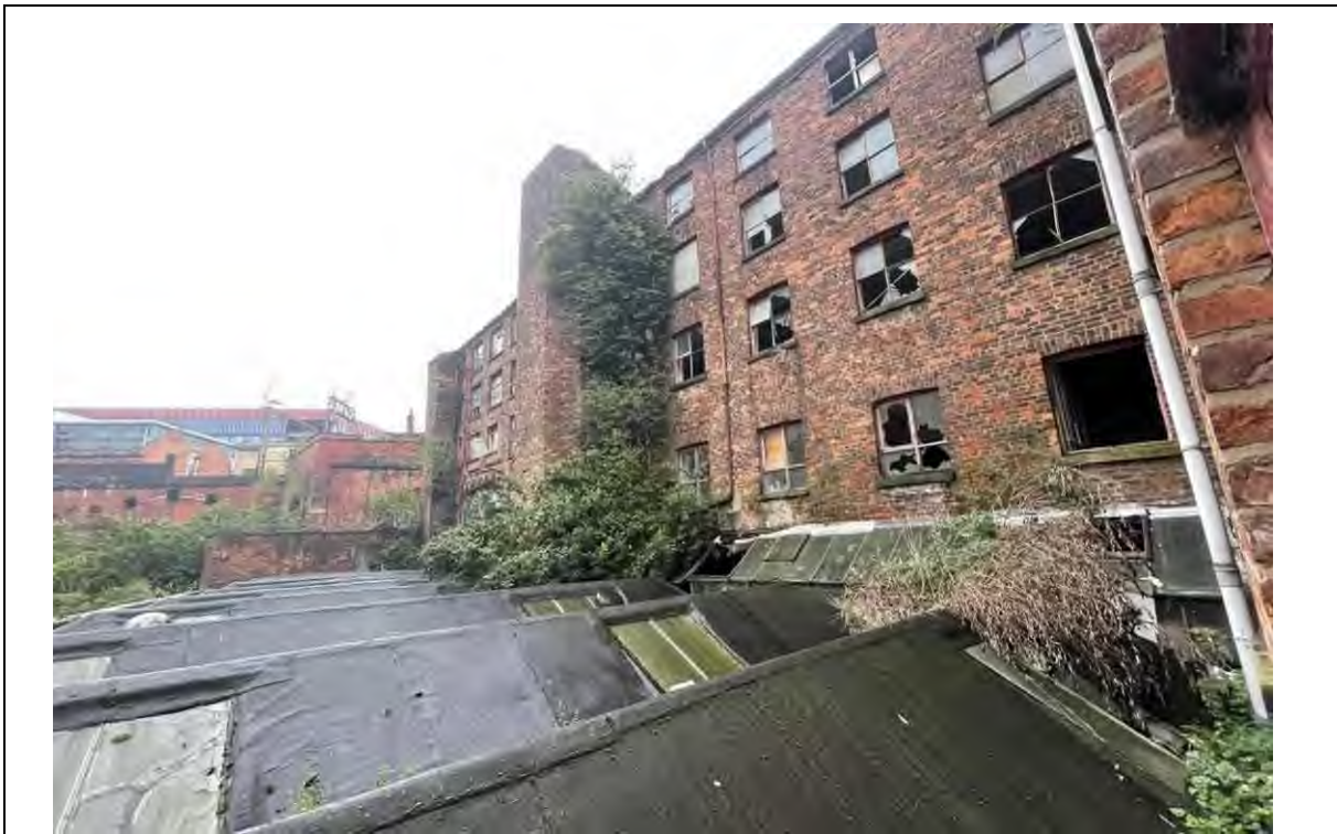
Figure 47: A view looking north along the rear, western elevation of the 1801 mill building from the first floor of the 1880s curved wing, showing the originally glazed roofs of the 1880s sheds below.
