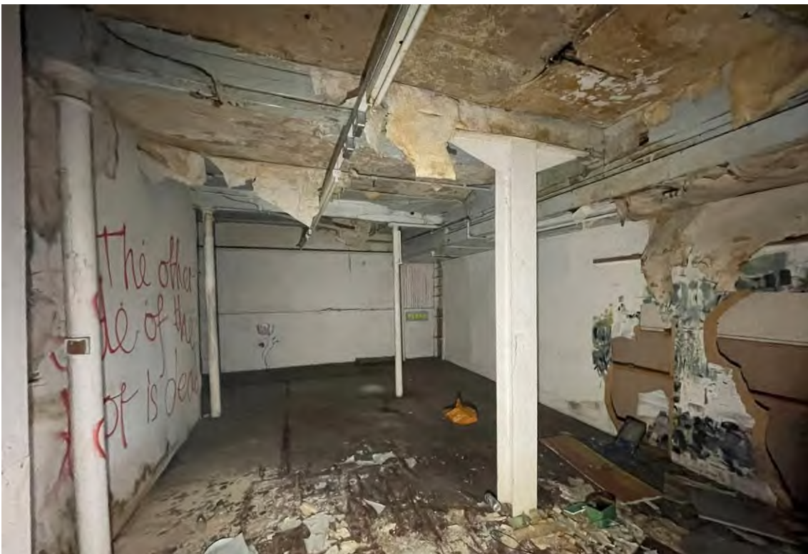
Figure 69: Example of mid-20 th century inserted strengthening.
