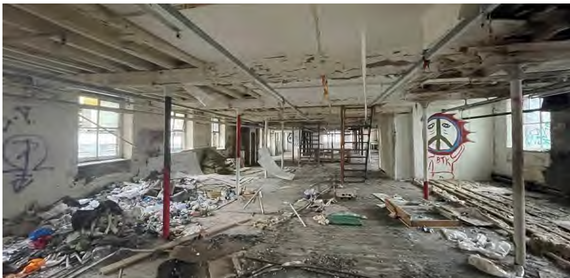
Figure 71: Looking north along the length of the 1801 building.
