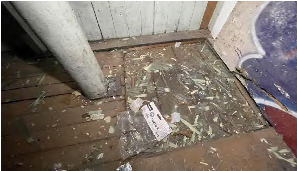
Figure 54: An area of original timber floorboards that are exposed beneath later floorboards to the south-east corner.
