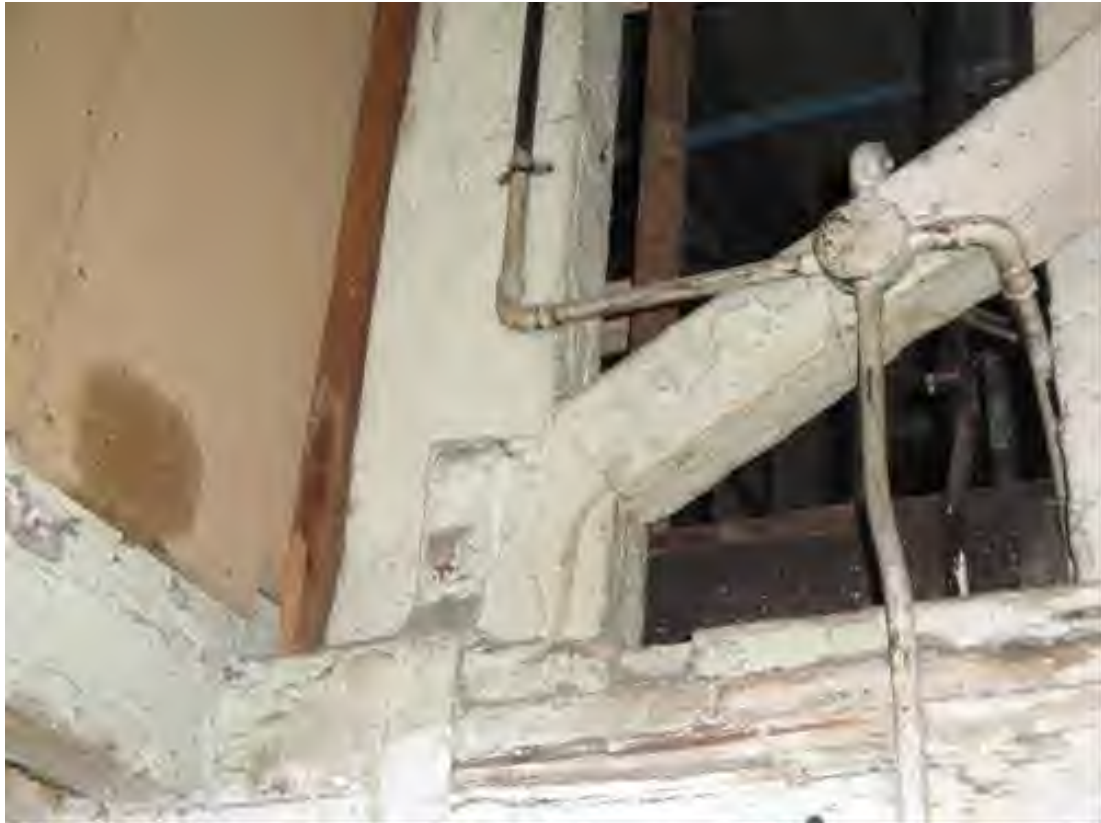
Figure 78: detail of part of southernmost roof truss to fourth floor of 1801 block showing carpenter's mark and notches to allow insertion of a fifth floor within the roof-space.
