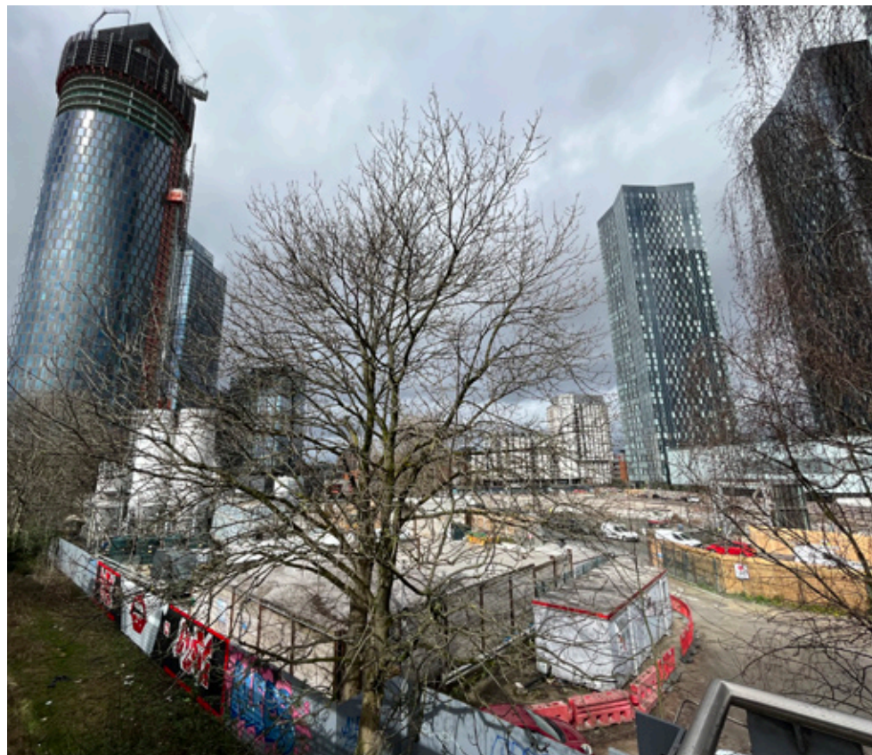
View of the concrete batching plant located on site.
