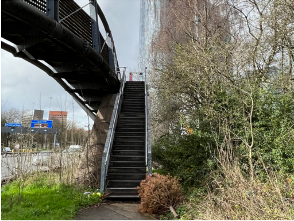
Stepped access to the Mancunian Way bridge.
