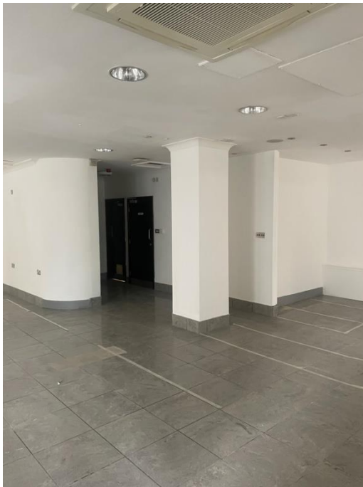
Figure 17: Interior of ground floor unit, looking north across the space. All internal fabric is modern and of No heritage significance.
