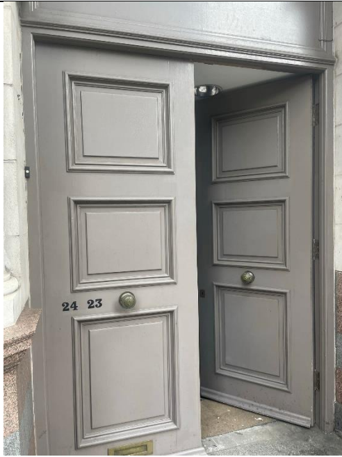
Figure 15: Double door, Mosley Street side, leading into ground floor unit. with arched panel above (featuring signage) No heritage significance. Surrounding stonework of high significance.
