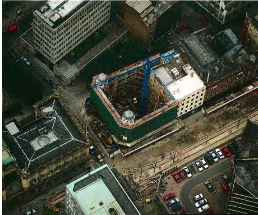
Figure 2 –Colwyn Chambers, c.1991 aerial view. Illustrating the façade retention project underway. As approved in October 1989.
