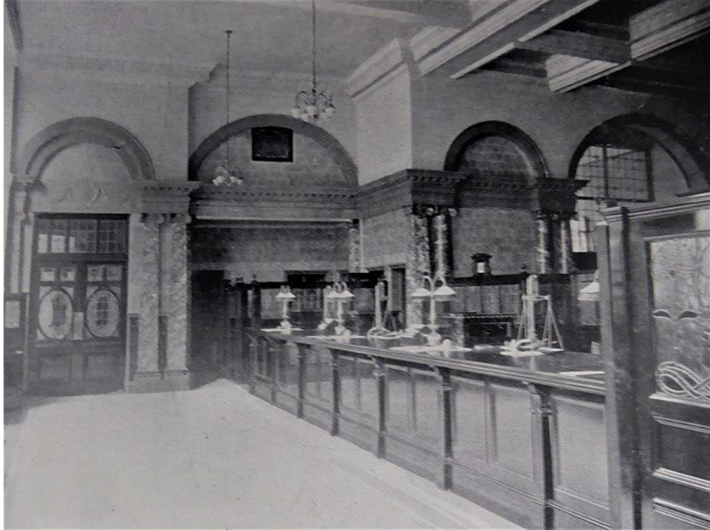
Figure 10: Interior of the Mercantile Bank of Lancashire, Manchester. Space was originally double height with intricate tiling and arched detailing. As illustrated by Figure 2, above, the entirety of these interiors were lost during the early 1990s works. Architect: J Gibbons Sankey. At corner of Mosley Street & York Street, Manchester. Source: https://commons.wikimedia.org/wiki/File:Mercantile_Bank_of_Lancashire_Interior.jpg
