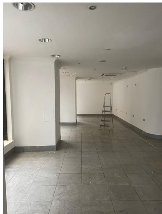
Figure 18: Interior of ground floor unit, looking north-west across the space. All internal fabric is modern and of No heritage significance.
