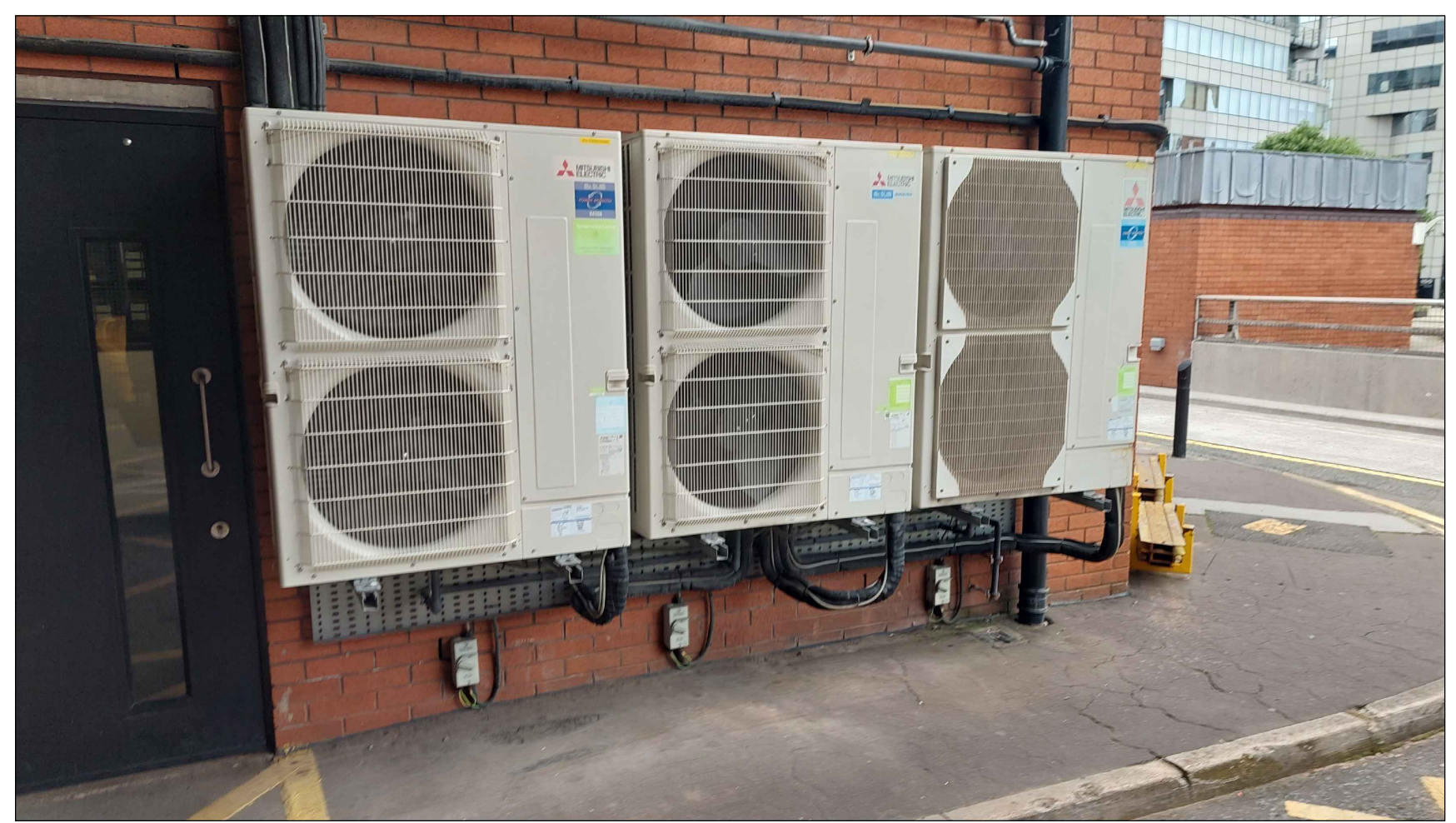
PHOTO 2 - EXISTING 3ND. CONDENSERS TO BE REPLACED FOR NEW. NEW SUPPORT FRAMES SHALL BE INSTALLED IN THE SAME POSITIONS AS EXISTING.
