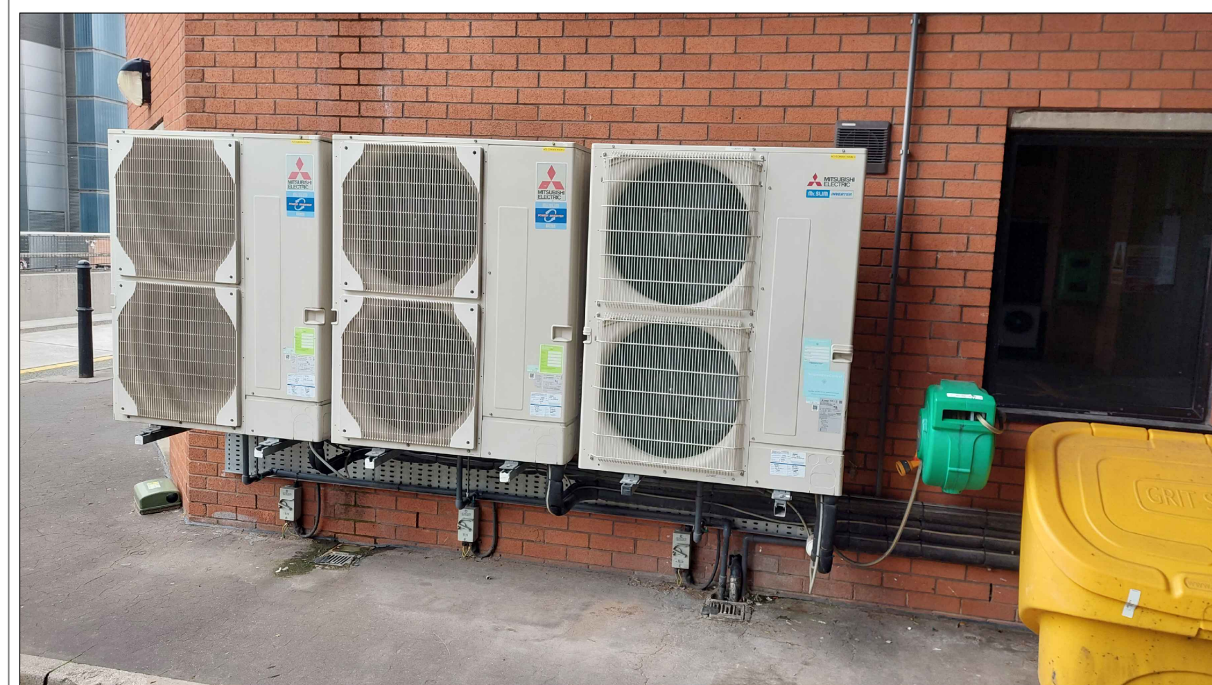
PHOTO 1 - EXISTING 3ND. CONDENSERS TO BE REPLACED FOR NEW. NEW SUPPORT FRAMES SHALL BE INSTALLED IN THE SAME POSITIONS AS EXISTING.
