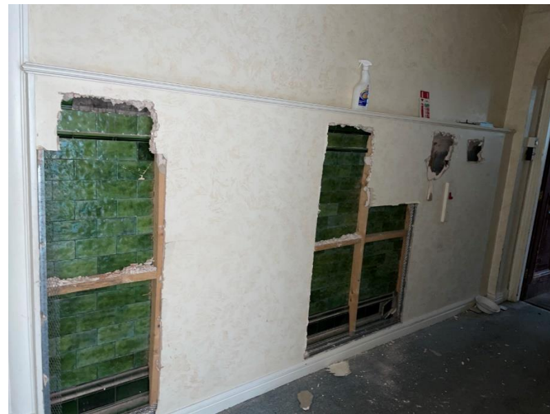
Fig. 13: plasterboard boxing removal – intrusive investigation at 4 th floor level
