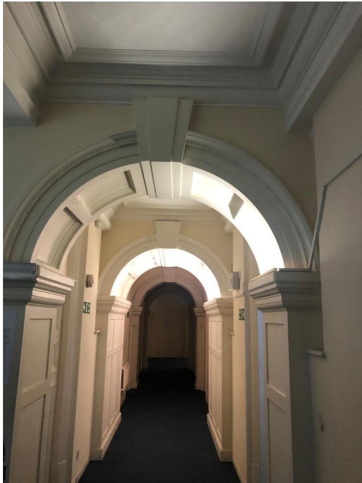
Fig. 12: typical current corridor appearance at 2 nd & 3 rd floors
