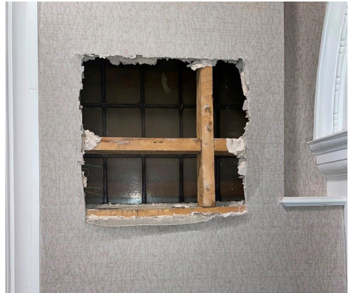
Fig. 15: Exposed internal leaded window at 3 rd floor level
