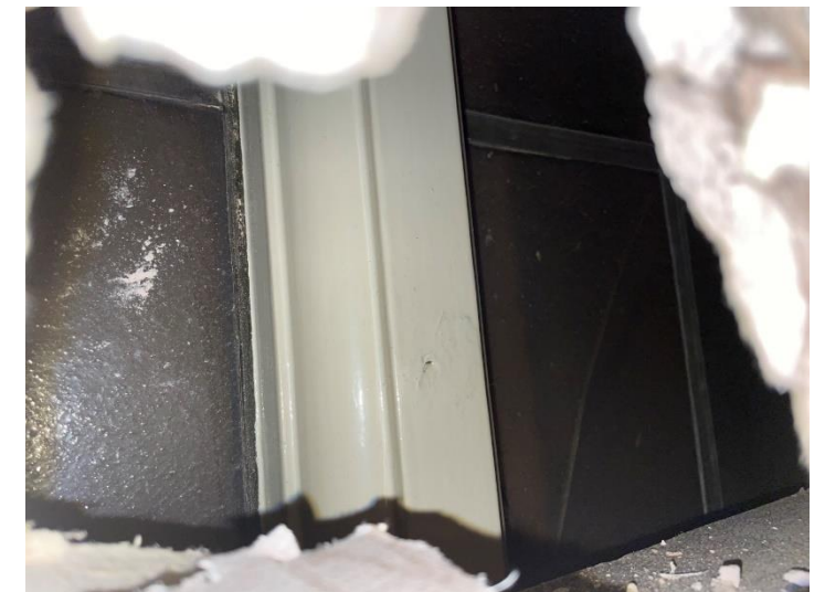
Fig. 16: typical investigative holes at 3 rd floor level showing similar tiling below dado level and internal windows above dado level
