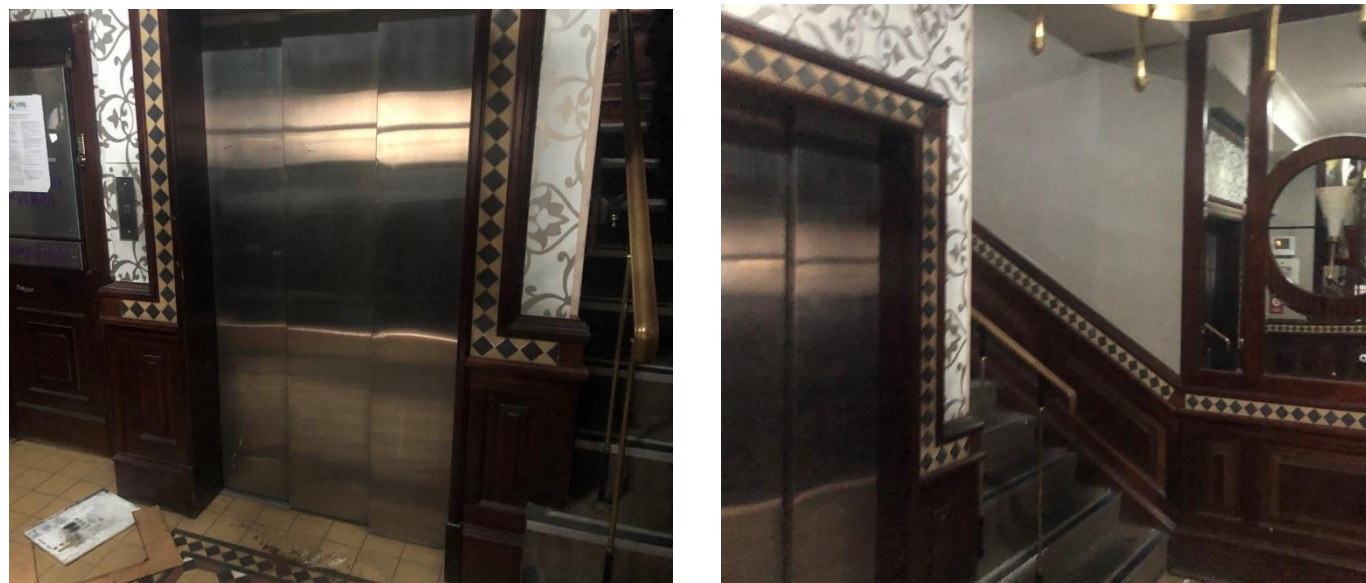
Fig 10: Lift shaft and stair well at ground floor level
