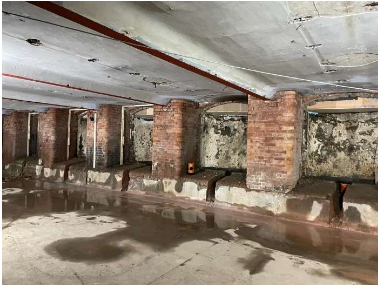
Photo 2: Internal view on the south wall of the warehouse, south block. The chambers can be seen between the pillars forming the external wall at that level.
