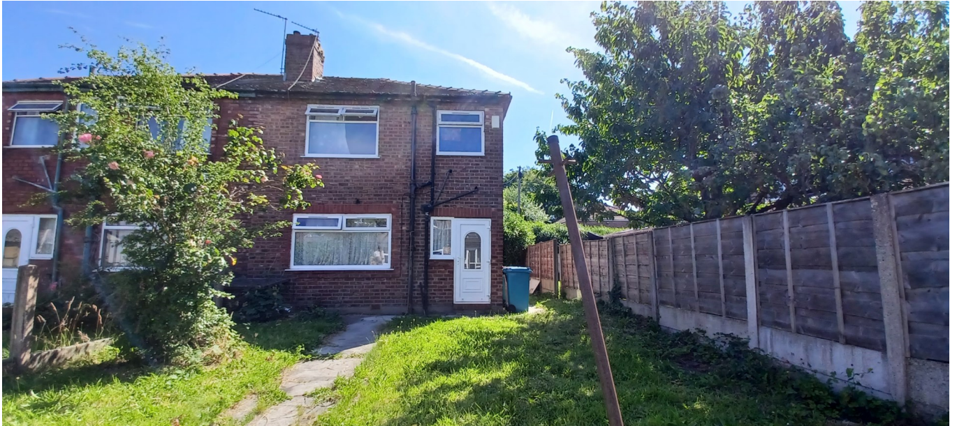
Figure 2. Rear elevation of No.1 The Grange.
