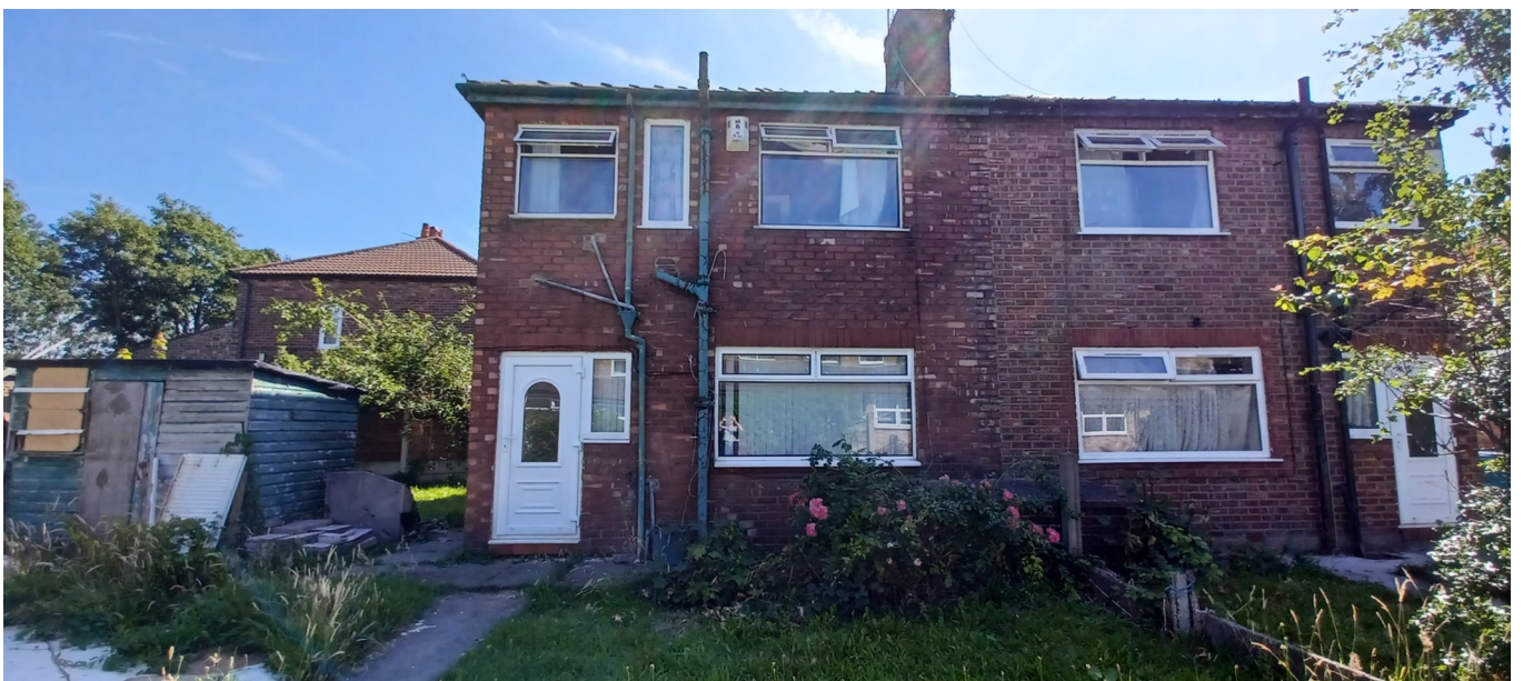
Figure 4. Rear elevation of No.3 The Grange.
