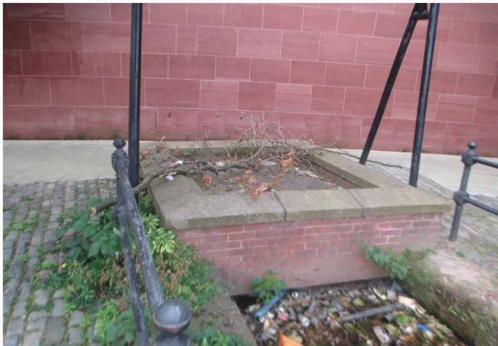
Figure 2 – inspection chamber location adjacent to Castlefield Basin Canal
