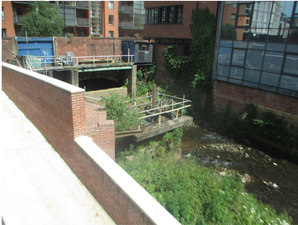
Figure 1.0 – End of River Medlock at Knotts Mill (Where Culvert commences)
