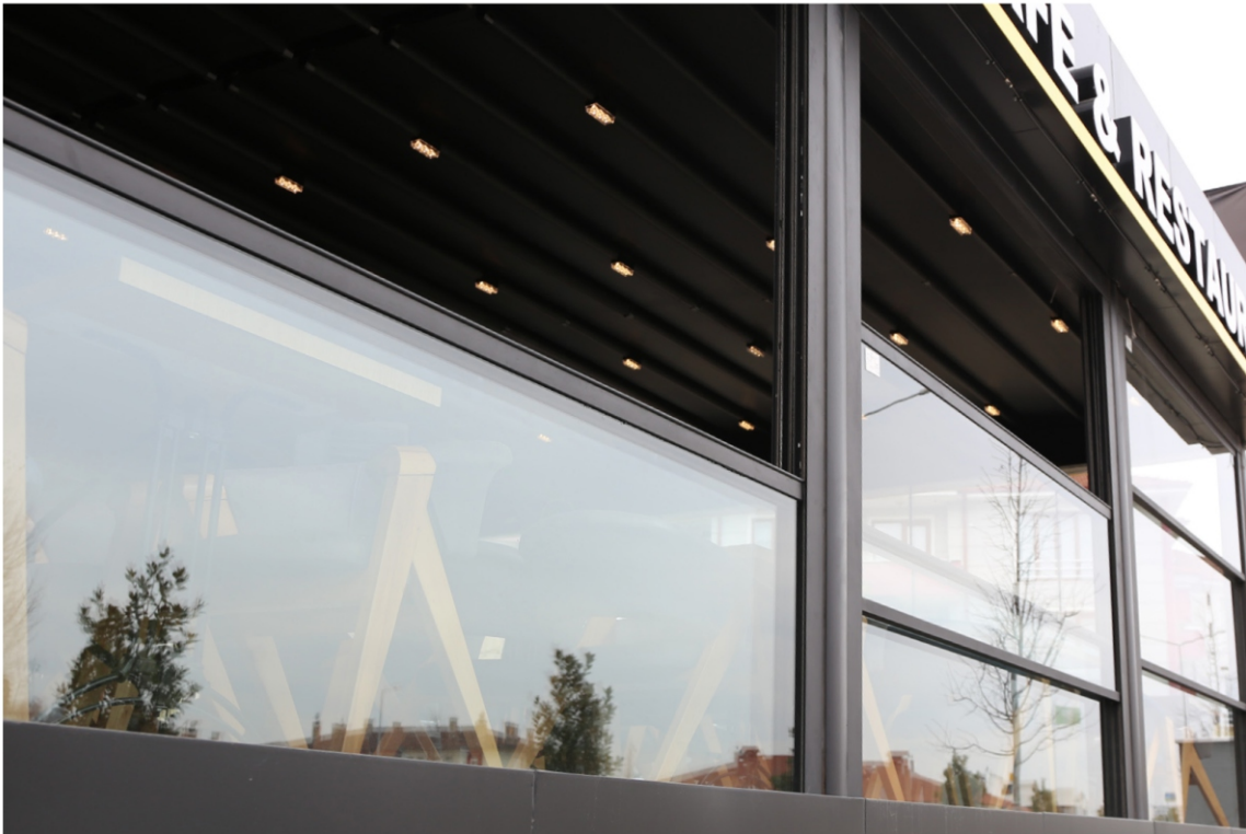
Guillotine glazing. Aluminium Frames / Toughened glazing
