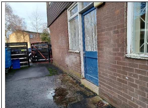
Current Area reserved for bins.
