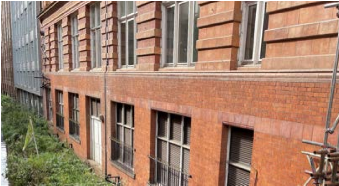
Figure 36: The southern elevation facing the Rochdale Canal, showing the inserted c1966 metal-framed windows into the original timber frames at ground floor level.
