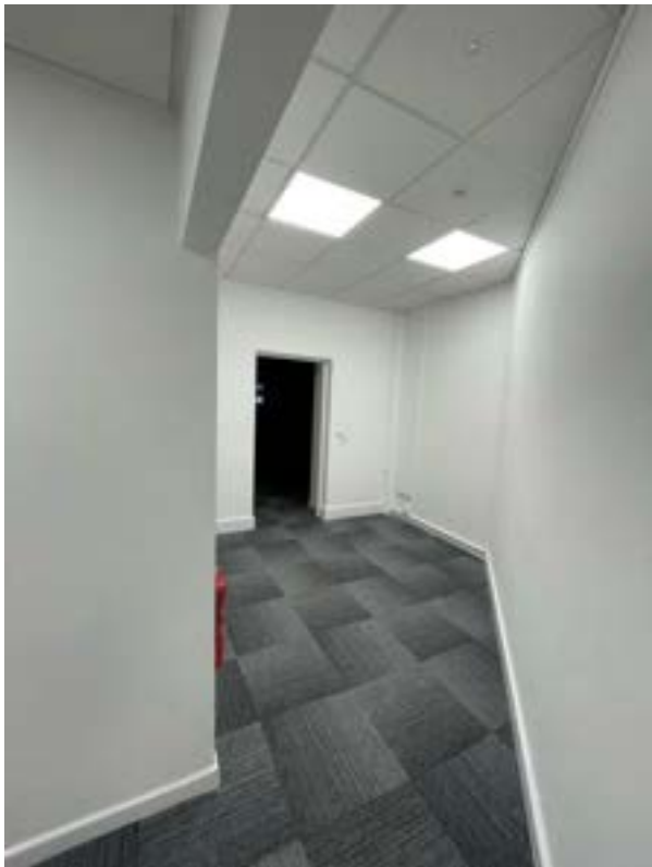
Figure 27: A modern studwork corridor to the centre of the former counting house office.
