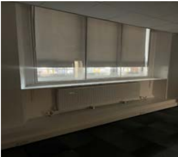
Figure 26: An example of one of the new/refurbished windows facing Oxford Street.
