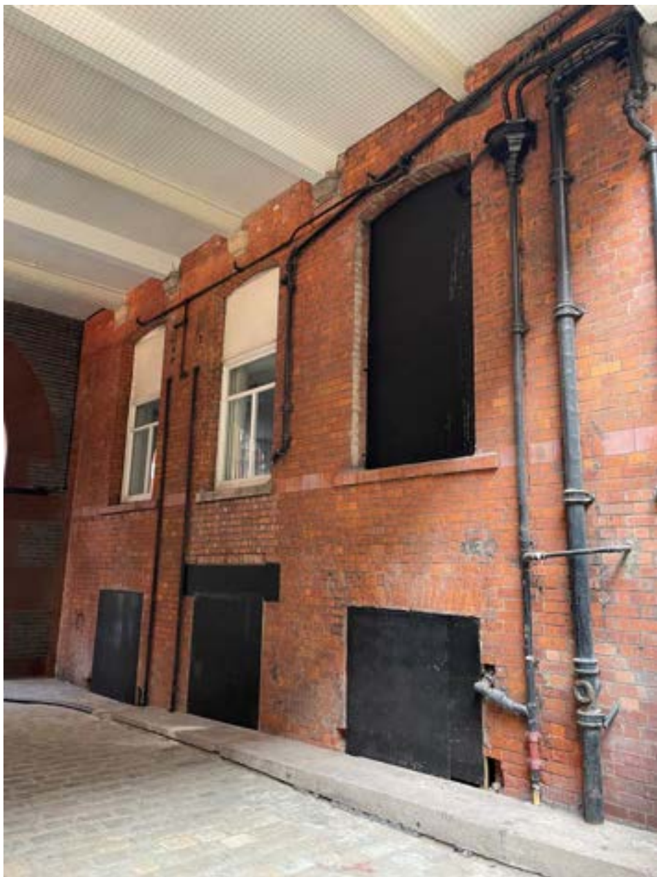
Figure 38: The courtyard elevation to the east of the demise, showing the altered modern windows and central window opening.
