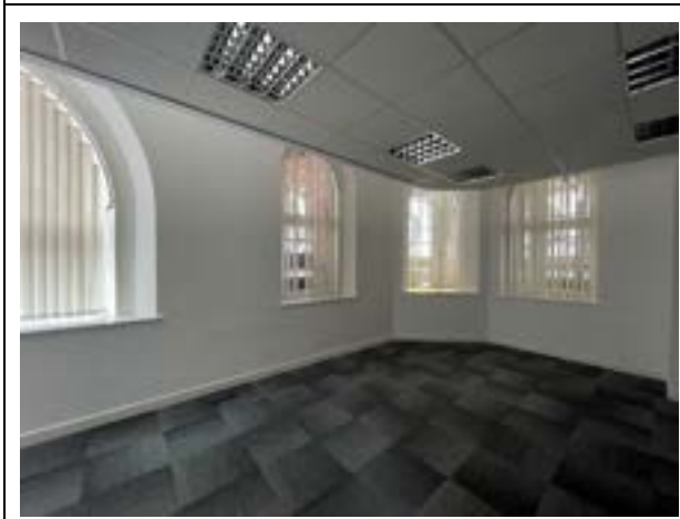
Figure 23: Looking north across the former boardroom, showing removal of all original decorative features.
