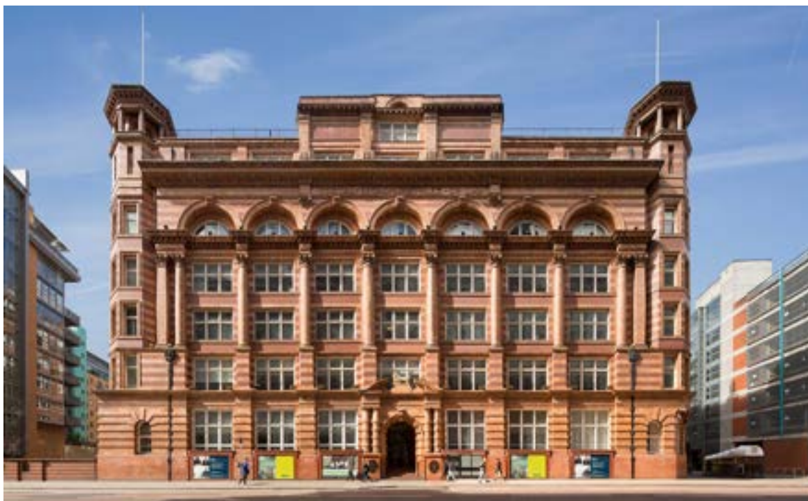
Figure 1 – The principal north-east front elevation as seen from Oxford Street (Source: https://adtworkplace.com ).
