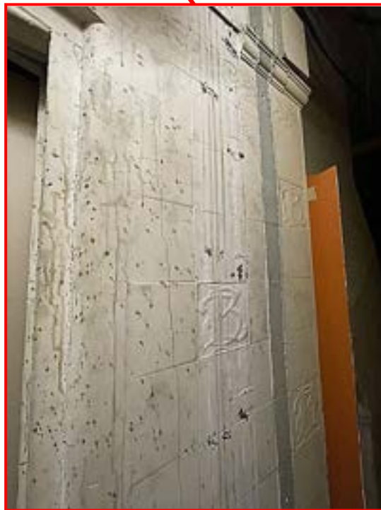
Figure 7: A view looking north across the original counting house office, which now forms part of the southern part of the Site's demise. Note the use of decorative tile to the walls featuring "TBL" initials. The door outlined red is now located within an electrical cupboard and can be seen in the detailed image above. (Source: Historic England Archive)
