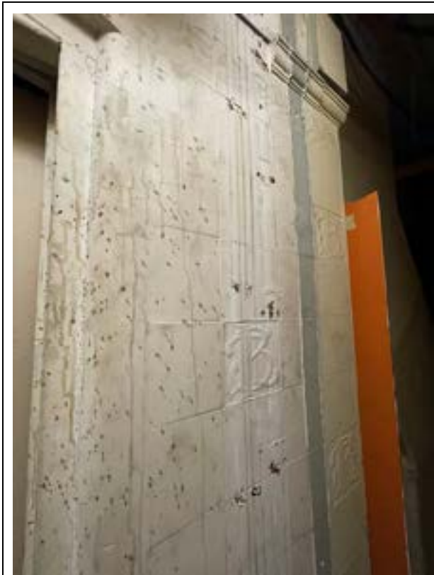
Figure 29: The surviving original iron red glazed tiles concealed within the electric cupboard. Compare to Figure 33 below.
