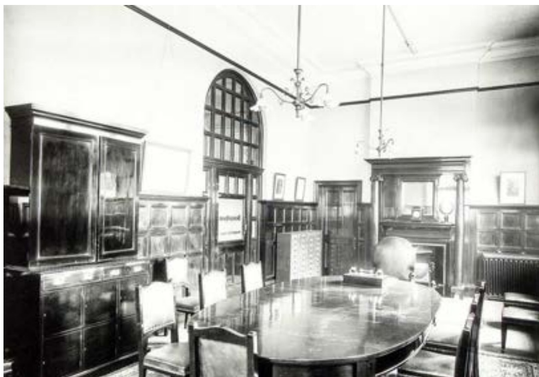
Figure 9: A view of the original boardroom (looking south), which now forms part of the northern part of the Site's demise. (Source: Historic England Archive)
