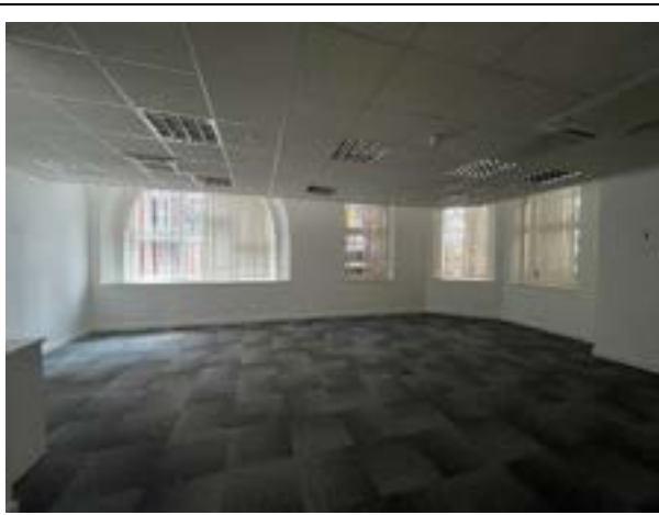
Figure 24: Looking north-west into the former boardroom from the originally adjacent room (walls now removed).
