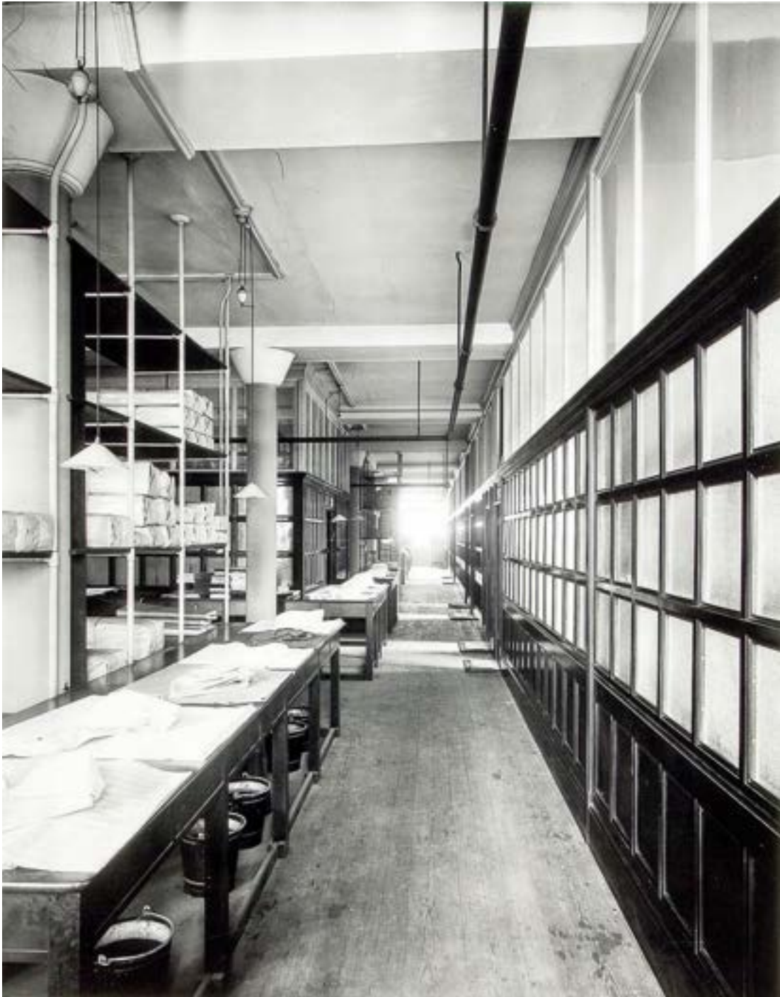
Figure 10: This photograph represents one of the warehouse spaces on the first floor of the building, and illustrates the type of circular, reinforced concrete column that can also be found in the northern half of the ground floor level. (Source: Historic England Archive)
