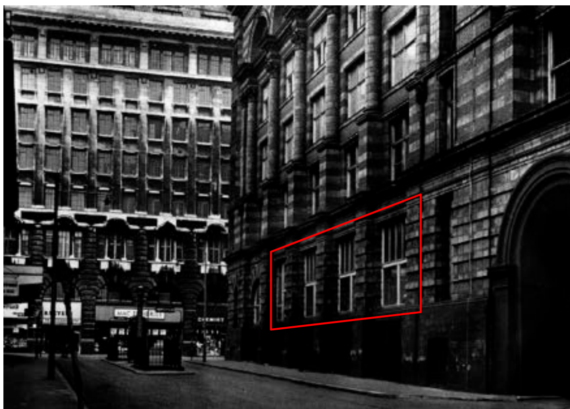
Figure 15: A view looking along Great Bridgewater Street in 1965 showing the four ground floor windows have already been replaced by this date (in the c1950s). The bottom parts of these windows were again replaced with the current windows in the c1980s/90s. (Source: Manchester Archives)
