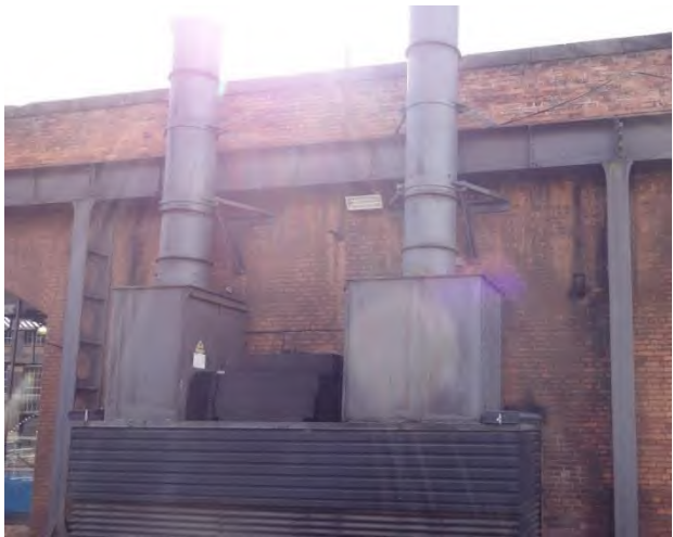
Figure 2-19 – Power Hall chimneys
