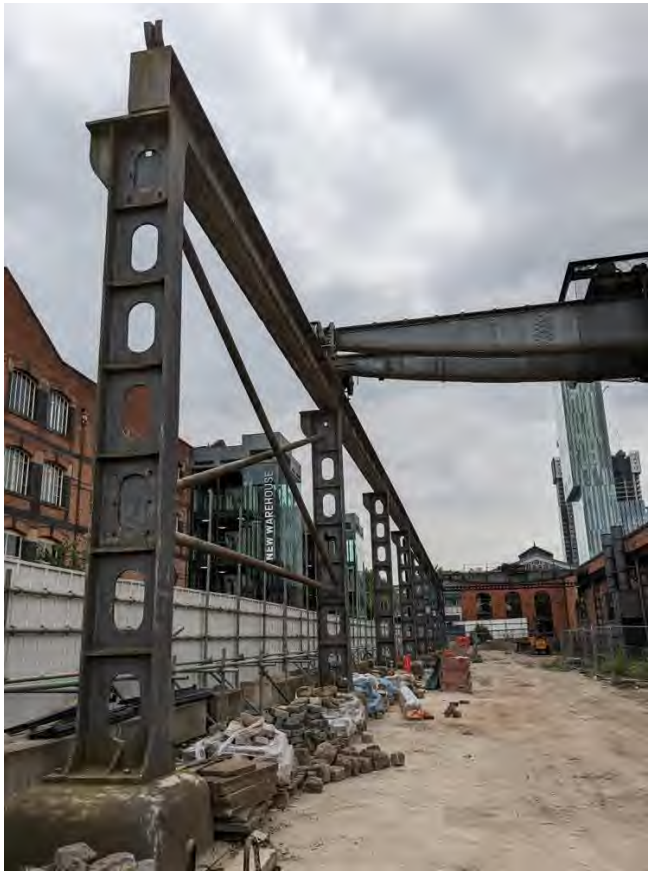
Figure 2-15 North bracing
