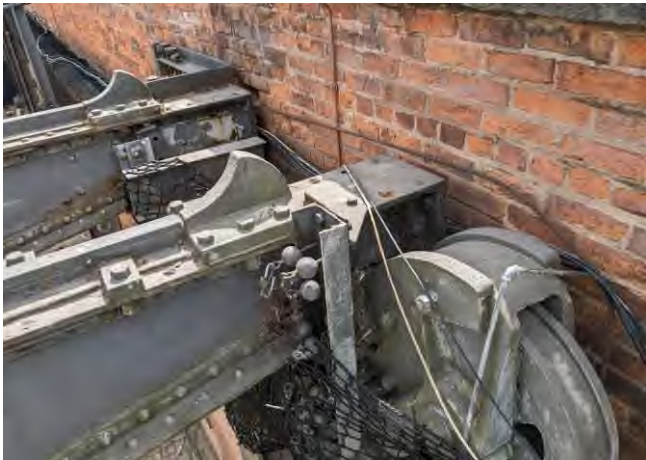
Figure 2-21 – Crane beam support
