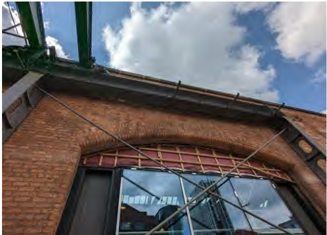
Figure 2-17 South cross bracing
