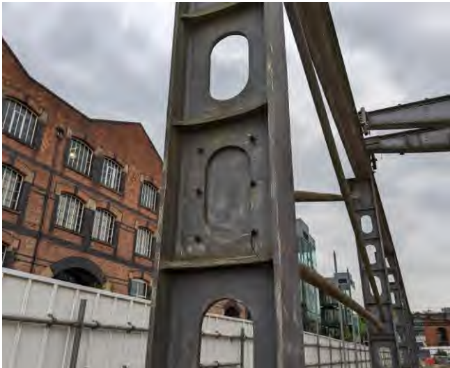
Figure 2-20 – North bracing connection detail
