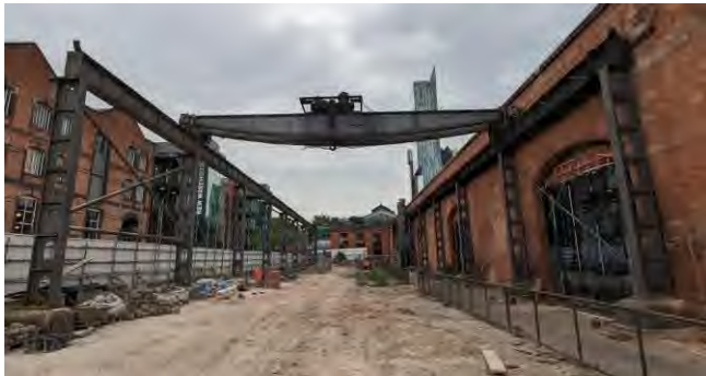
Figure 2-14 General view from west
