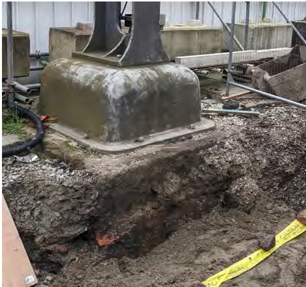
Figure 2-9 Plinth / foundation detail
