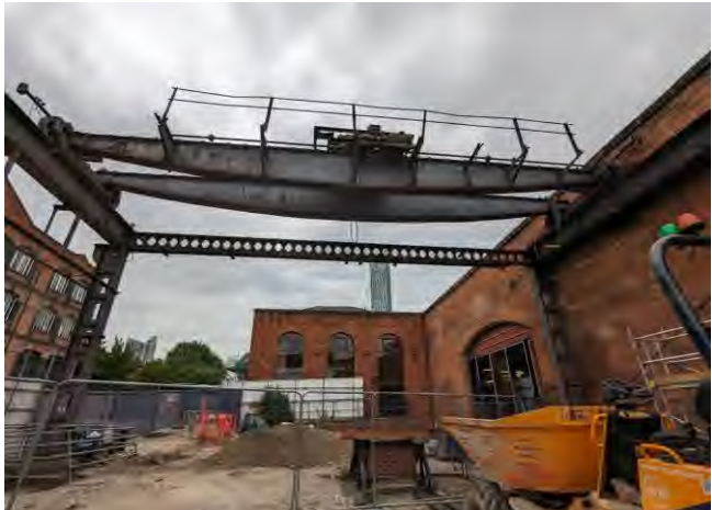
Figure 2-16 Crane beams
