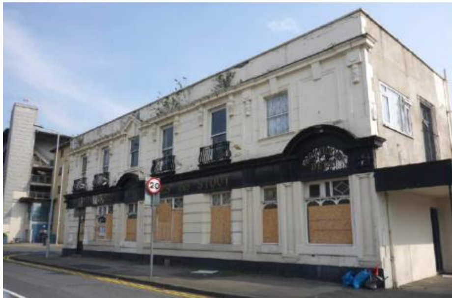
Junction Hotel old Warde Street North Facade
