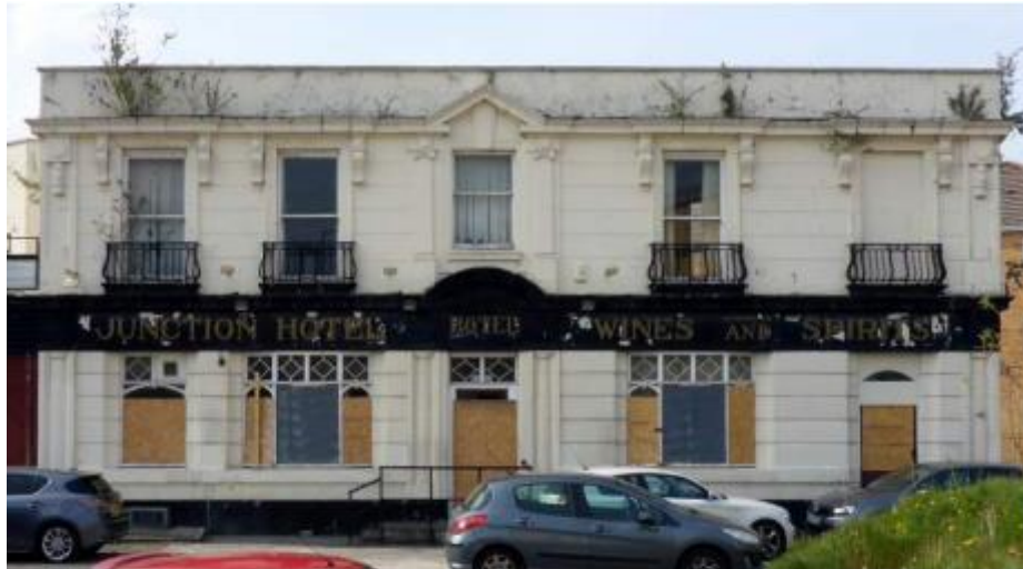
Junction Hotel old Preston Street South Facade
