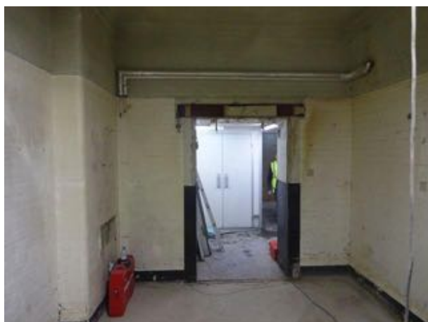
Photo B8 of Walk in Fridge
