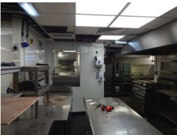
Photo B3 of Kitchen pillar
