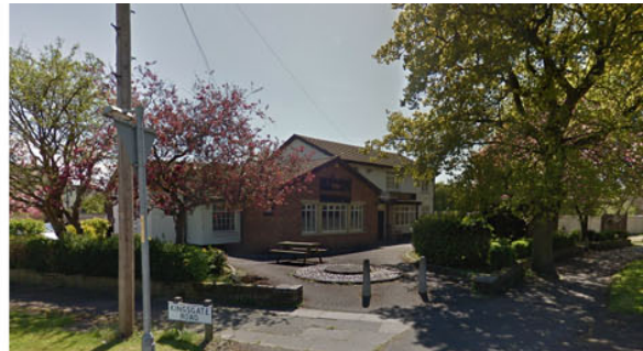
2 – Site From Kingsgate Road / Selstead Road Junction
