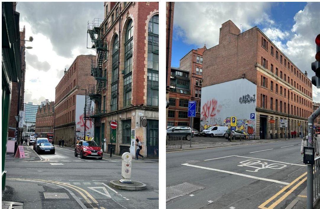
Figures 8 and 9: Views of Bradley House from Port Street
