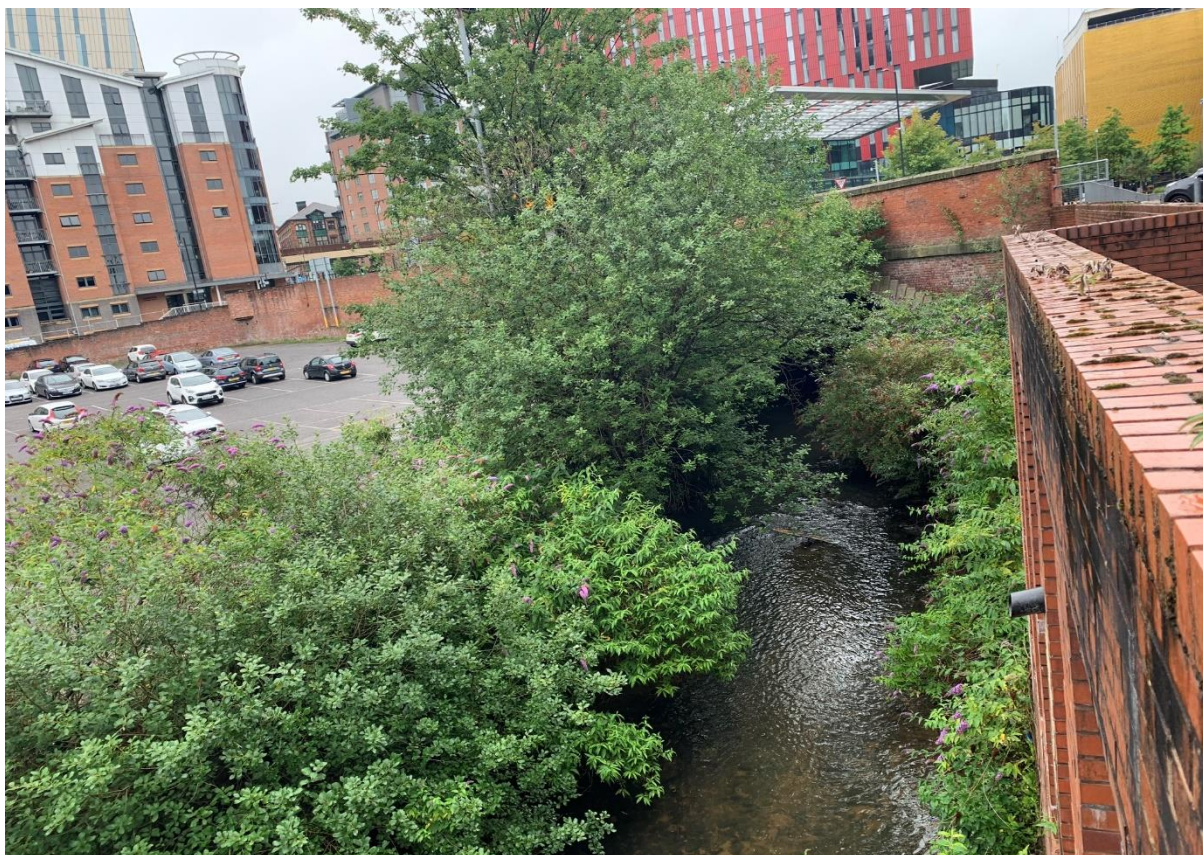
Plate 12 – River Medlock to the North of the Property and Culverted Beneath First Street
