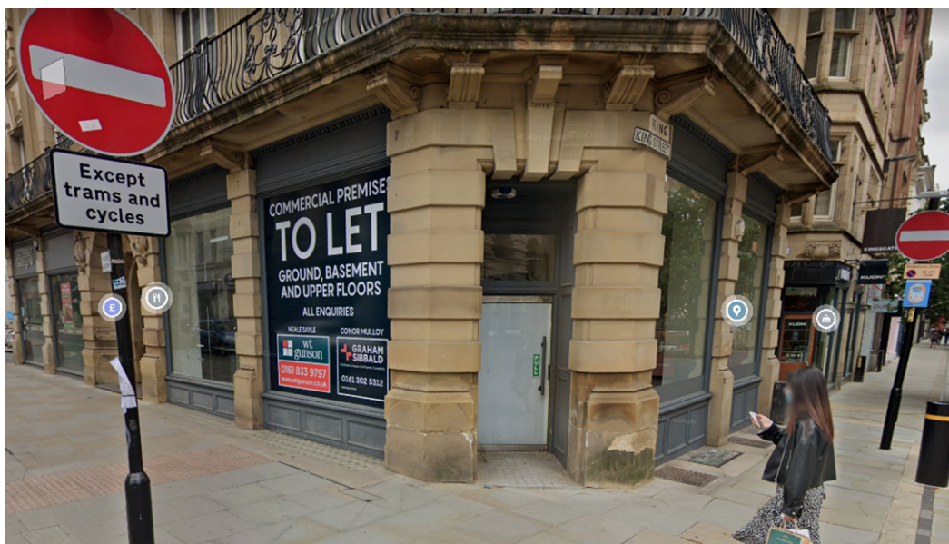
Bulkhead on Neighbouring Unit
