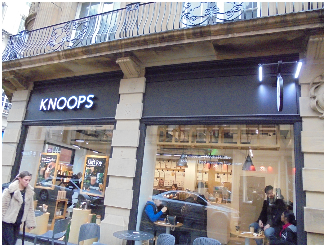
Installed Fascia Signage
