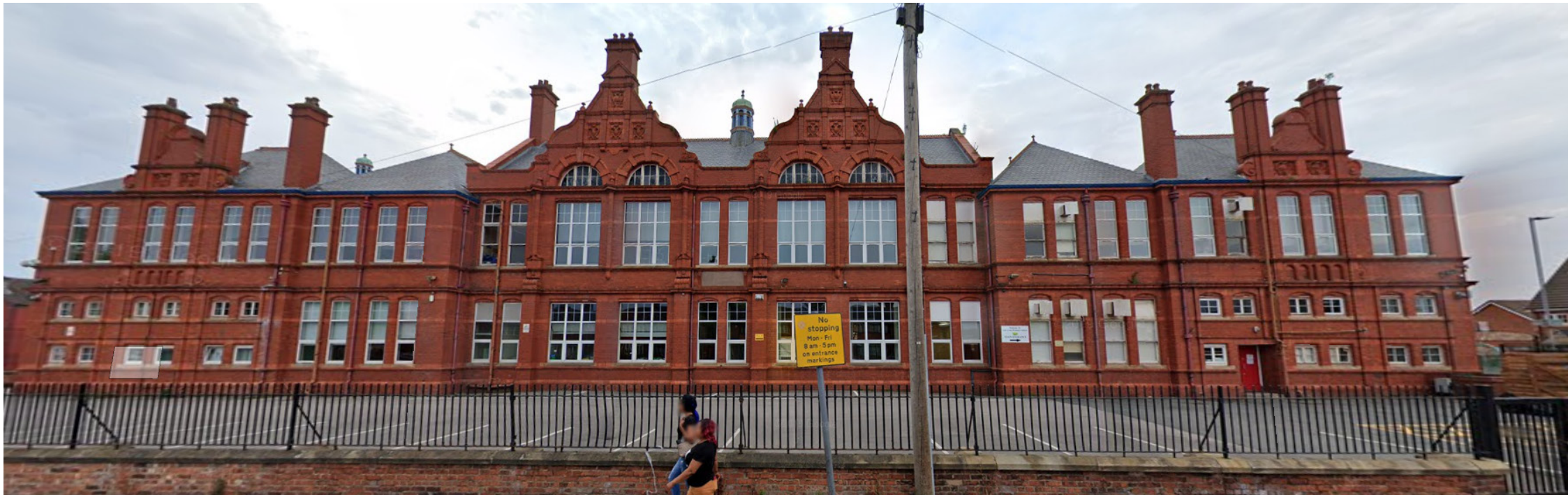
3. Lily Lane Primary School - red brick with expressed vertical elements
