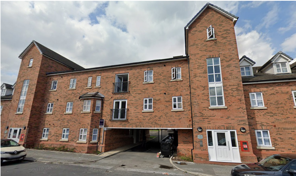
2. Undercroft providing access into the development.
