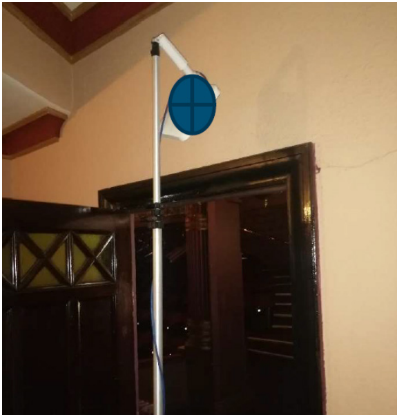
Location AP 36 - Circle Floor one - Unit is at high level and centered on the door in low prominence location.
