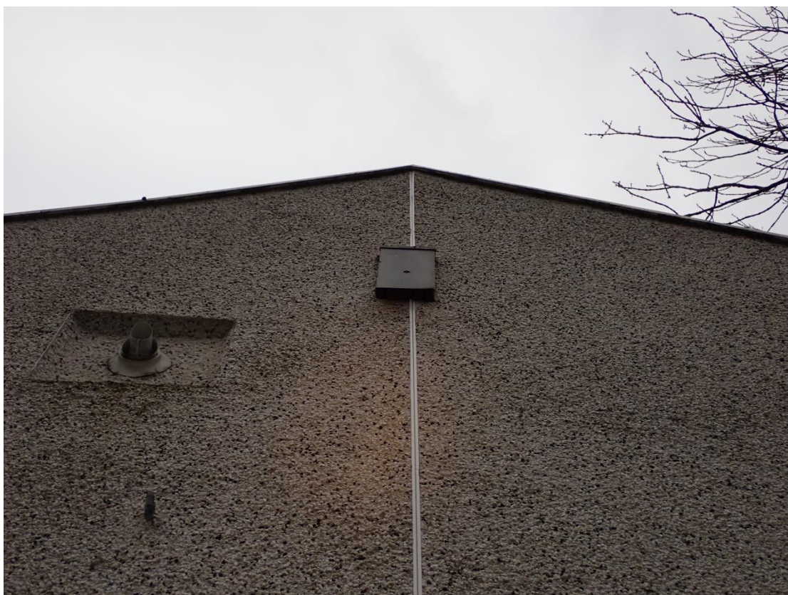
Photograph 7. Electrical box on the northern aspect of the building.
