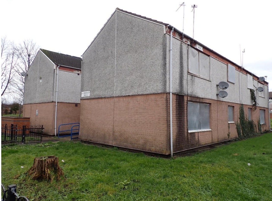
Photograph 1. South-eastern aspect of the building.
