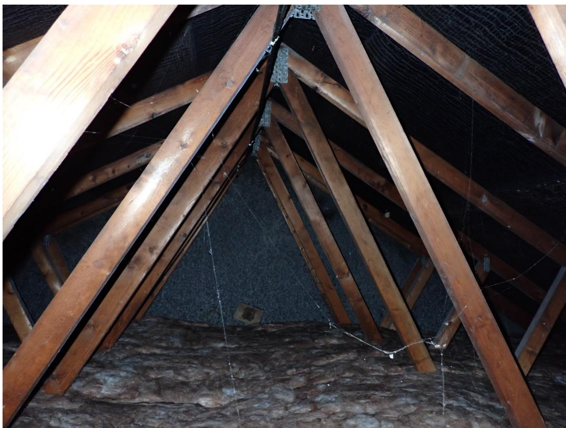
Photograph 11. North internal stone render wall and rock wool floor insulation in Flat 13.
