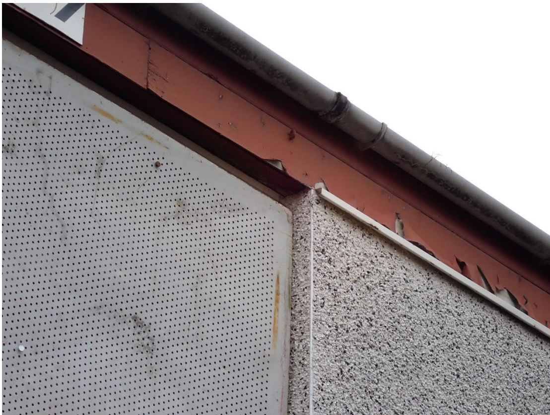
Photograph 4. Wooden bargeboards located at the eaves of the building.
