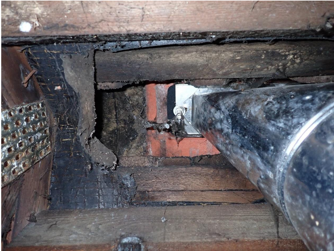
Photograph 9. Ridge tiles are visible around the central ventilation system in Flat 13. The same feature is present in each of the loft spaces.
