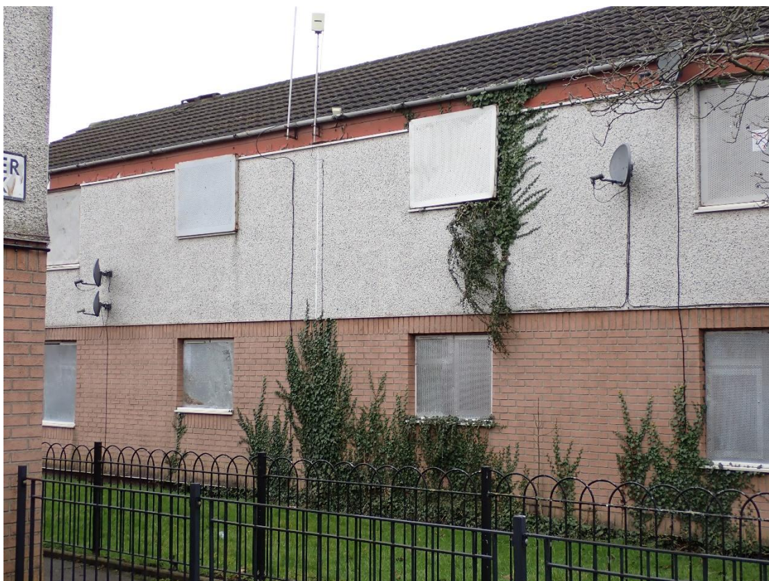
Photograph 2. Eastern aspect of the building.
