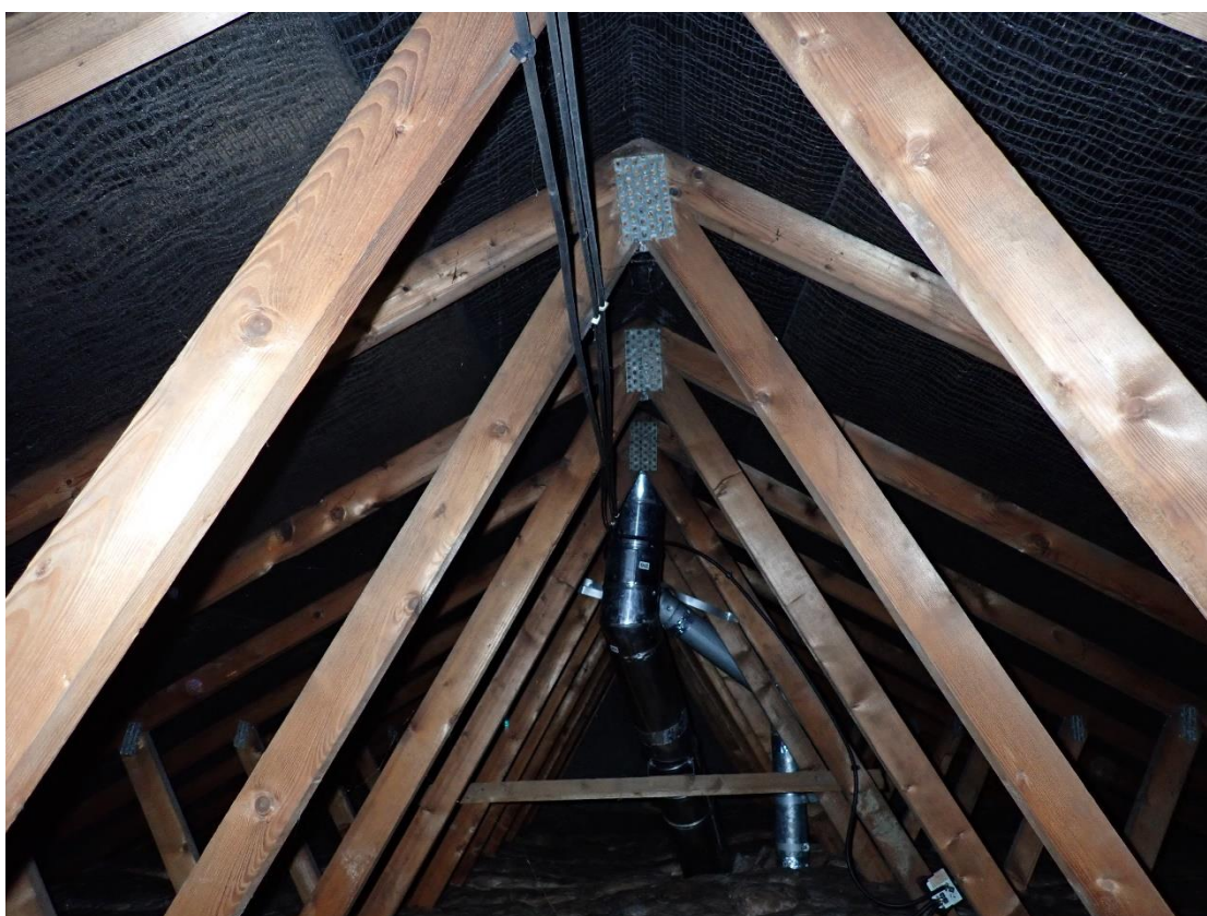
Photograph 8. Loft space of Flat 13; representative of all of the loft spaces in the building.
