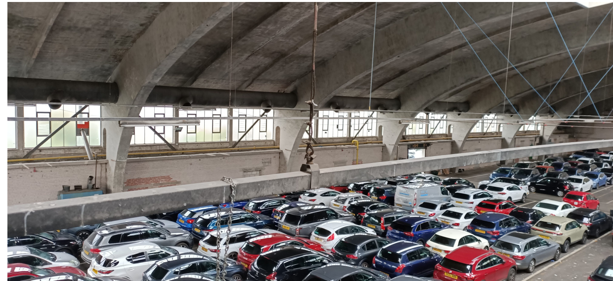
Internal view showing West Elevation windows
