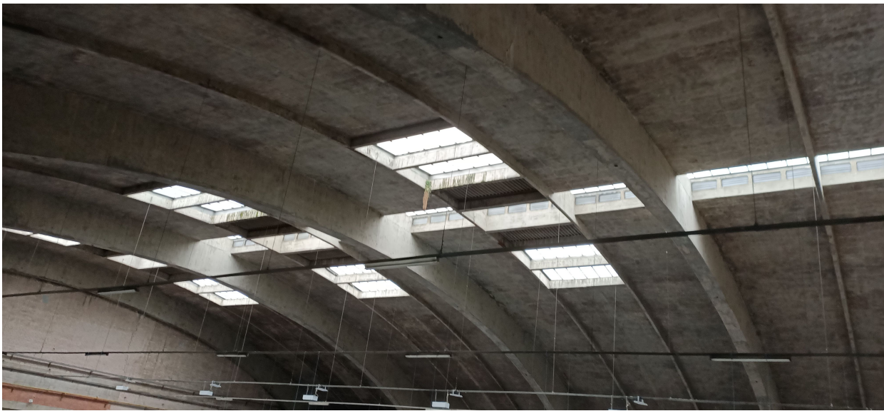
Internal view showing the concrete roof and rooflights
