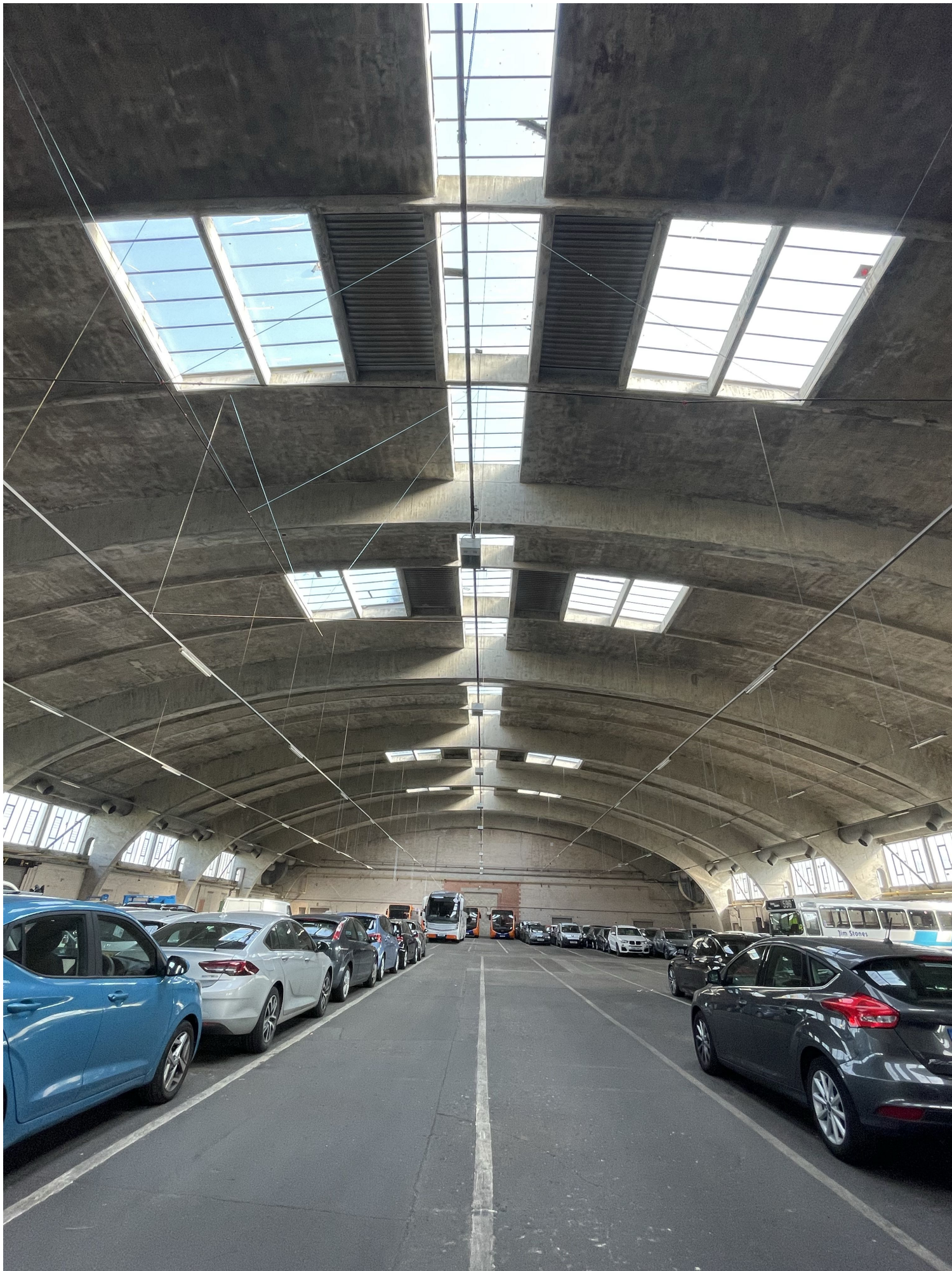
General Internal view from entrance
