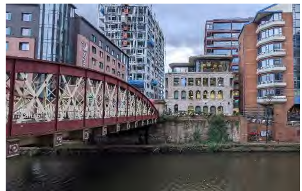
Figure 13: View north from the pedestrian realm on the riverbank, looking across to modern development within Salford. The Grade II listed Irwell Bridge is visible to the west (February 2023).
