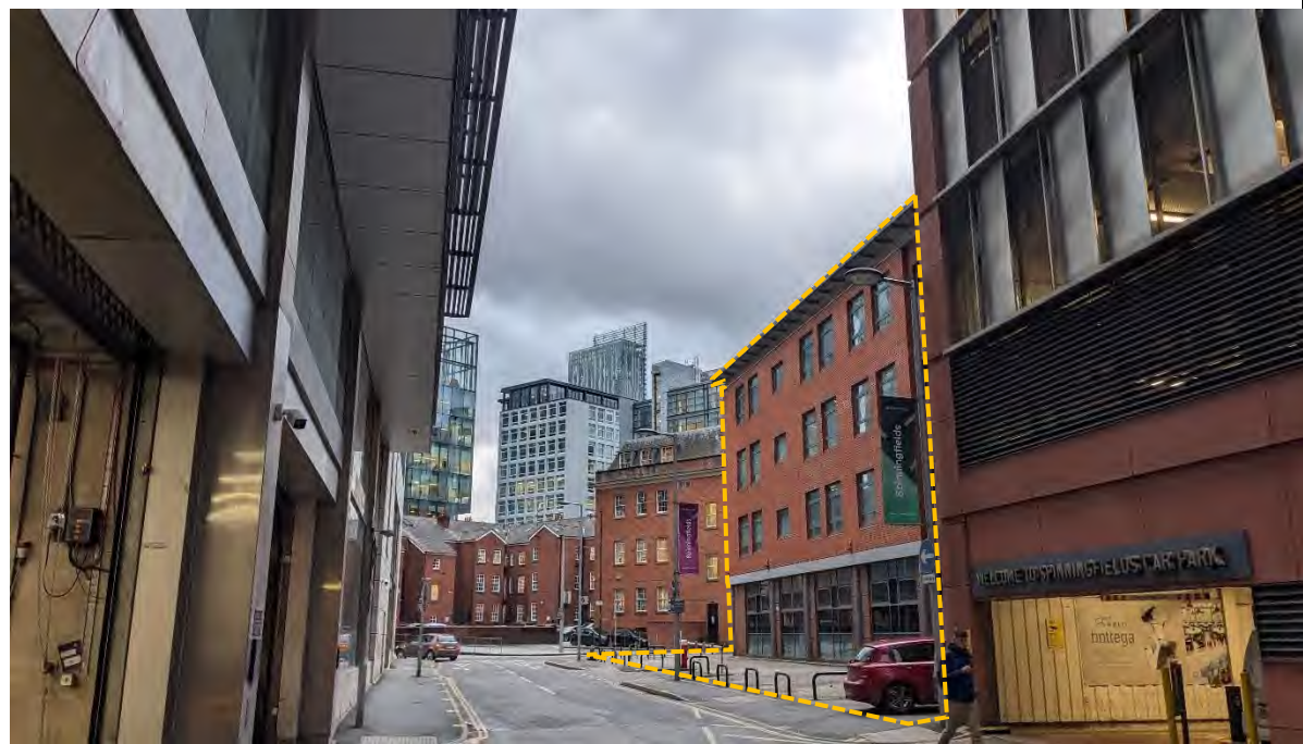
Figure 6: View of the Site's rear elevation and rear car park in its local context, as seen from New College Street to the north-west of the Site (February 2023). Site outlined in yellow.
