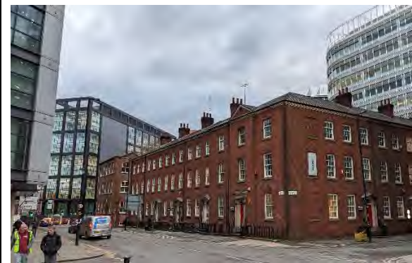
Figure 12: Looking north-west along Quay Street across the finer, traditionally informed building to the east of the Site (obscured from this location). Other, large and modern
