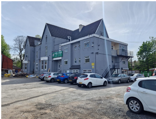
Front elevation of 122 Withington Road, looking south-west. The main entrance lies below the green signage
