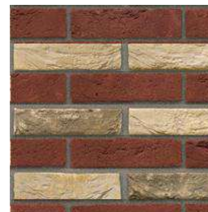
Red and Buff Banded Brickwork
