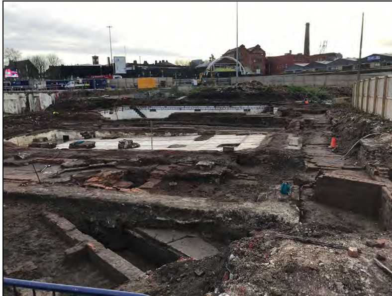
Plate 2.0: Mayfield Baths site following excavation
