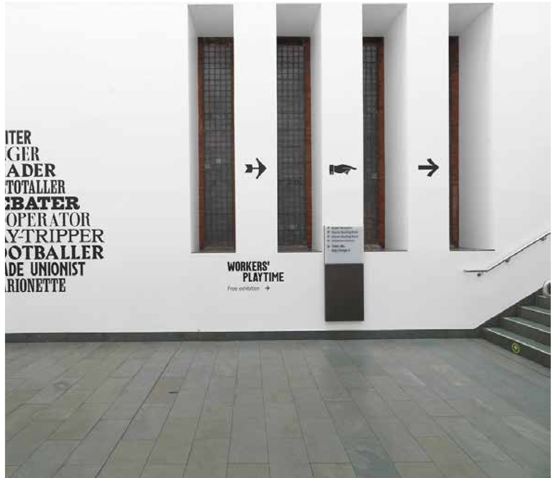
Photograph of existing atrium, including 1920s lancet windows behind modern plasterboard reveals.
