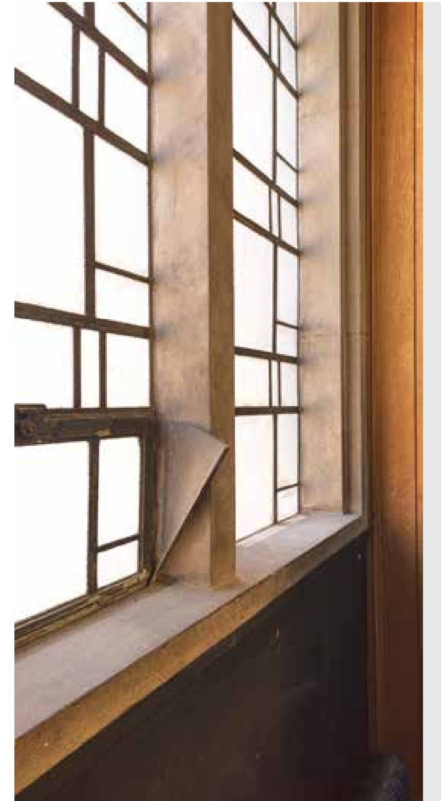
Photograph of existing room, including deep window reveal (where proposed secondary glazing is proposed for installation).
