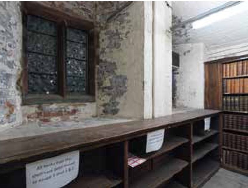
Top left and top right - Proposals for new glazed screen in existing arch, to convert room into Sorting Space. Bottom left - Conditions of current cellar spaces requiring tanking to protect collections. Bottom right - Proposal to bring air circulation into cellars via adapted existing vents in south elevation and new AHU unit.
