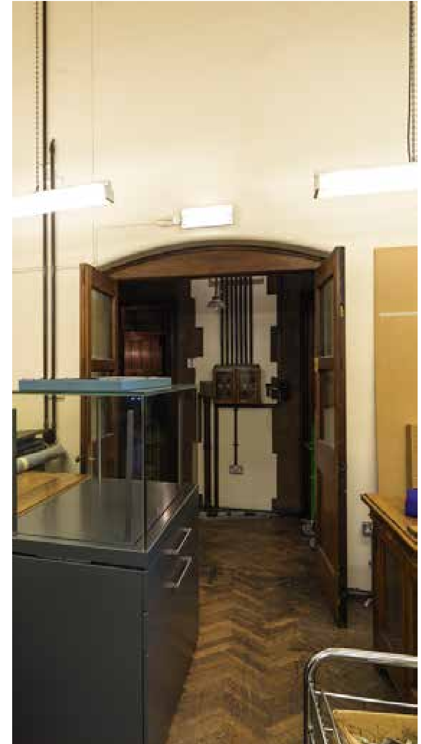
The room which the proposed (yet discounted) lift would have been placed, including the historic floors and walls which would have required breaking through.
