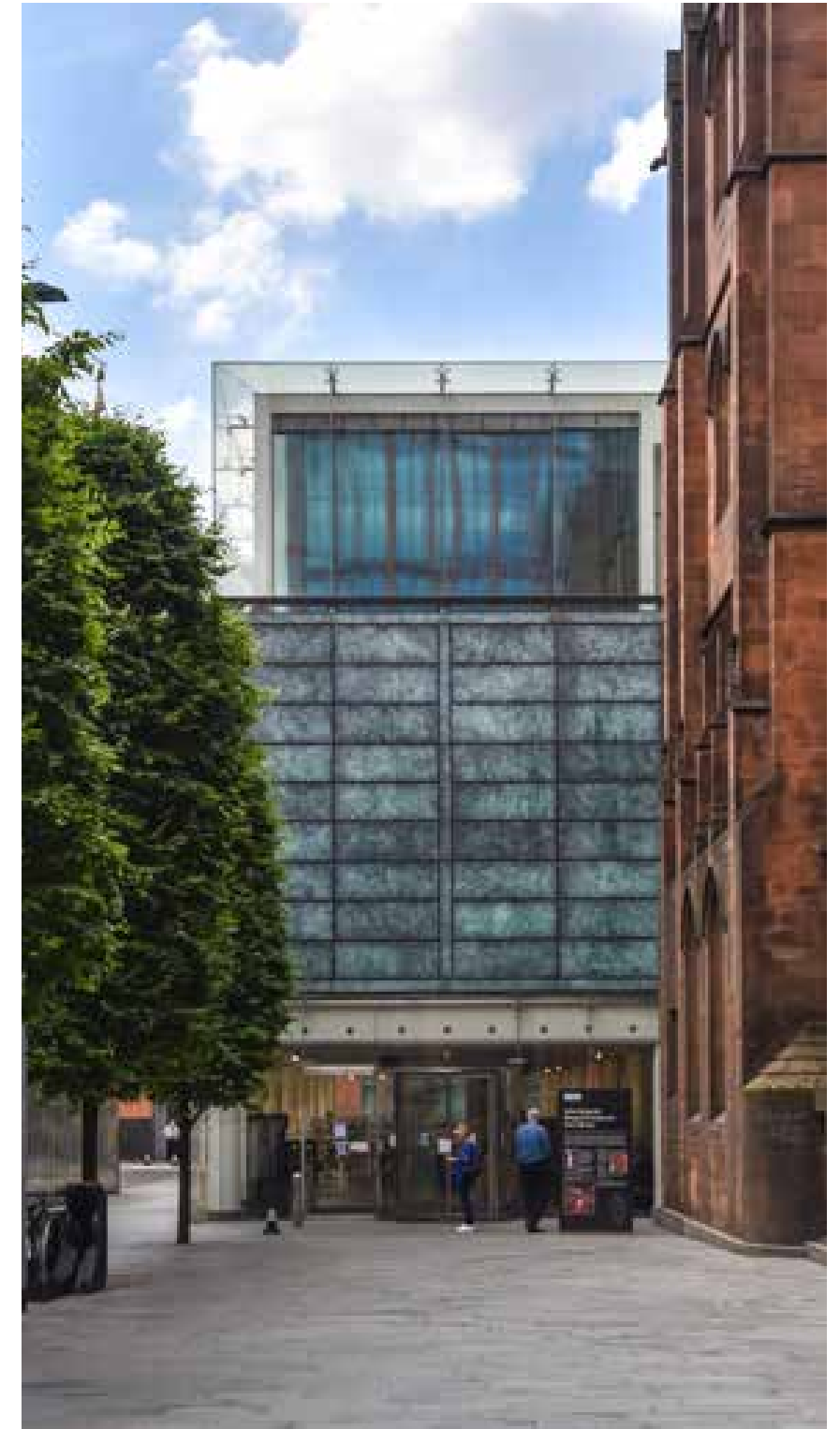
The modern entrance to the Rylands, with the modern reading room above; part of the 2007 extension.
