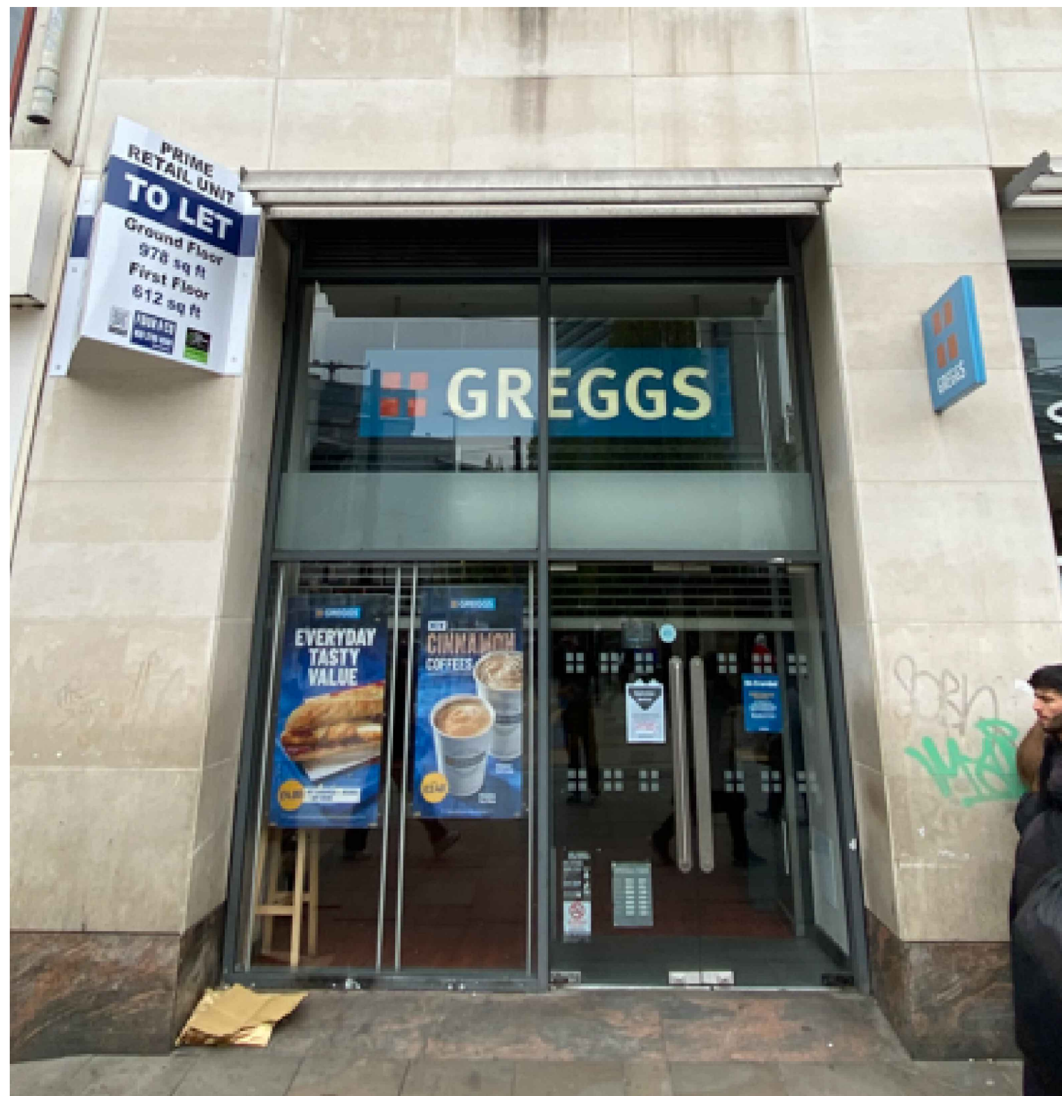
SHOPFRONT (EXISTING - APRIL 2023)
