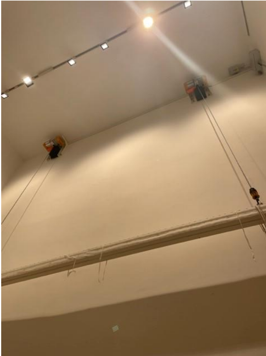
Photo 4. Existing hoist showing cables, lifting bar and motors
