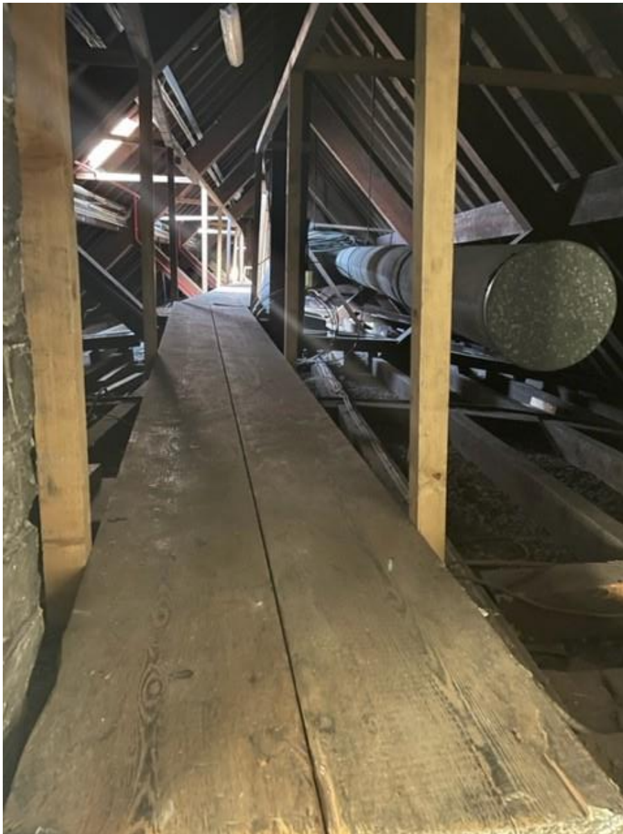
Photo 2. Roof void above Grand Hall. Boarding out required to the ceiling joists on both sides of the second roof truss to allow safe access.
