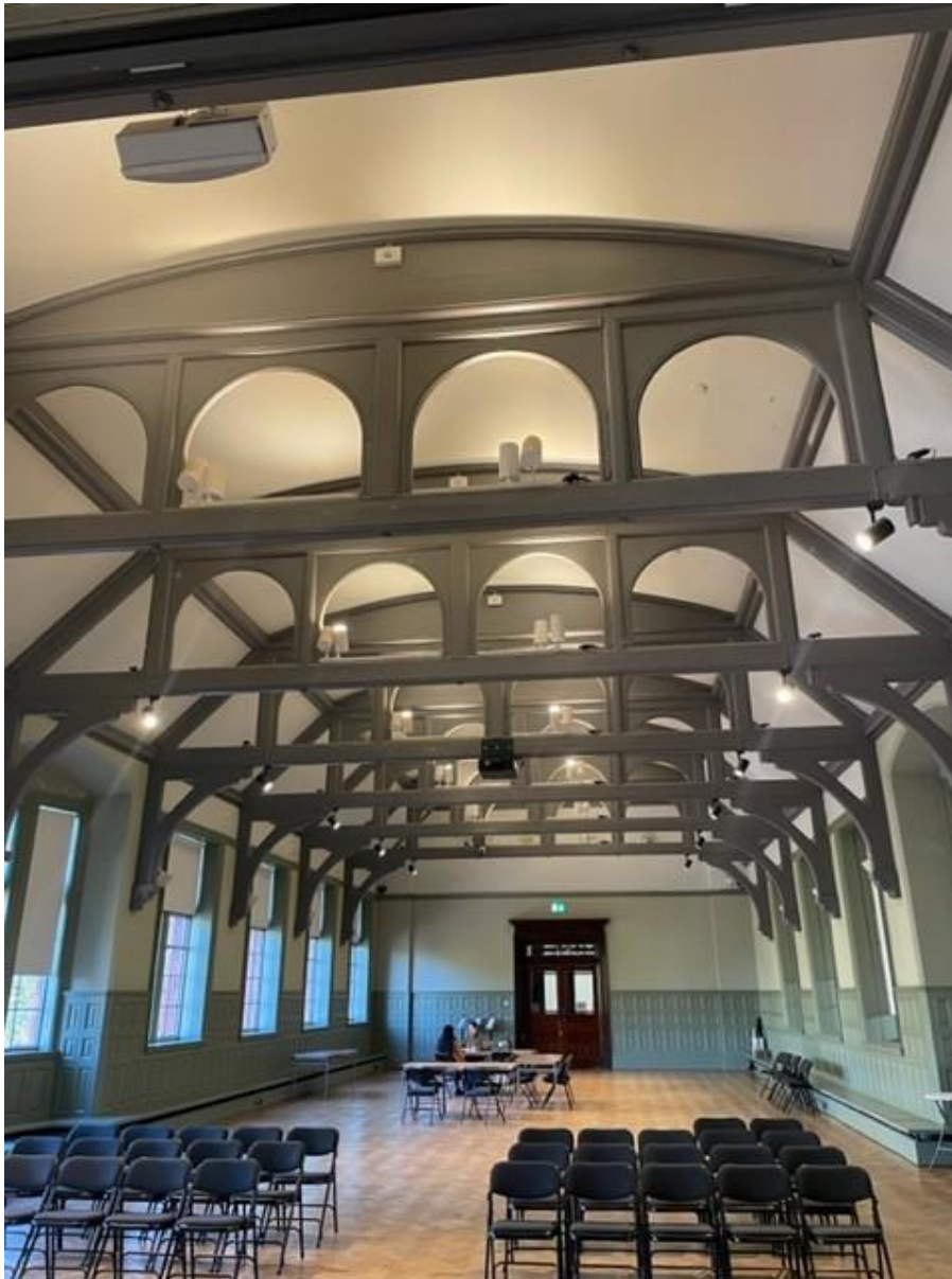
Photo 1. Grand Hall. Holes to be drilled after second truss from the south side of the room.
