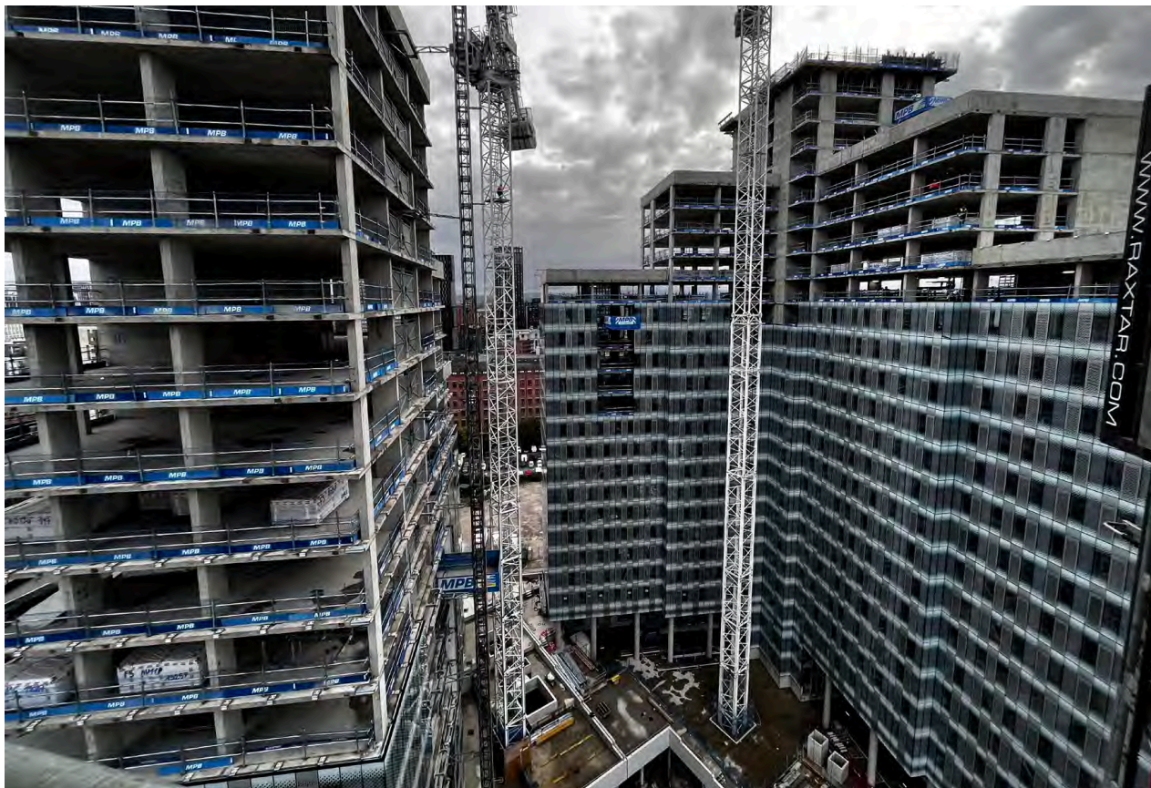
View of internal courtyard and Blocks A/B looking from Block D (Autumn 2023)
