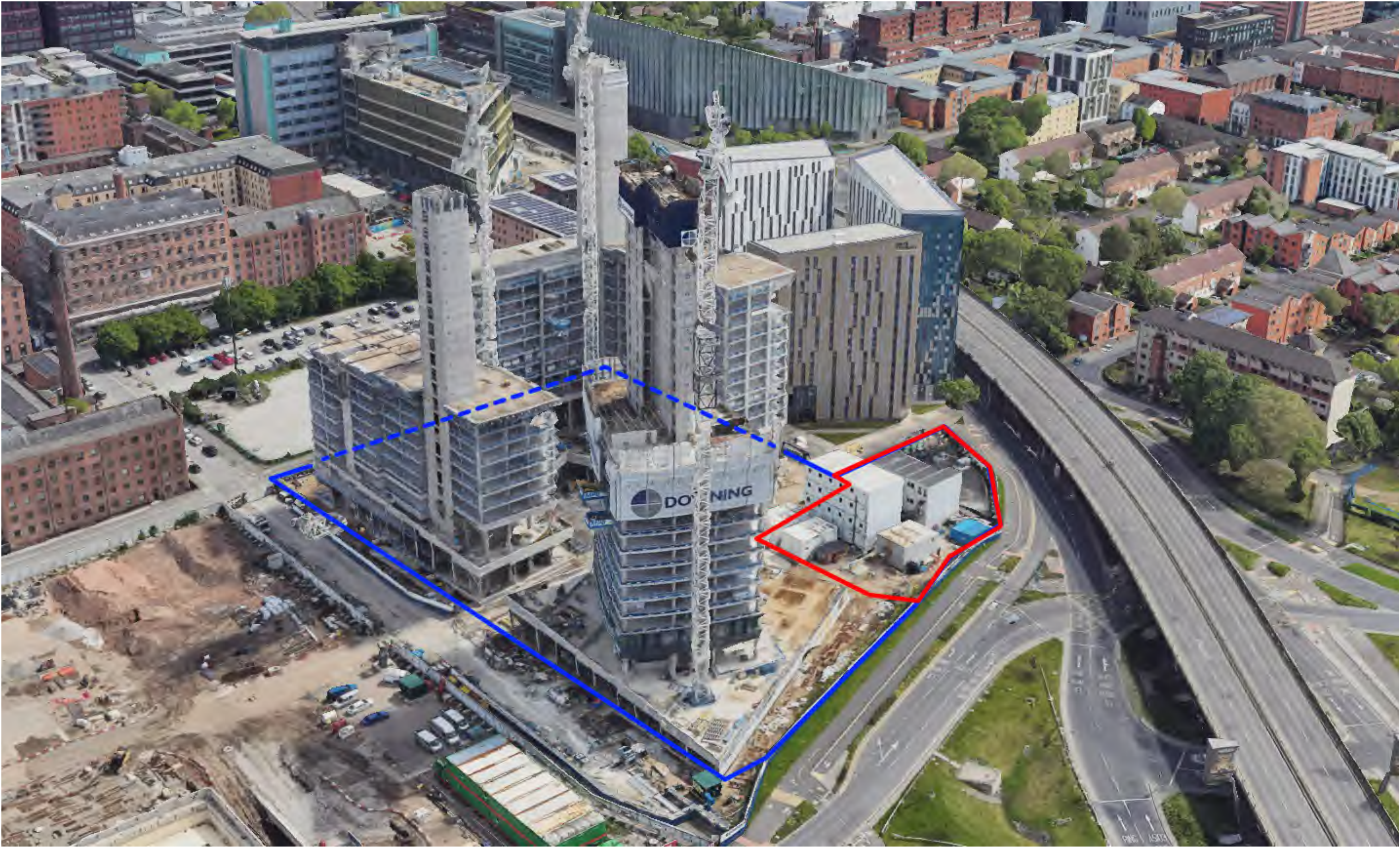
Aerial View from North West (Autumn 2023)
