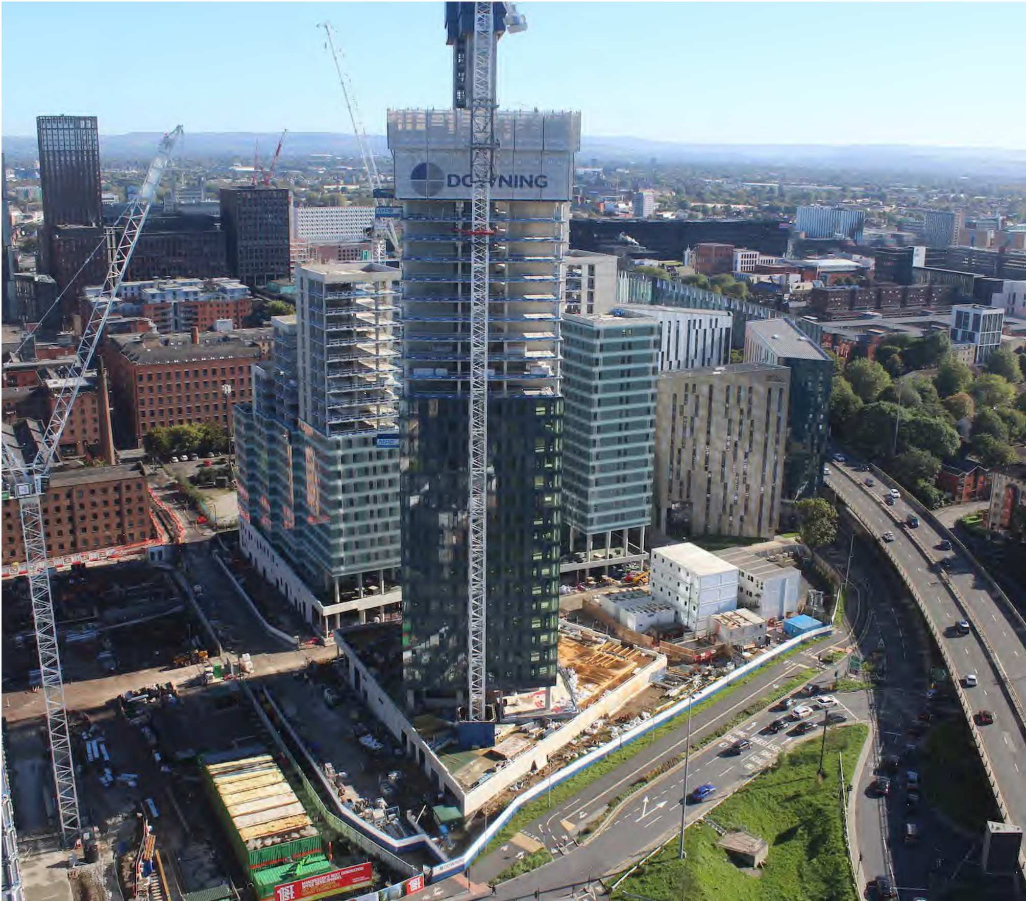
Aerial Photo from Autumn 2023 showing progress on Blocks A/B/D of the consented scheme. The plot for block C can be seen to the right , occupied by site cabins at present.
