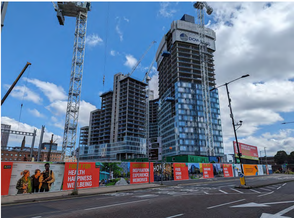
View from North West looking at consented scheme under construction (Aug 2023)
