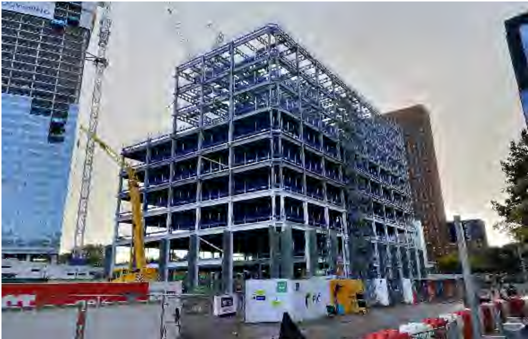
Plot 9 Under Construction [As of Autumn 2023]
