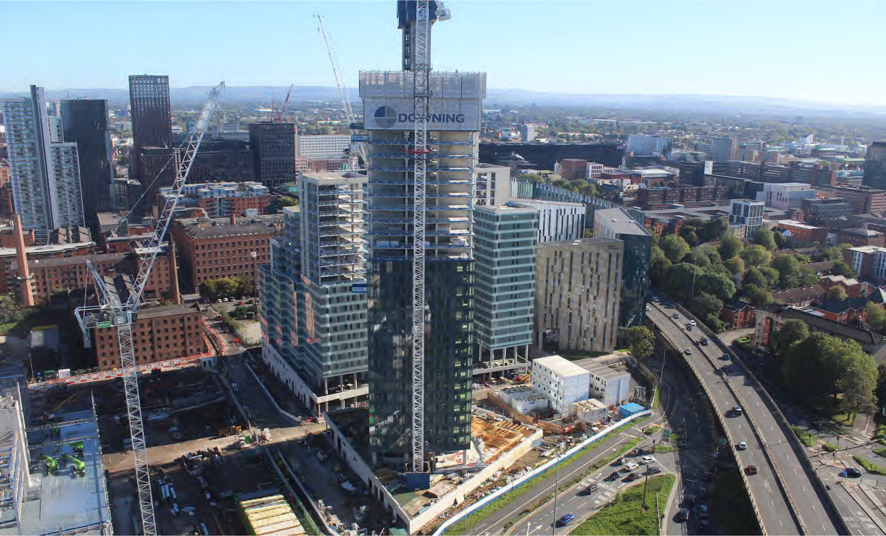
Aerial View from North West (Autumn 2023)
