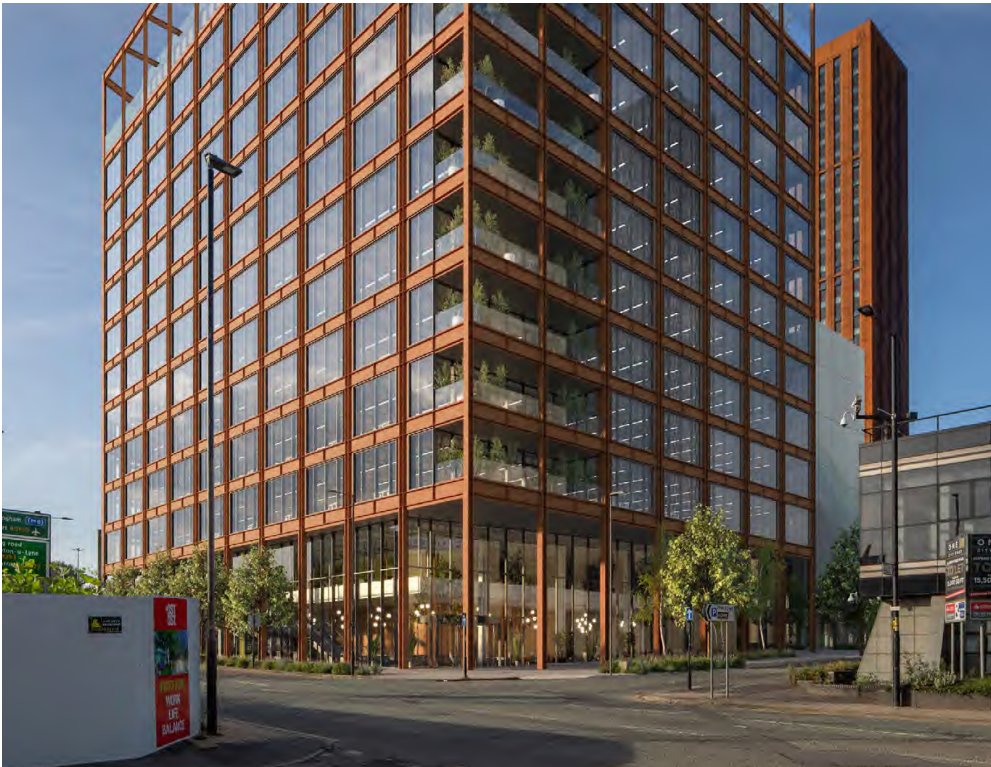
View of One Medlock Street looking South West
