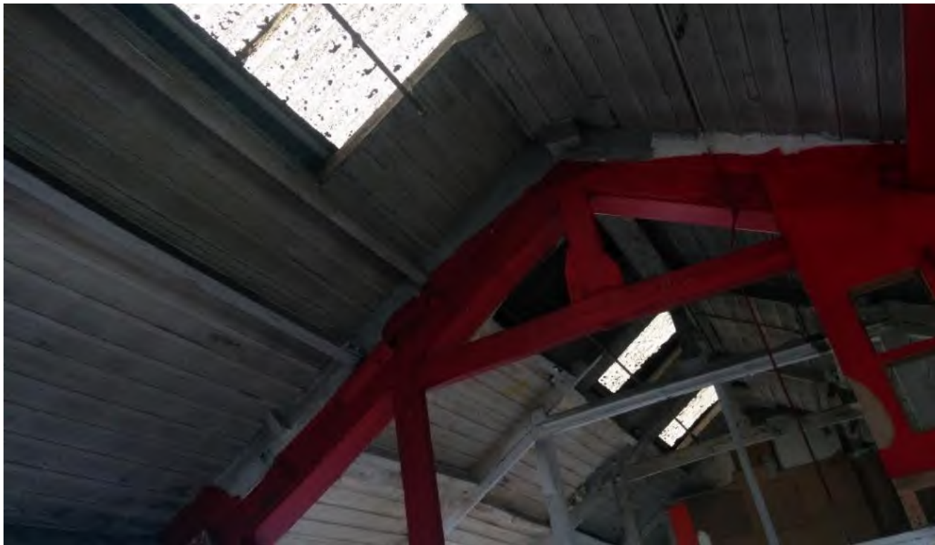
Figure 39 - Roof skylights and timber roof trusses (taken 2018)
