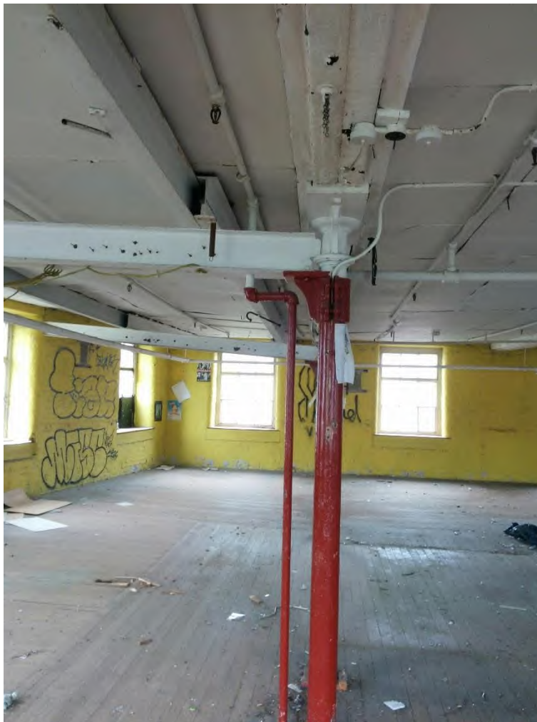
Figure 15 - New steel beams (taken 2018)
