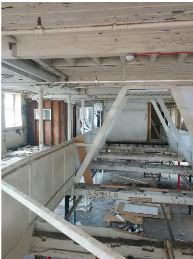
Figure 48 - Mezzanine along central part (taken 2018)
