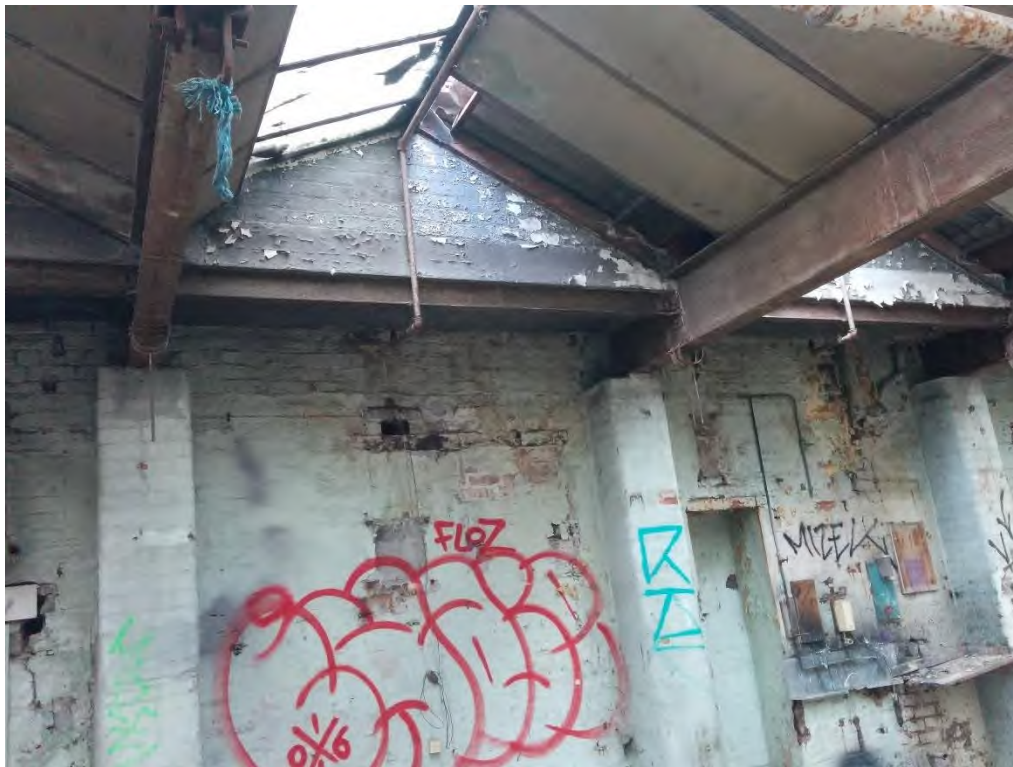
Figure 76 - Brickwork piers offering support to steelwork beams (taken 2018)
