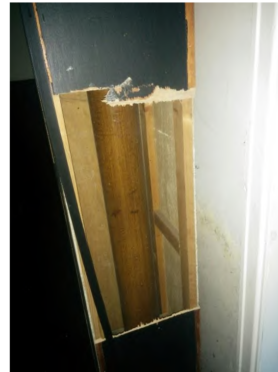
Figure 57 - Previous opening up works around cast iron columns at Upper Ground Floor Level (taken 2018)
