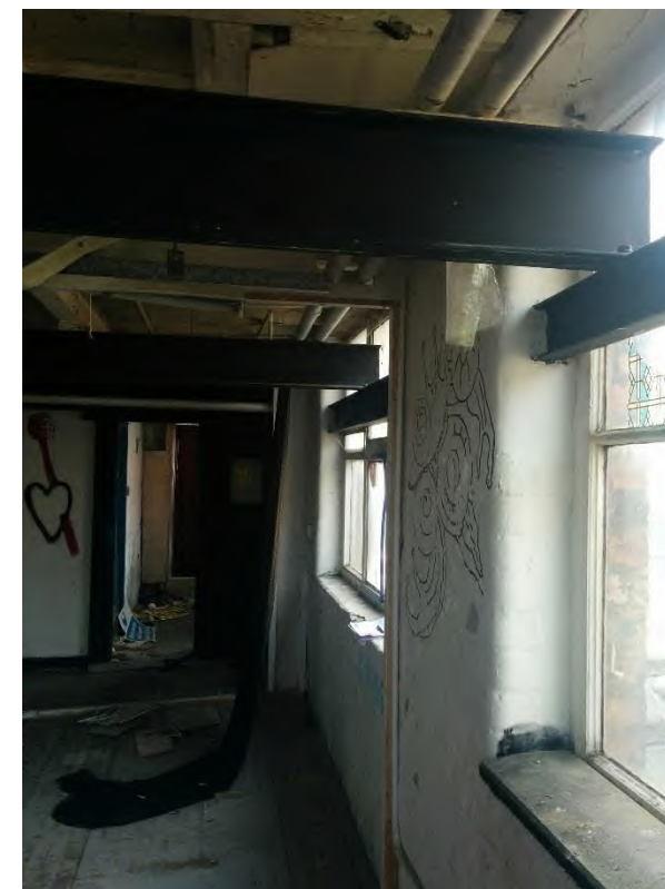
Figure 53 - Steel lintels at windows in first floor level (taken 2018)
