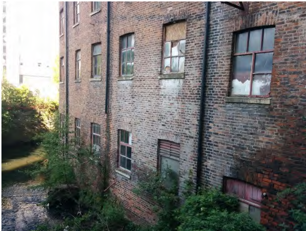
Figure 77 - Heavy vegetation growth on south elevation (taken 2018)
