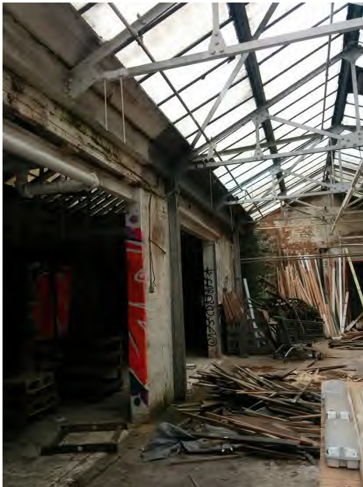
Figure 71 - Galvanised steel roof trusses and masonry piers (taken 2018)
