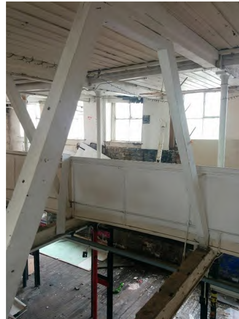
Figure 44 - Simple timber truss arrangement at mezzanine level supporting underside of third floor (taken 2018)
