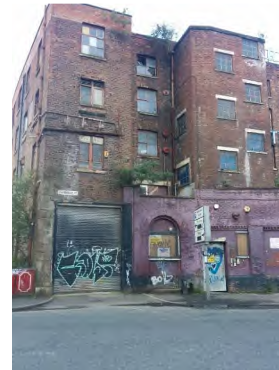
Figure 84 - Stone lintels above staircase windows (taken 2018)
