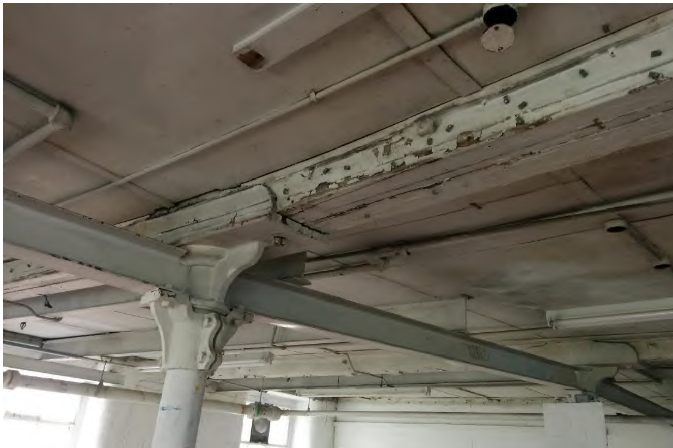
Figure 25 - Primary steel beams bearing onto cast iron columns (taken 2018)
