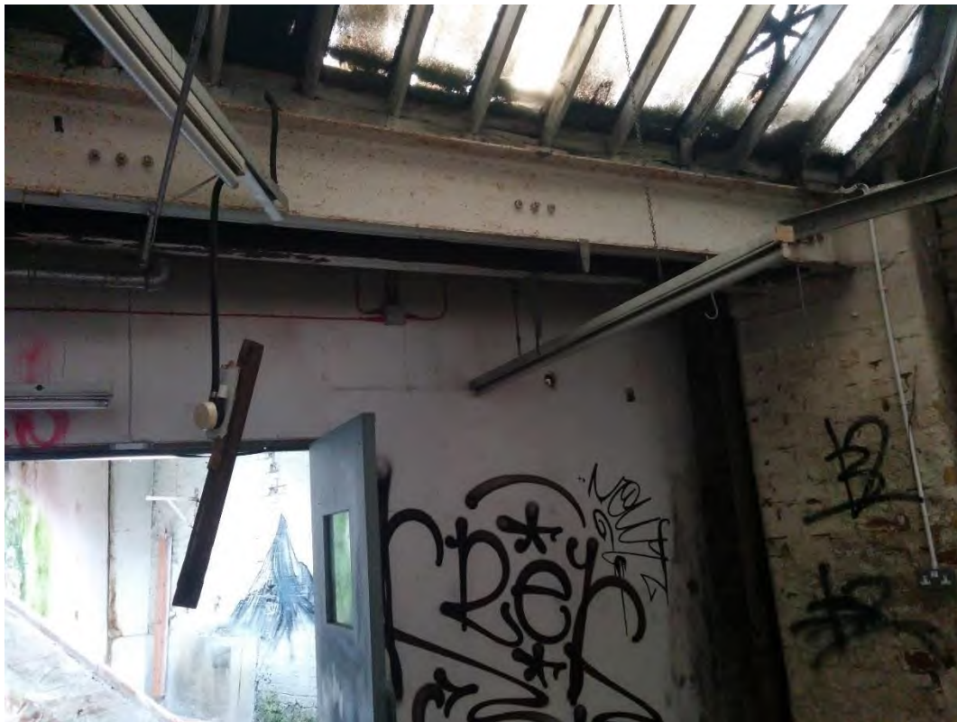
Figure 73 - Timber beam strengthened with two PFC steel sections (taken 2018)
