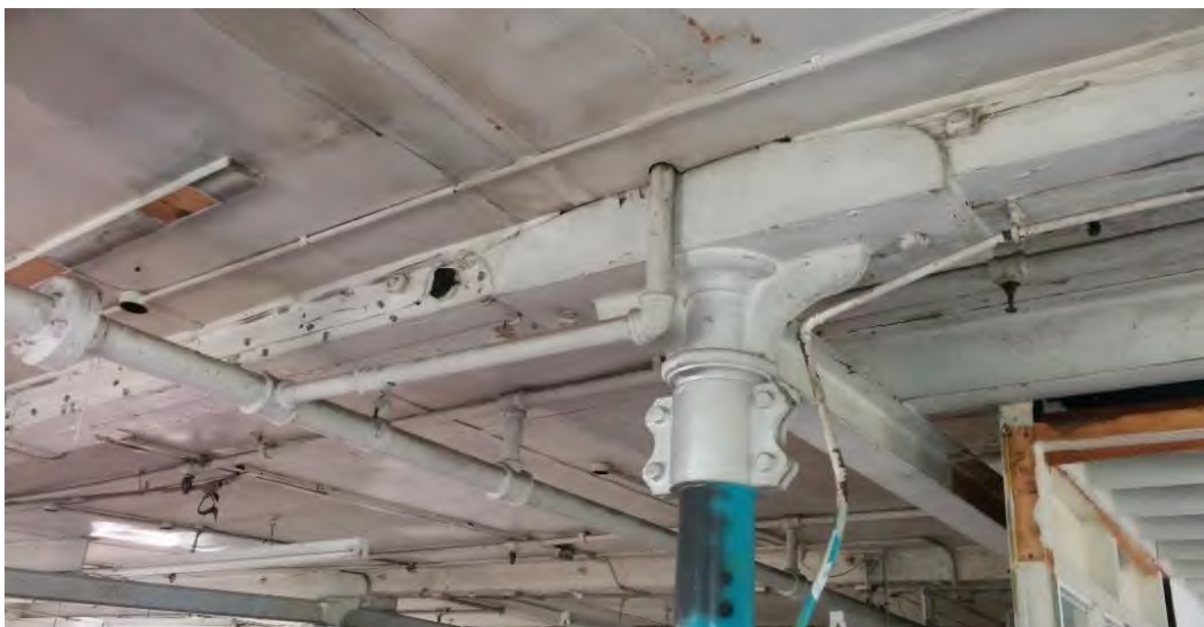
Figure 26 - Secondary steel beams bearing onto primary steel beams (taken 2018)
