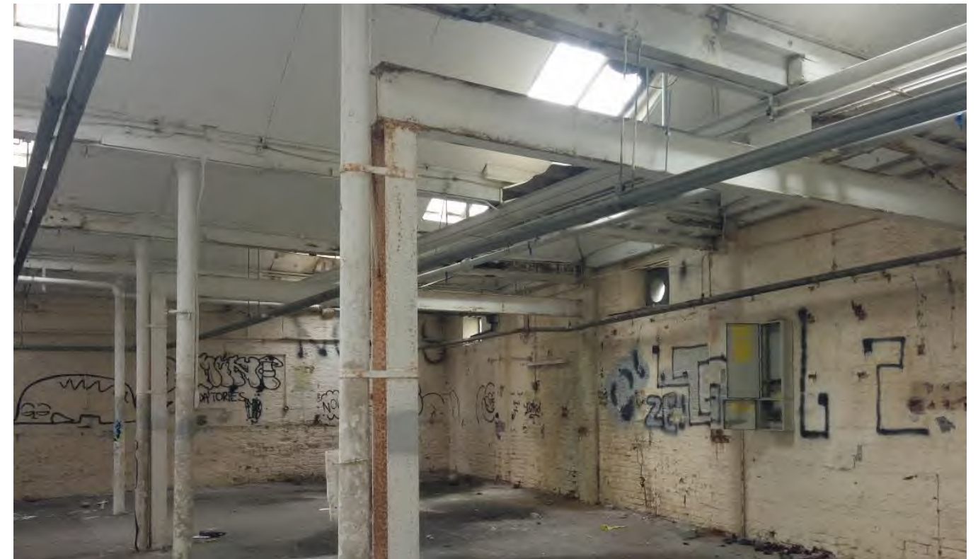
Figure 65 - Portal frames at every other bay offering support to timber roof (taken 2018)
