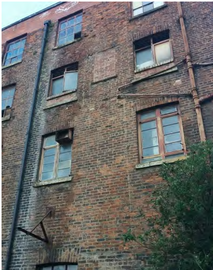
Figure 79 - Modern brickwork infill at second floor (taken 2018)
