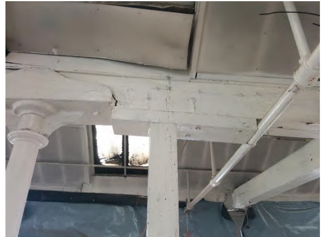
Figure 16 - Timber board introduced with the timber posts (taken 2018)
