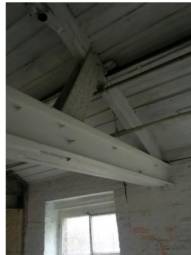
Figure 42 - Timber beam strengthening with PFC sections and steel plates (taken 2018)
