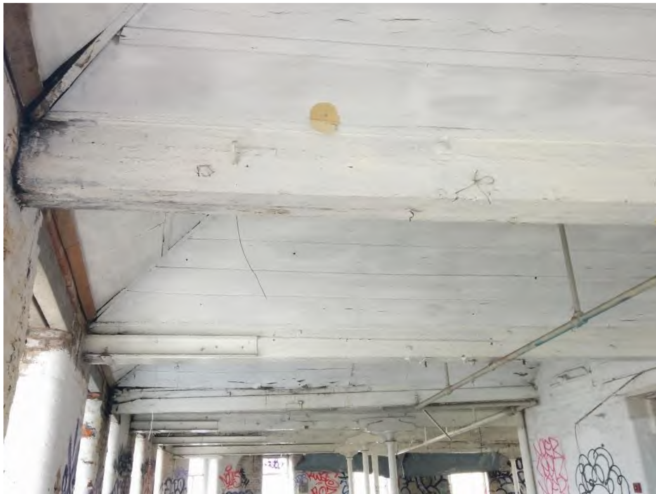
Figure 11 - False ceiling at roof level (taken 2018)
