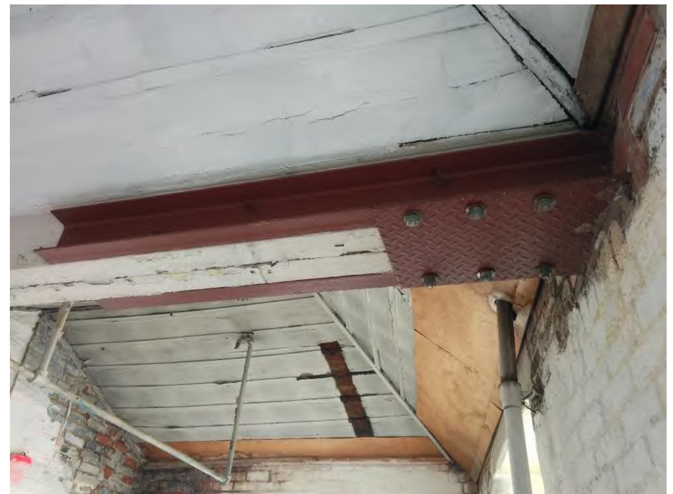
Figure 12 - Previous strengthening of timber beams (taken 2018)
