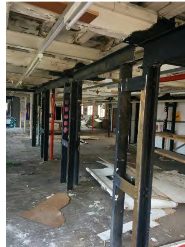
Figure 52 - Supplementary steelwork structure at first floor (taken 2018)
