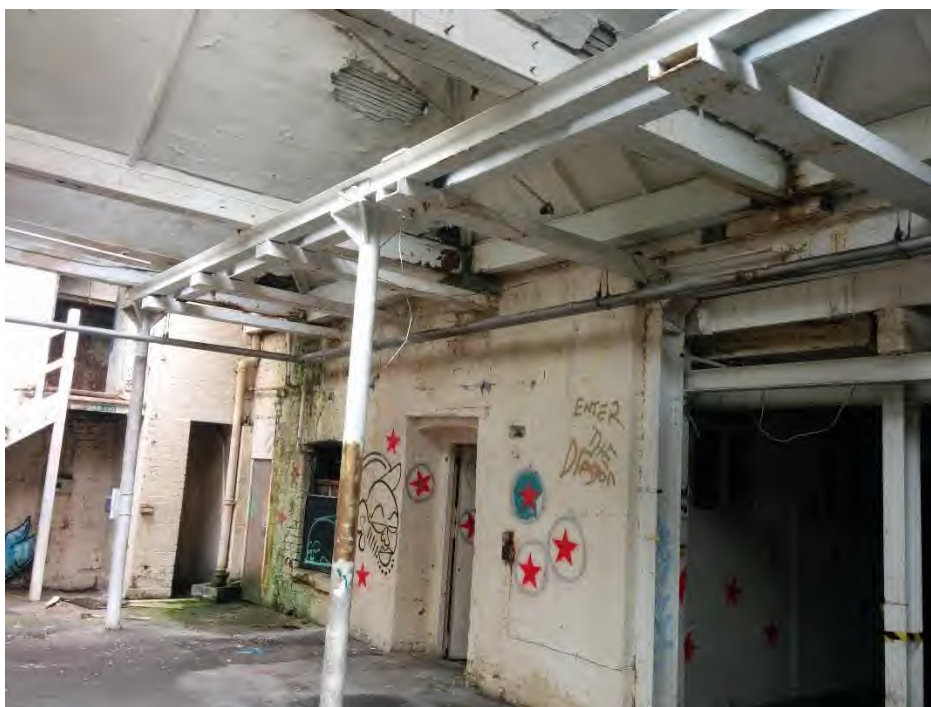
Figure 64 - Additional steelwork PFC sections (taken 2018)
