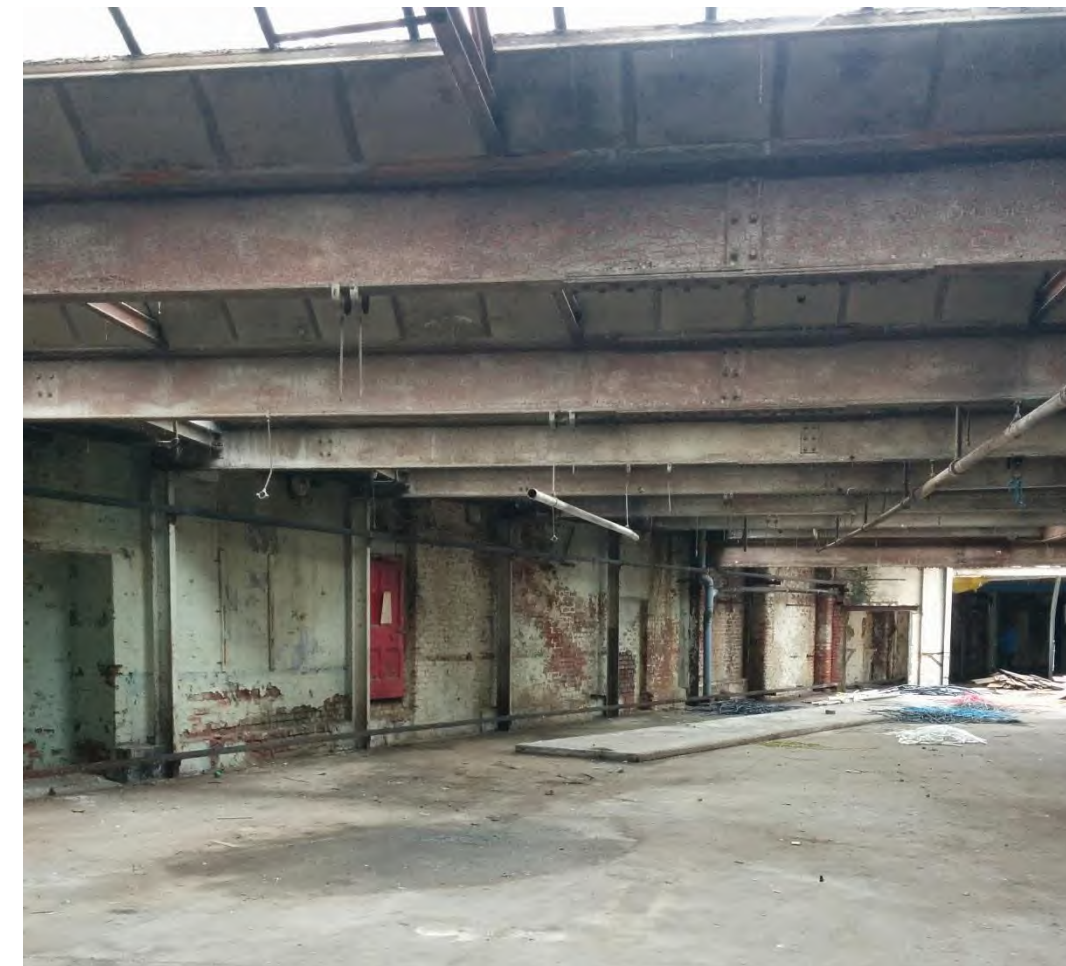
Figure 75 - Western section of the shed (taken 2018)
