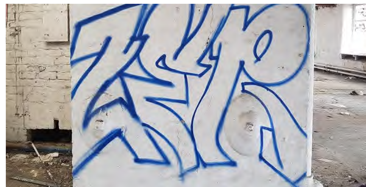
Figure 18 - Brickwork pier adjacent to the lift shaft (taken 2018)
