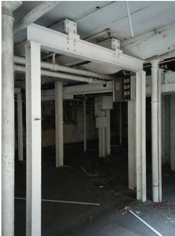
Figure 60 – Steelwork frame in basement (taken 2018)
