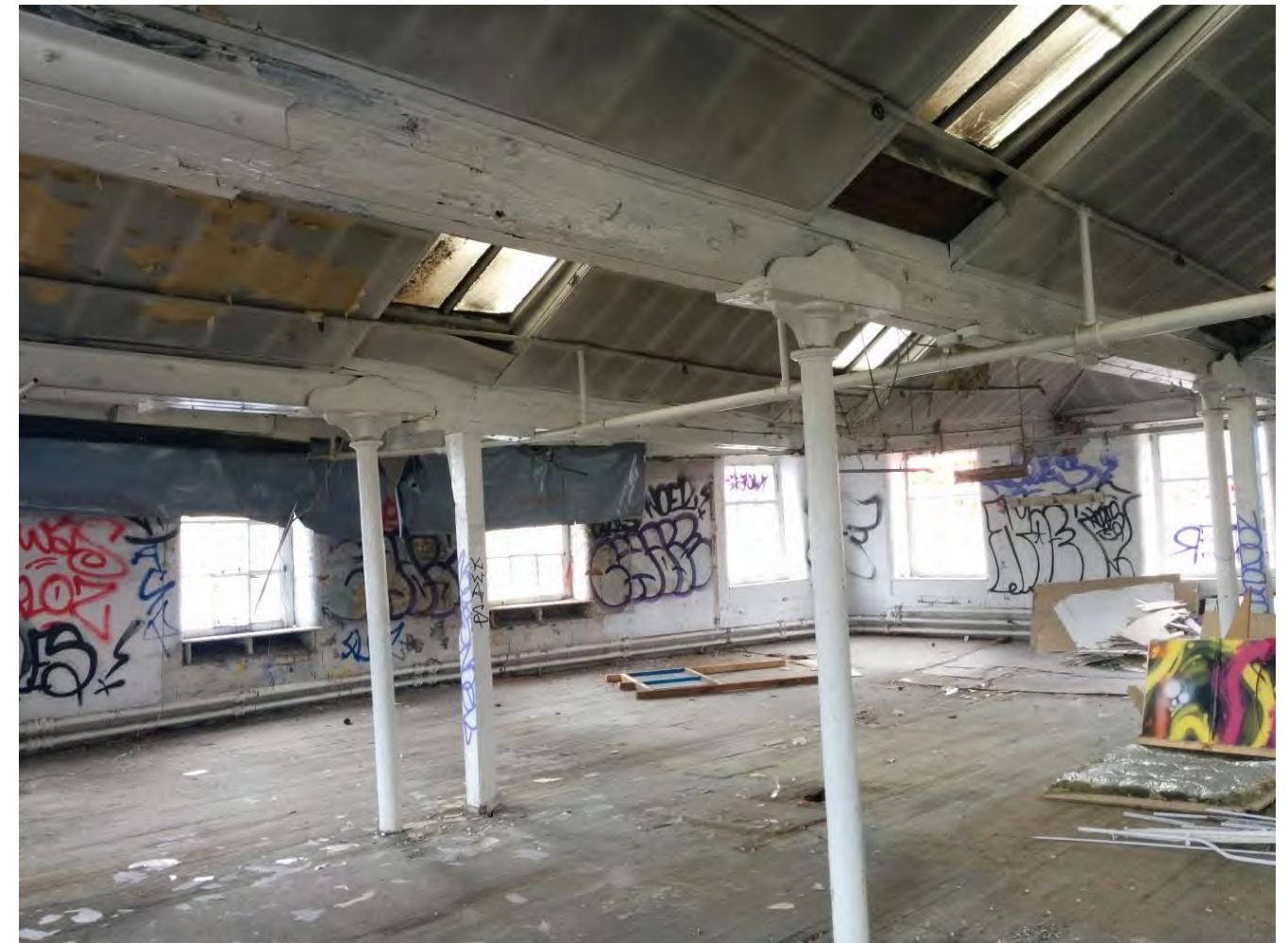
Figure 10 - Warehouse Roof Structure (taken 2018)
