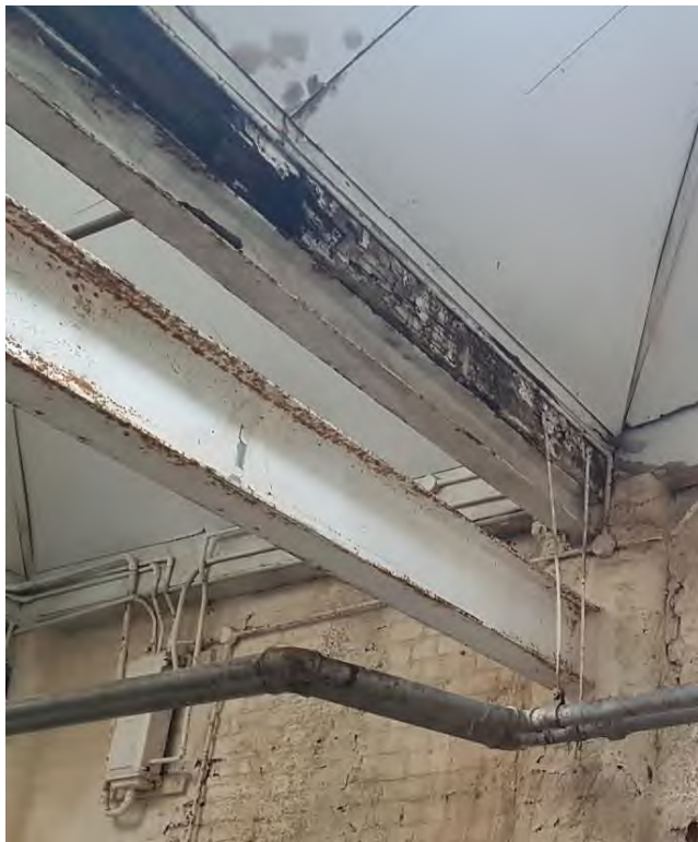
Figure 62 - Additional steel beams supporting timber beam (taken 2018)
