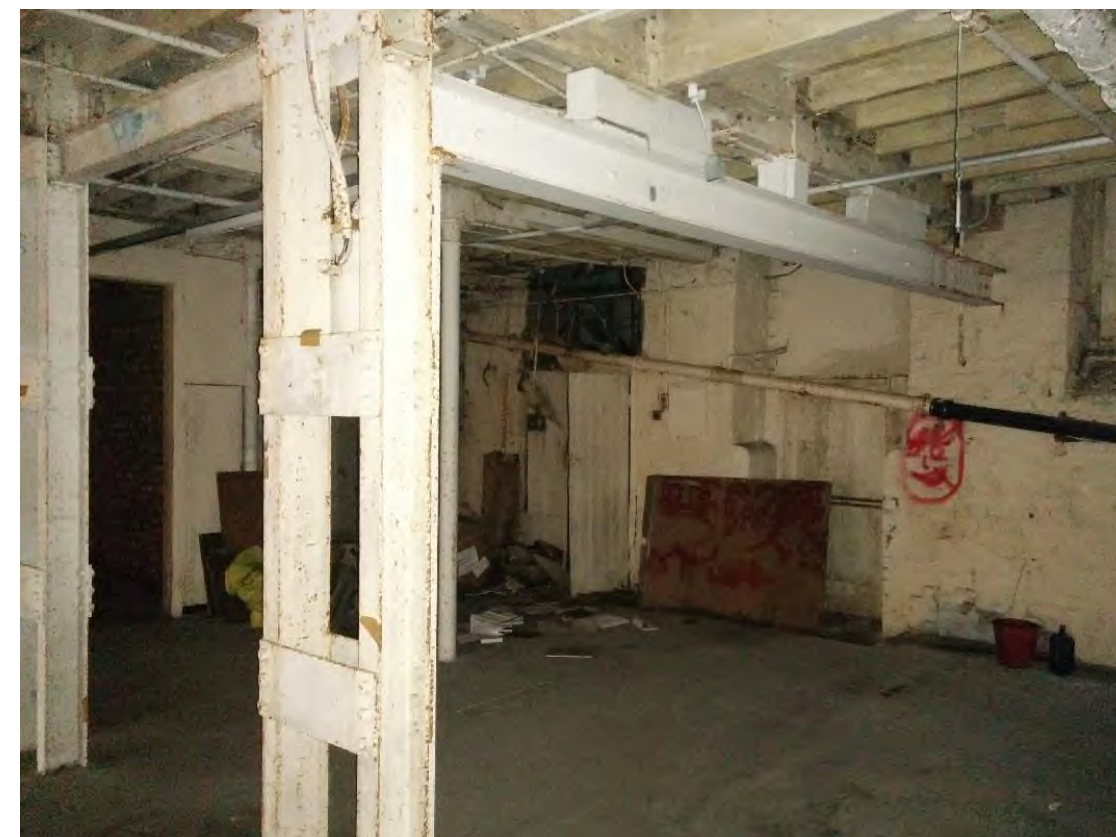
Figure 59 - Supplementary steelwork in basement (taken 2018)
