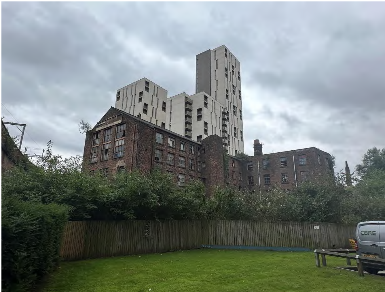
Figure 81 - Western elevation (adjacent to River Medlock) showing continued vegetation growth (taken 2023)
