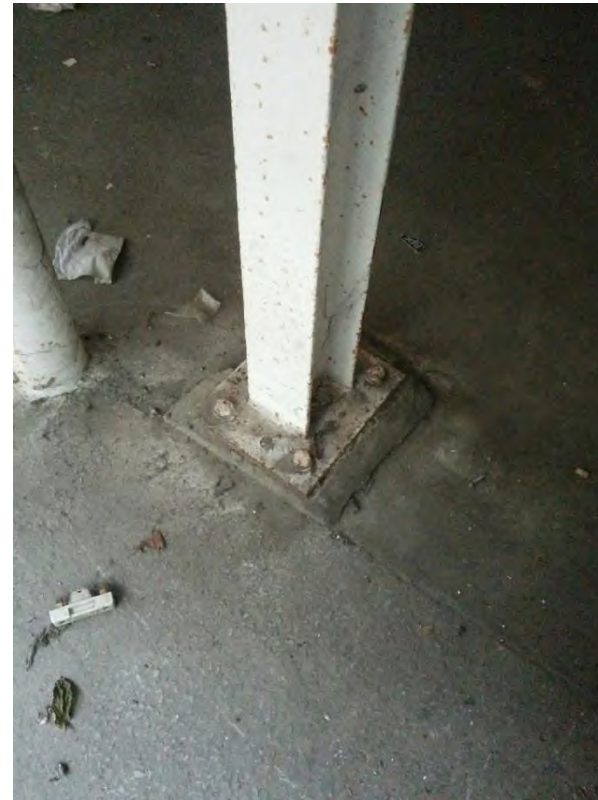
Figure 61 - Column baseplate detail (taken 2018)
