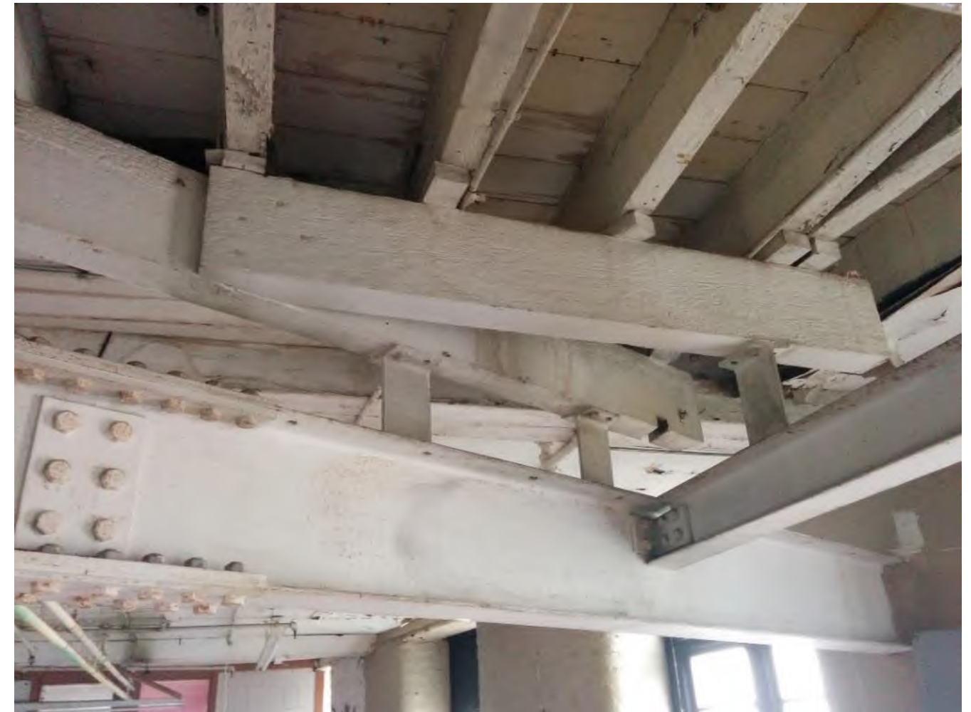
Figure 27 - Complex steel and timber beam structure (taken 2018)
