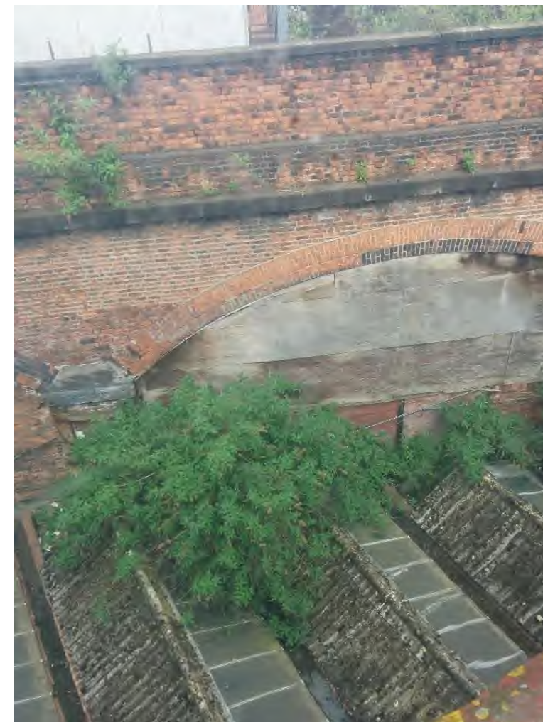
Figure 70 - External roof structure of the shed (taken 2018)
