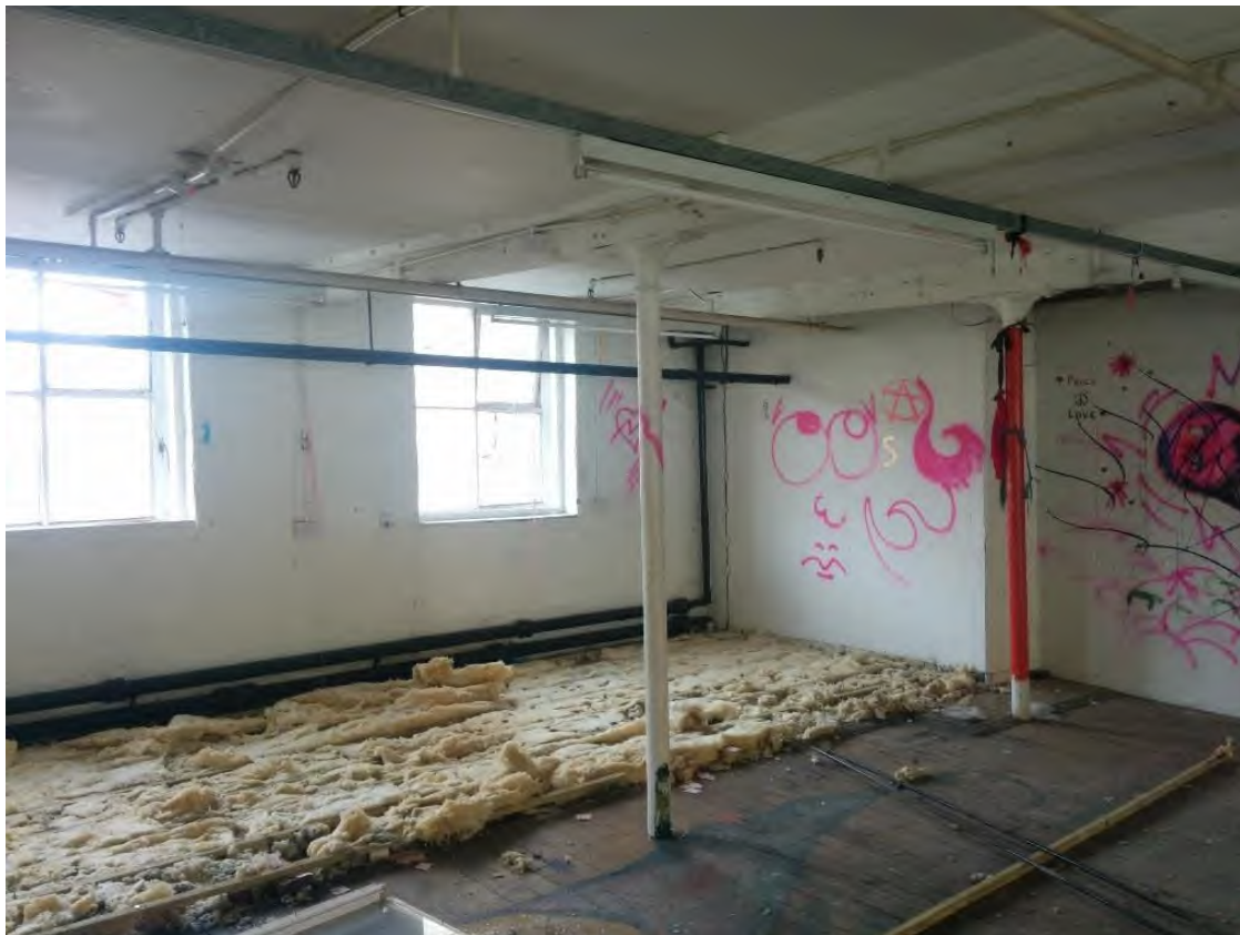
Figure 51 - Fibre materials overlaying timber floor at first floor level (taken 2018)
