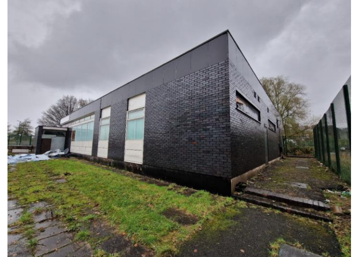
Right: View of existing bank building showing existing brickwork, glazing, high-level fascia and perimeter security
