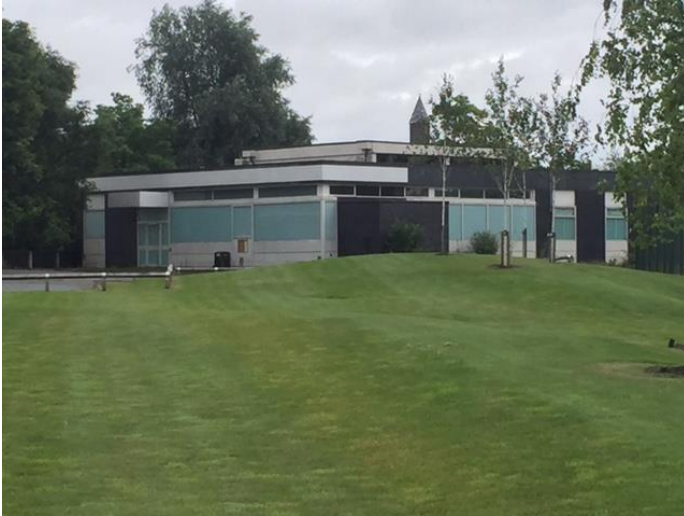
Left: View of existing bank building showing existing brickwork, glazing, flat roof and clerestory window
