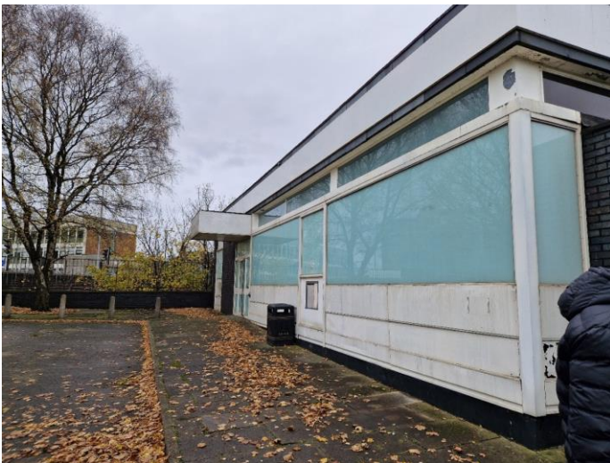
Left: View of existing bank building showing existing entrance, glazing and high-level fascia
