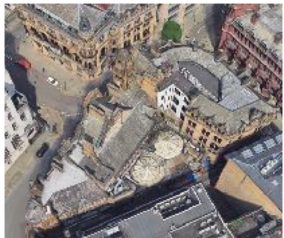
Fig. 2 Aerial view from rear of site
