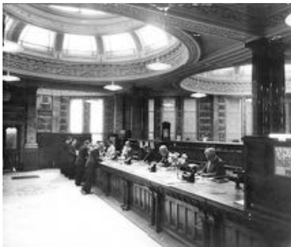
Fig. 5 Ground Floor Banking Hall 1969
