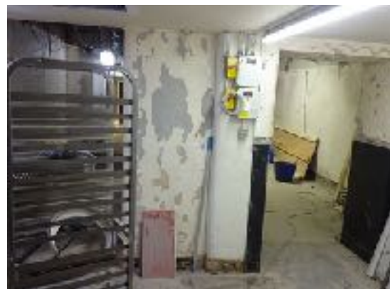
Fig. 11 Former Walk In Fridge/Freezer
