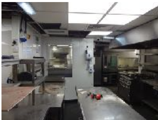
Fig. 10 Kitchen Area Photograph
