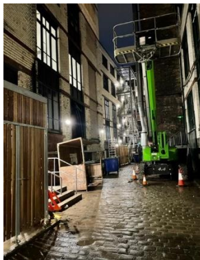
View of lighting beyond archway prior to neighbouring security light triggered
