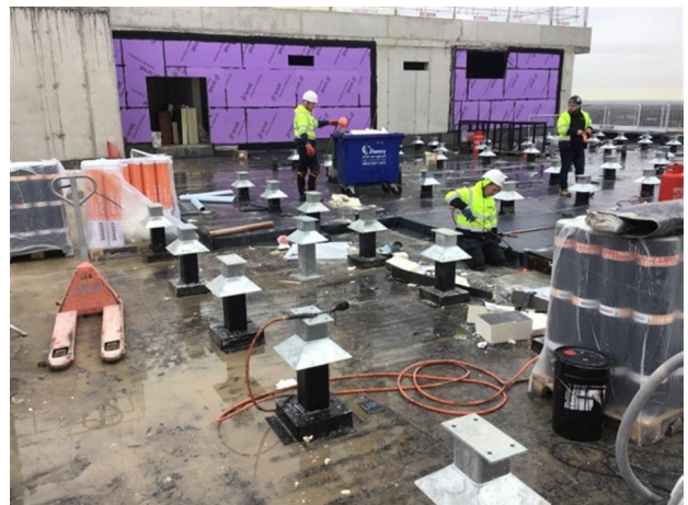
Photo 8 - Overview of level 9 section 1
