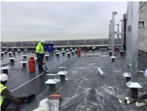
Photo 5 - View of progress to date
