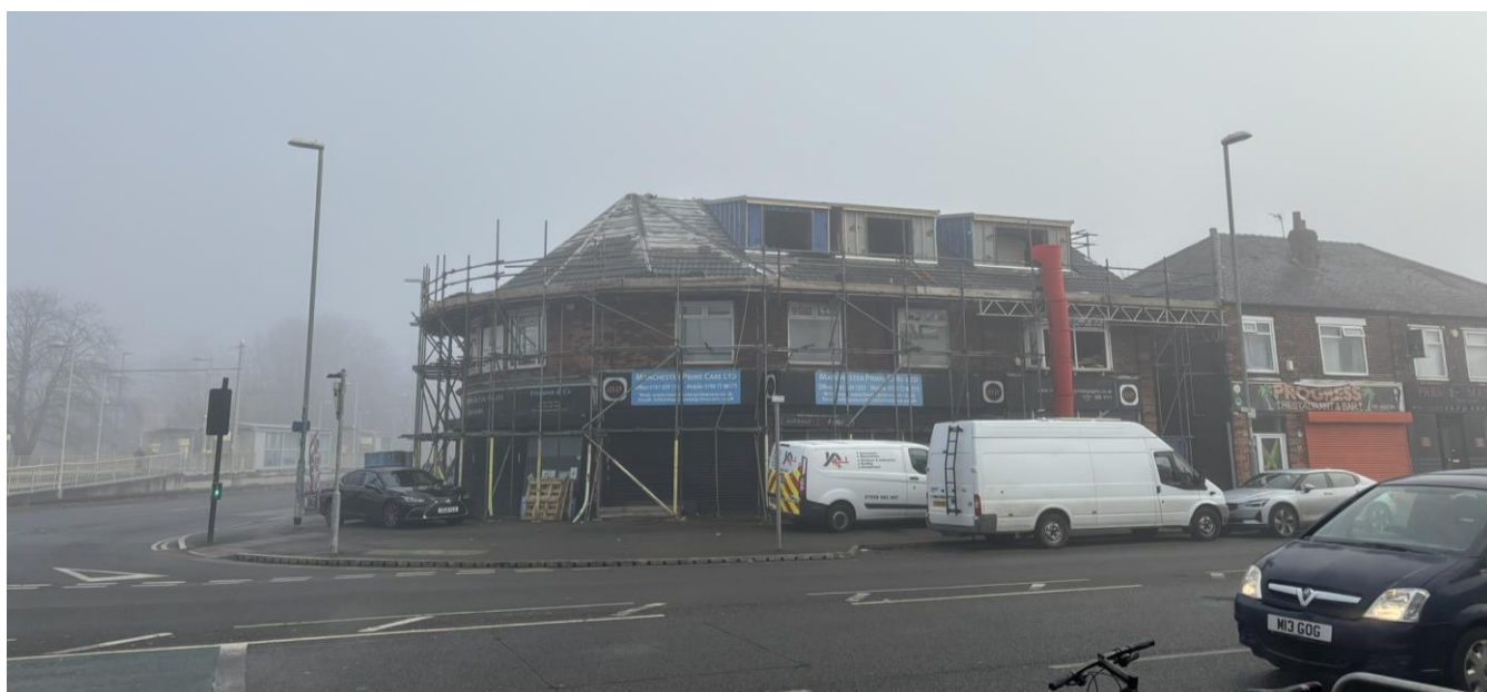
Figure 1. View of application site.
