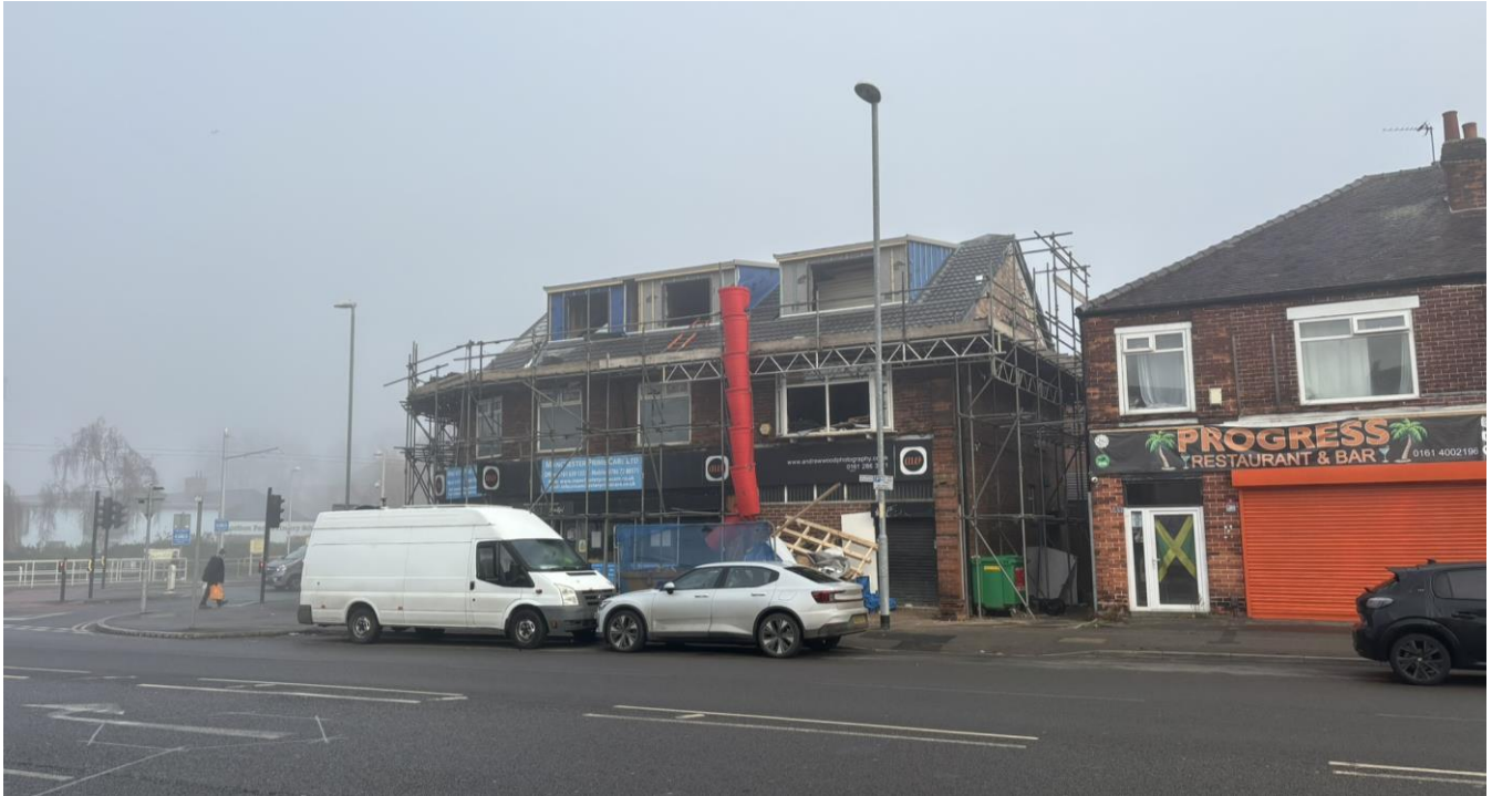
Figure 2. View of application site.
