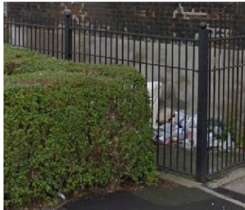
Image of existing metal railing
